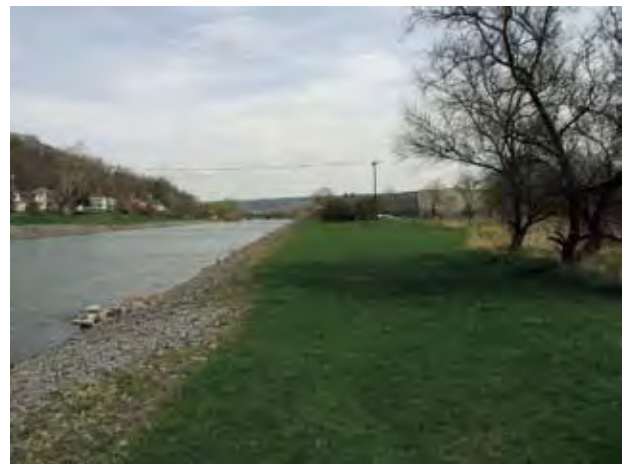
Cayuga Inlet Flood Control Channel through the west side of the City of Ithaca
