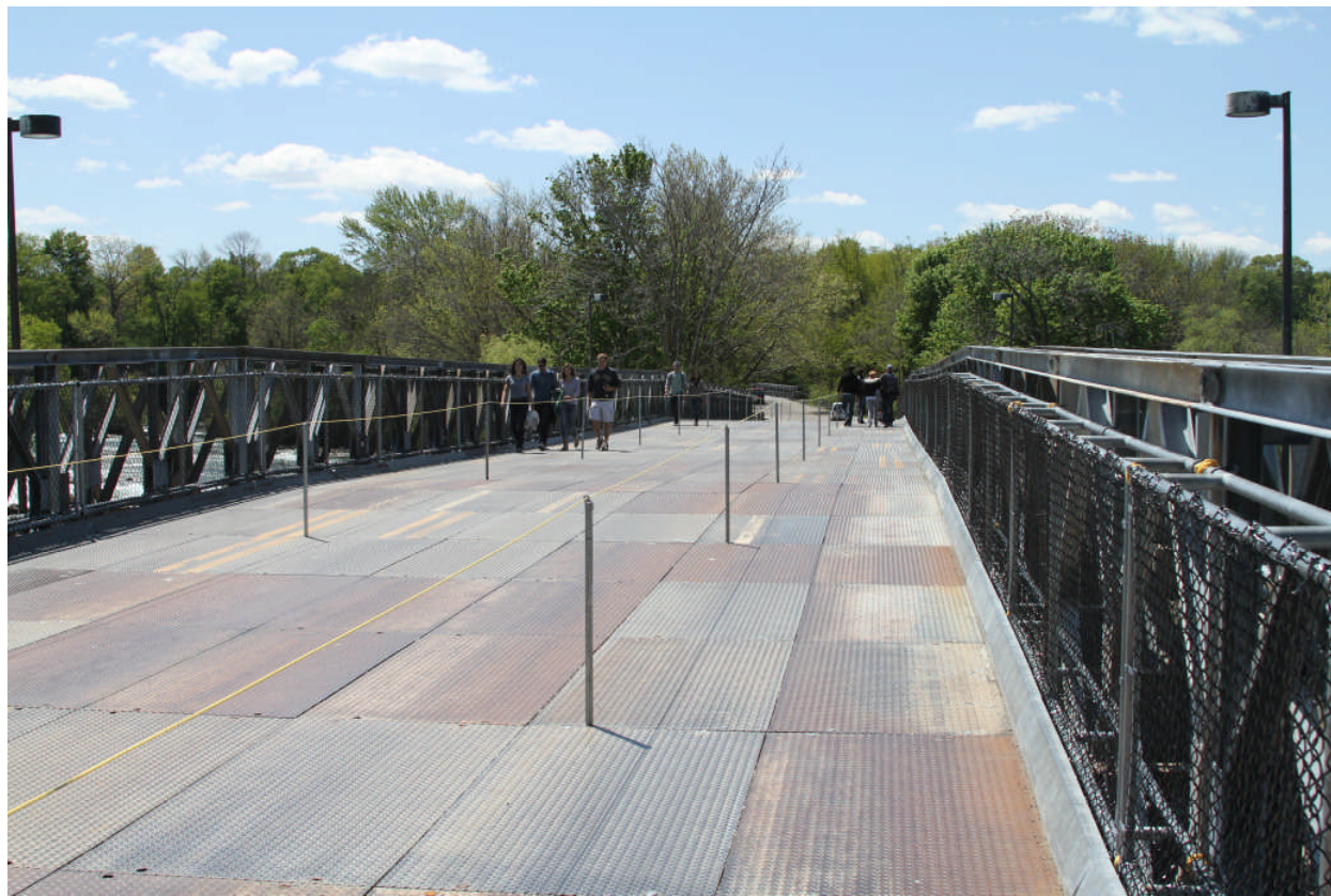
Figure 1.2.1.2.c Temporary Mabey Truss Bridge
