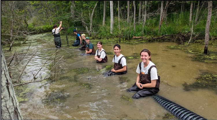
FORCES Stewards, SCA, and EFT Staff installing a 'Beaver Baffle' to level out ponds at Mark Twain State Park. Photo: OPRHP
