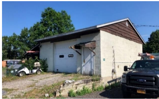
The Regional Maintenance Facility at Baird, which serves OPRHP's Taconic Region
