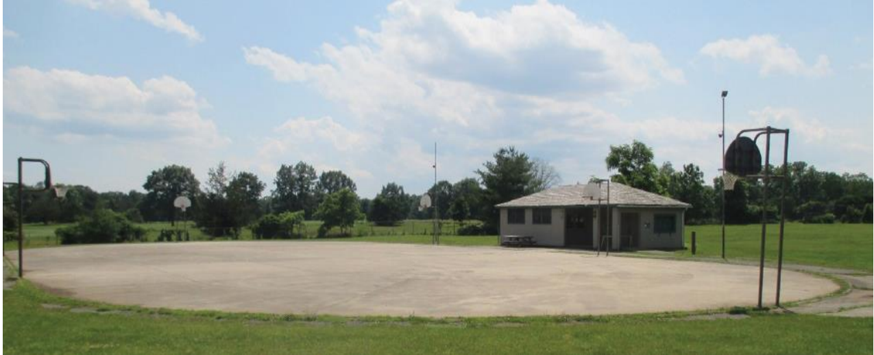
A former roller rink pad at Baird is now used for basketball. The small building to the rear is no longer in use; original to the Park, it has been used as a ball-lending stand and a nature center.
