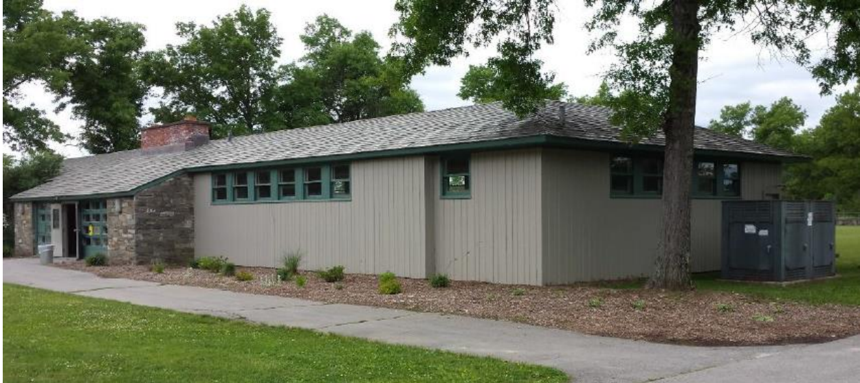
The Park's original bathhouse will be retrofitted as an event facility
