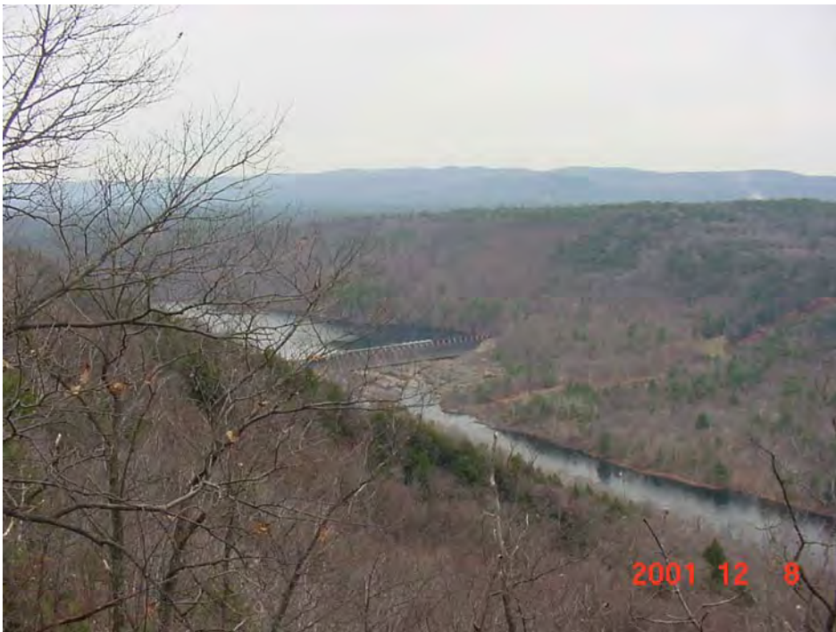
Western Ridge Trail, central, spur 2 dam
