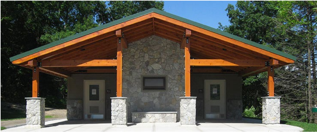
A Lot Restroom
