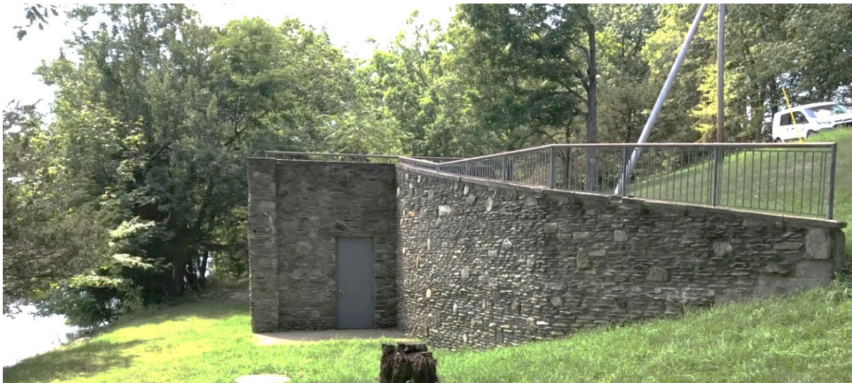
The Park's water treatment facility uses water from the lake to provide potable water.
