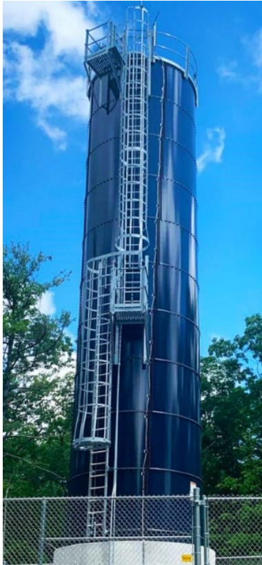
East end water tower
