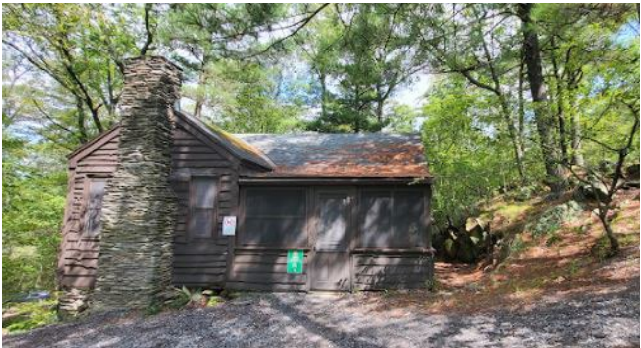
Original CCC-built cabins are still in active use at the Park’s campground.
