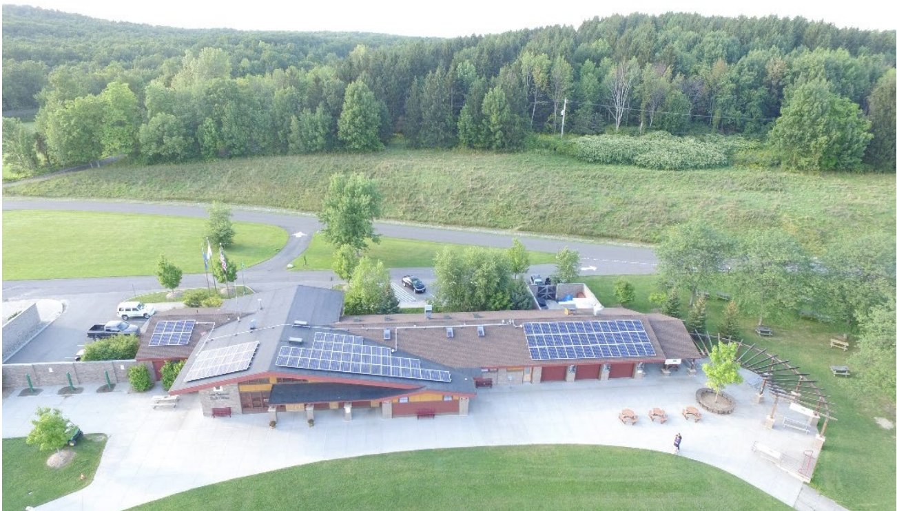
PV system on the West Bathhouse roof.
