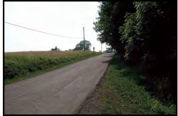
SP 41+300 W: View west at intersection of the trail crossing of Glenwood Heights Road. Site distance is adequate in the upslope direction from both north and south trail approaches.
