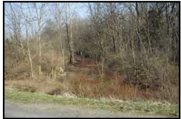
SP 66+300: View south from Gorge Road to trail corridor. Gorge Road is 8 feet above the trail elevation. Ramps will need to be constructed in this area.
