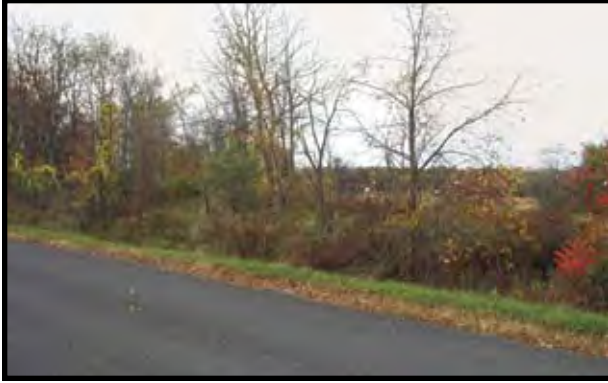
SP 50+200: View of trail corridor north from Houghton Road intersection. This segment of trail is fairly overgrown and difficult to locate in the landscape.
