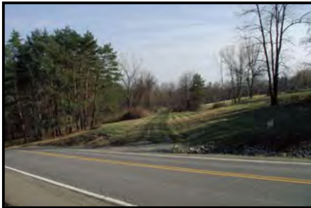
SP 43+700: View of the trail south of Perry City Road. Road crosses at a 45-degree angle and has a steep cross slope towards the east (left in photo.)
