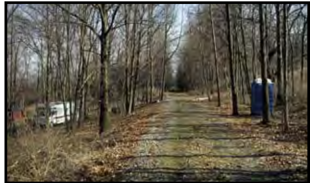
SP 42+500: A residence has been built along the east side of the corridor. A screening treatment is recommended between the trail and adjoining land use.
