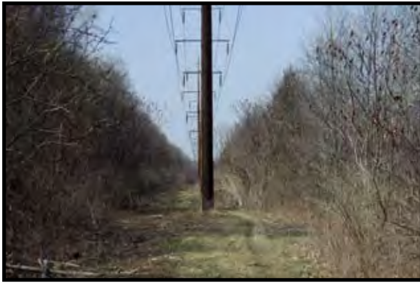
SP 24+000: Between the Cass Park Trailhead and approximately SP 32+500 the trail will co-exist in the corridor with an existing electric transmission line. The trail weave around the poles.
