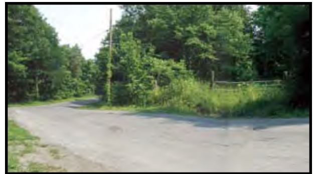
SP 41+300 E: View southeast at the intersection of the trail and Glenwood Heights Road. Site distance for trail users traveling north is limited downslope. Selected clearing of vegetation may improve the condition with the support of the warning sign program.
