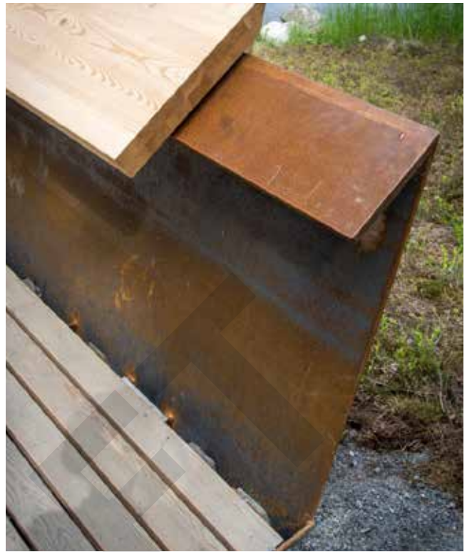
CORTEN STEEL WITH GLULAM Material for super structure and deck
