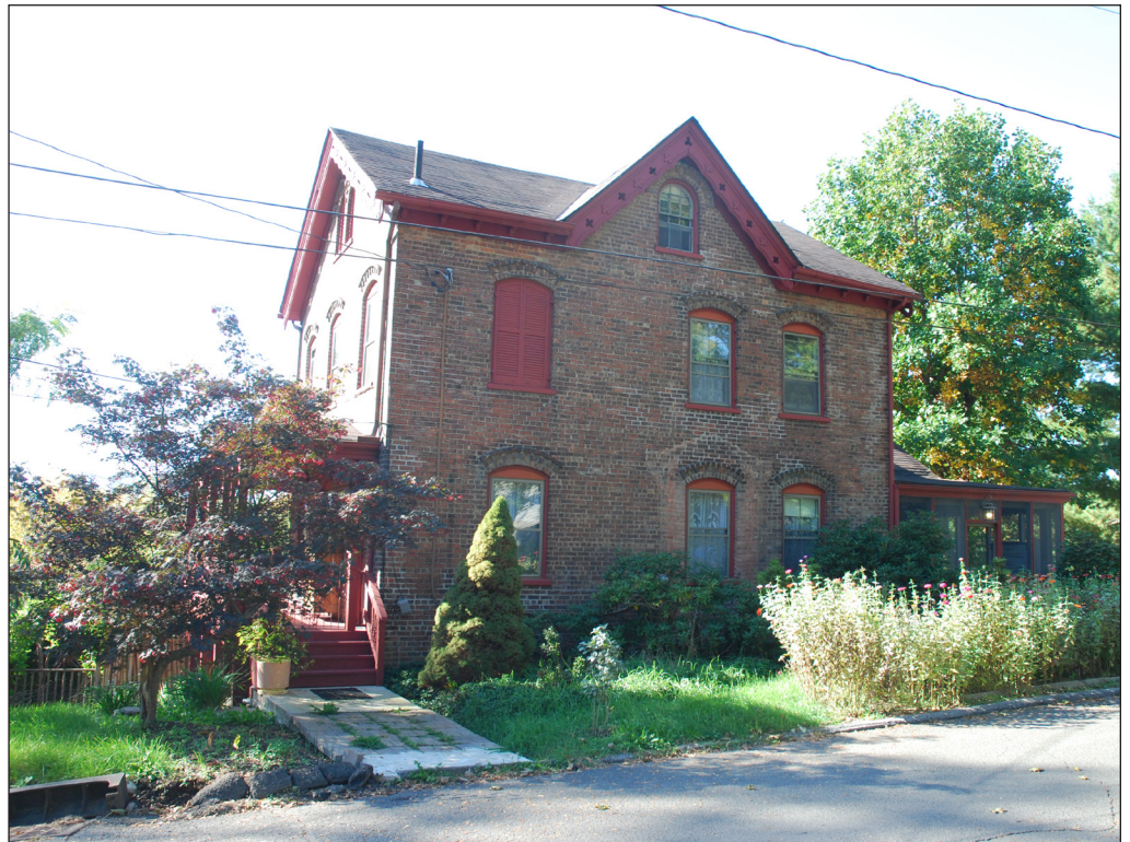
17 Newlins Mill Road, north elevation 4
