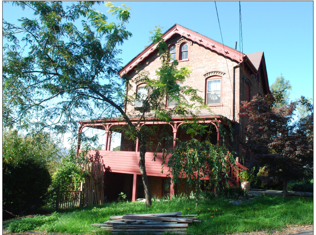
17 Newlins Mill Road, east elevation 3
