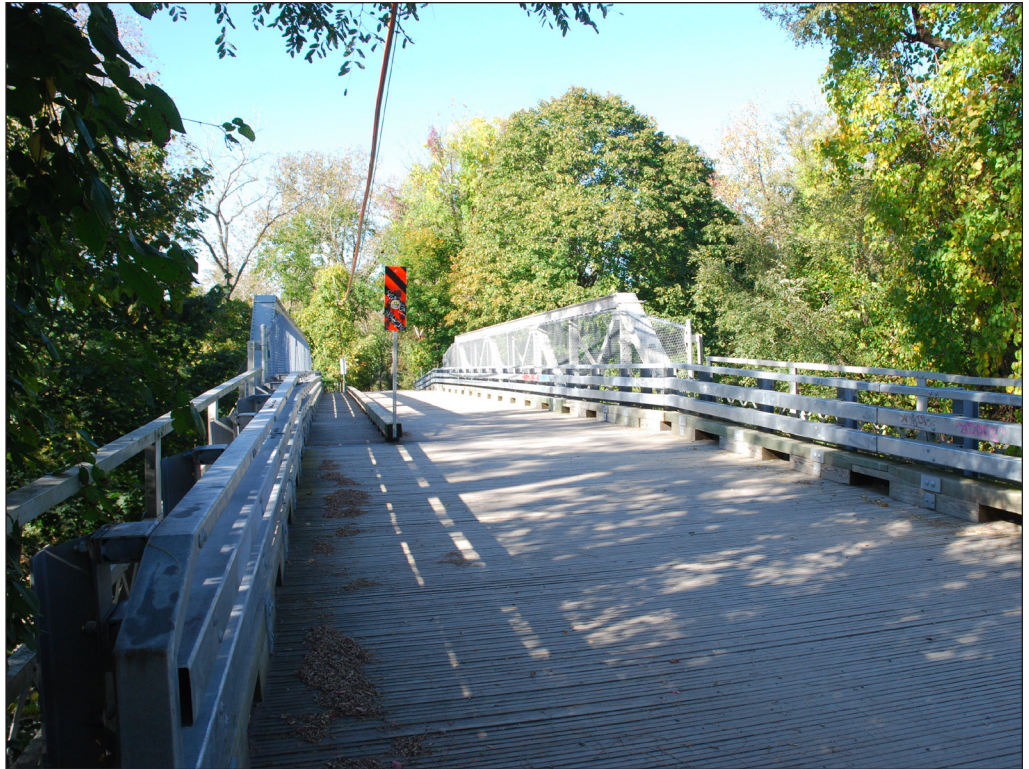
Denning's Point Road Bridge (S/NR-eligible) 1
