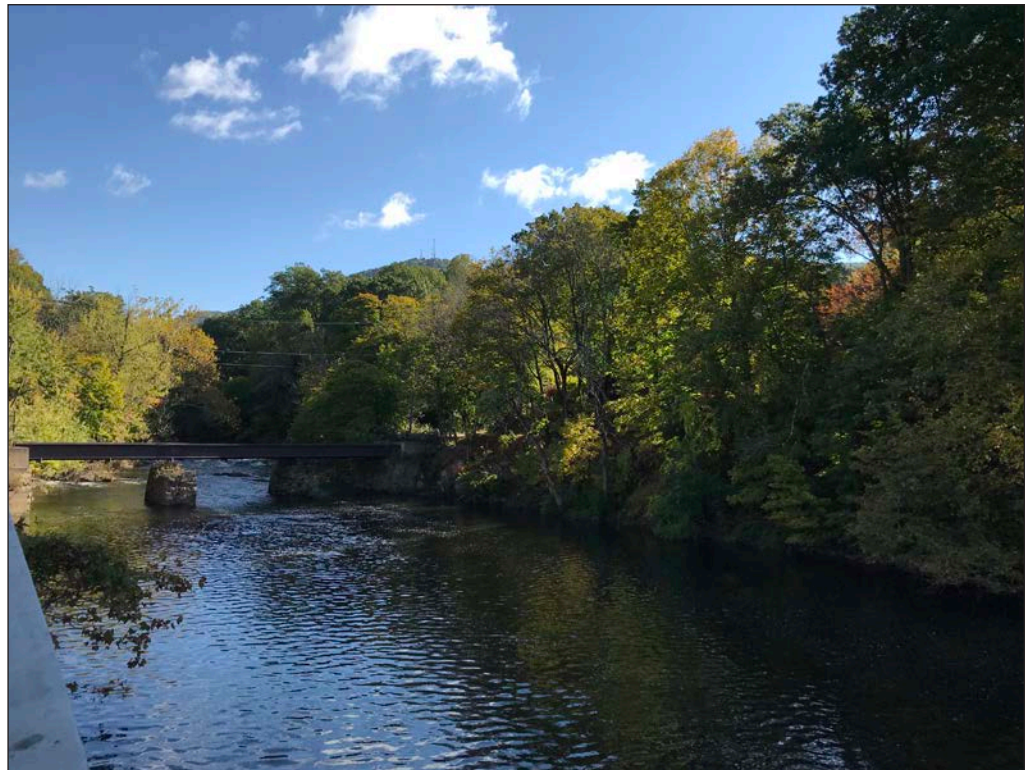
View from Madam Brett Park to Old South Ave Bridge facing east 10
