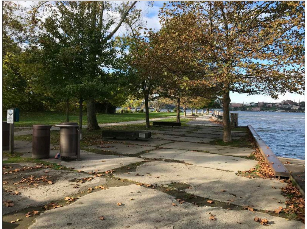
View from Long Dock Park facing southwest 5
