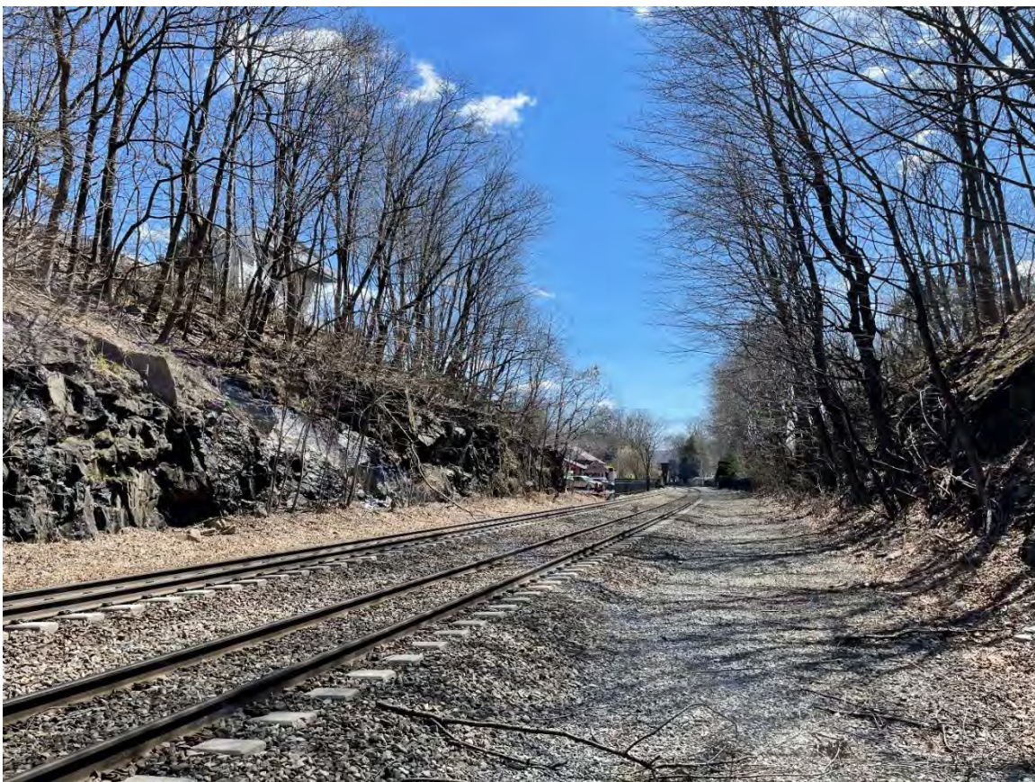
Figure 13: View along southbound tracks looking southeast towards Main Street. Note the steep grade and rock to the right of photo where the trail alignment is proposed to be outside of the MNR clear zone
