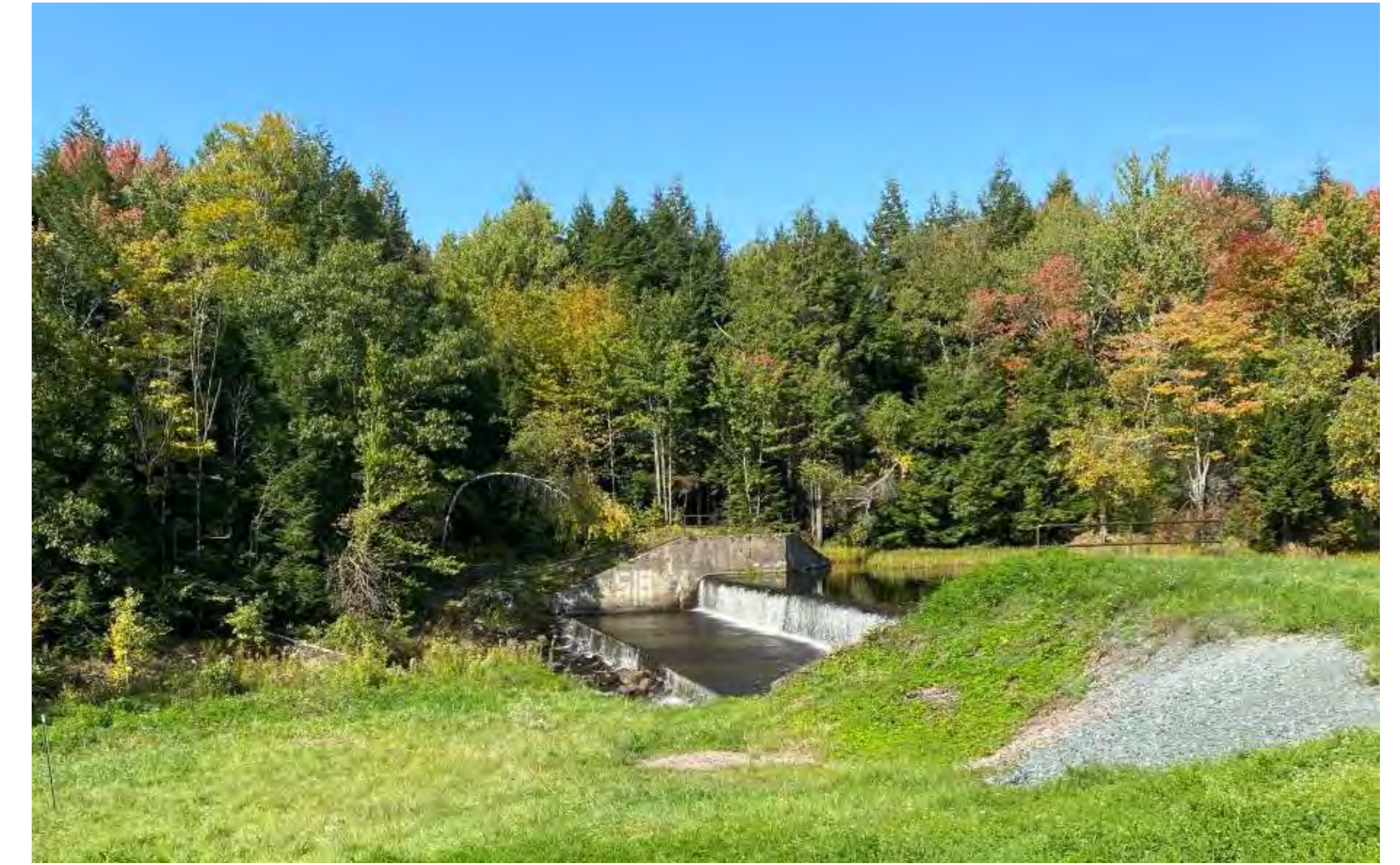
Concrete Spillway Weir and Earth Embankment Dike
