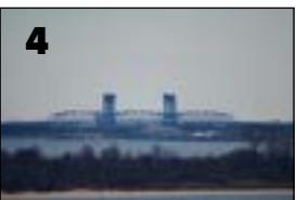
Marine Parkway Bridge
