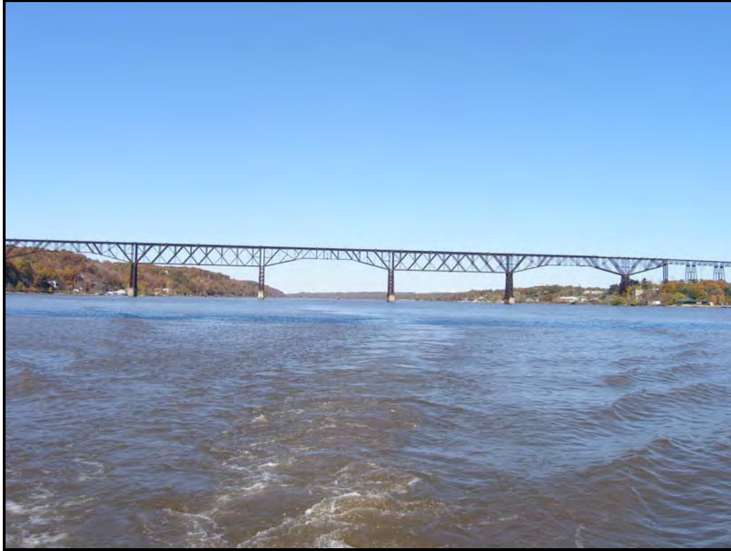
Photo 1 – Overall view of the river spans of the bridge, looking north.
