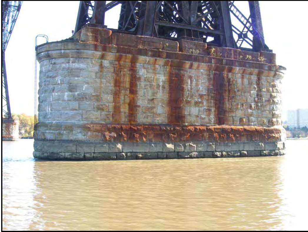
Photo 7 – Pier 3, north and west elevation of the pier.
