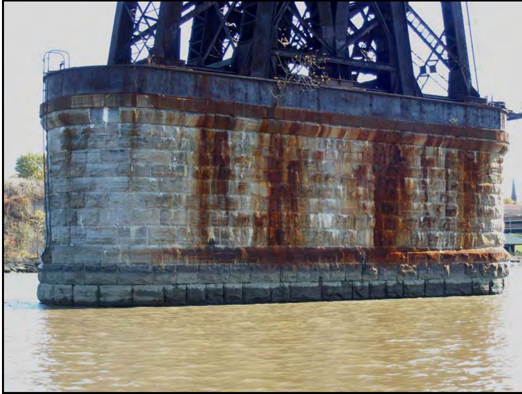
Photo 11 – Pier 5, north and west elevation of the pier.
