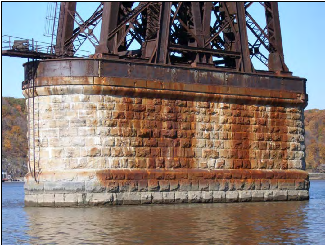
Photo 12 - Pier 5, south and east elevation of the pier.
