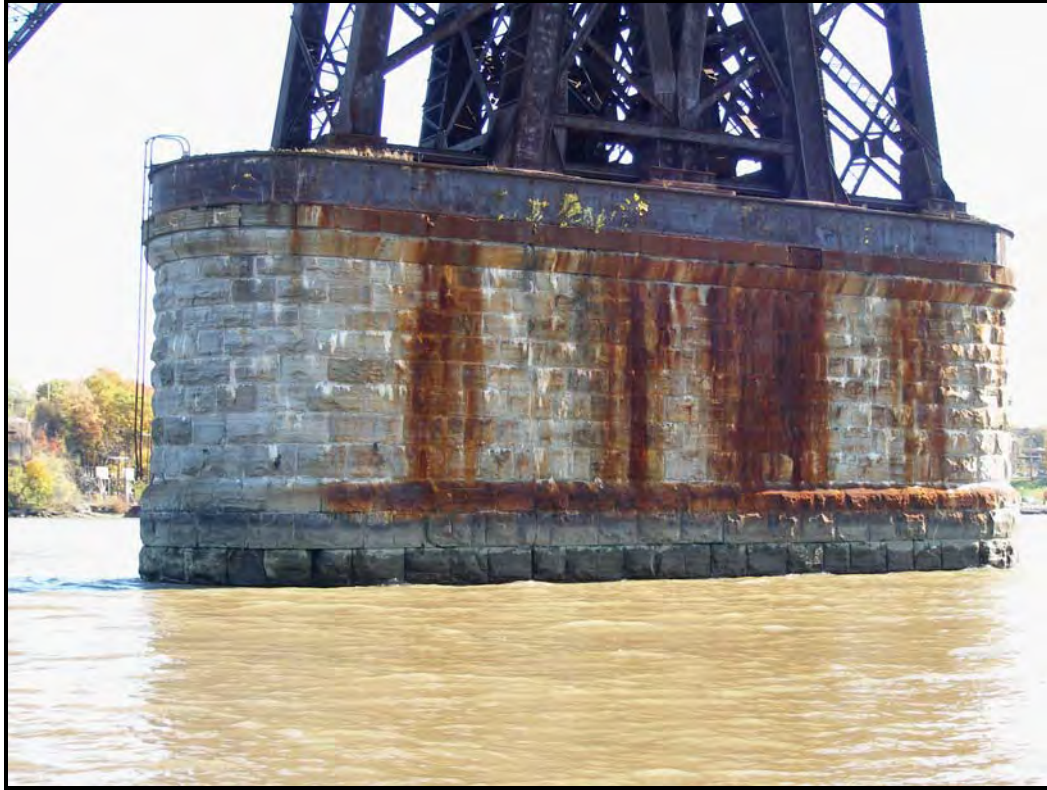
Photo 9 – Pier 4, north and west elevation of the pier.
