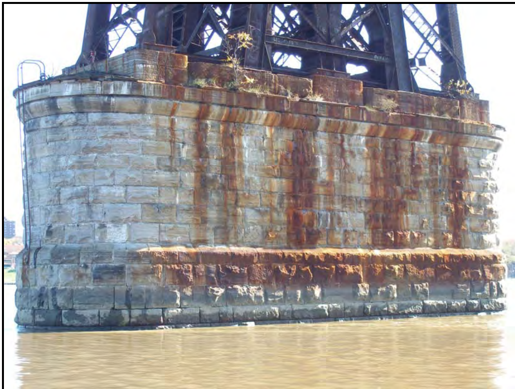
Photo 2 – Pier 2 west and north elevation.
