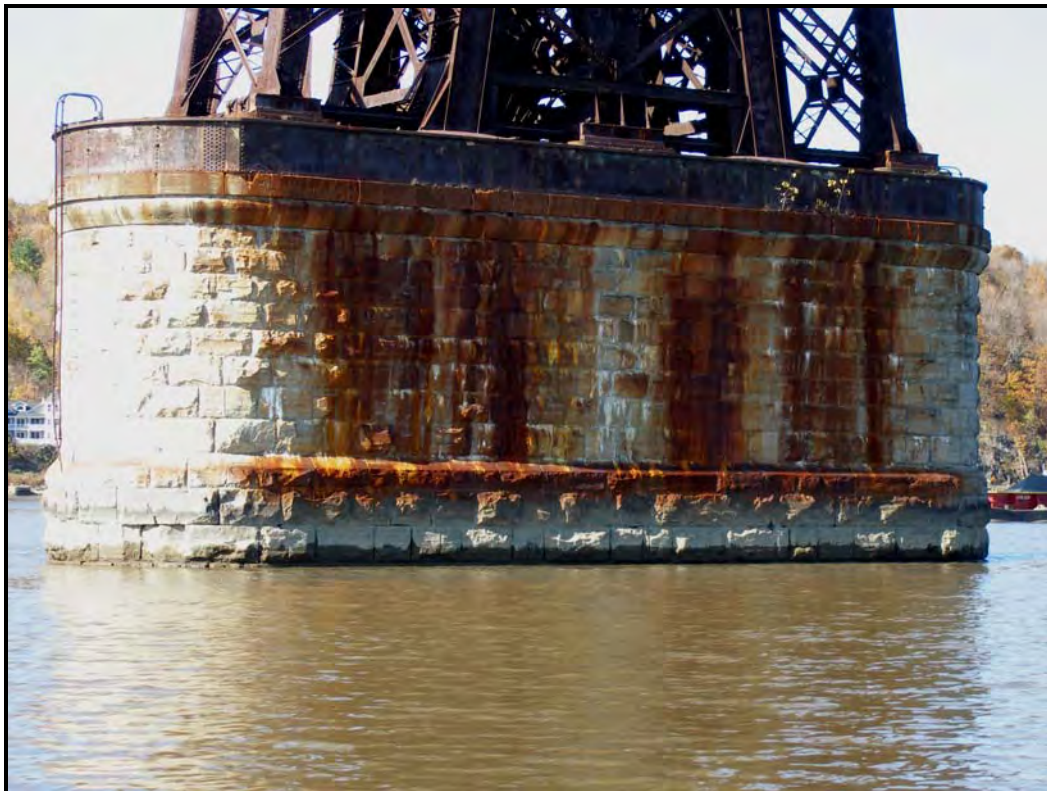
Photo 10 – Pier 4, south and east elevation of the pier.
