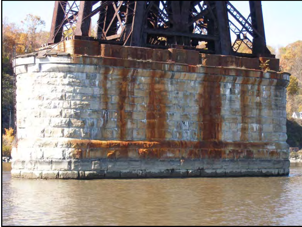
Photo 3 – Pier 2, south and east elevation.
