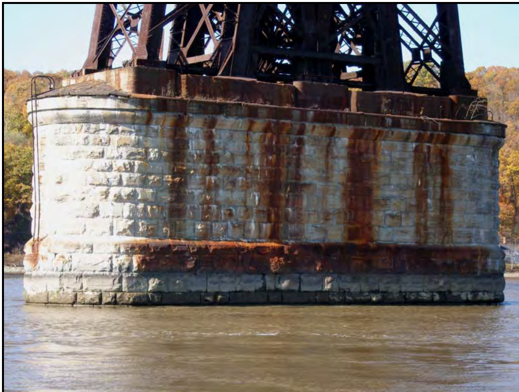
Photo 8 – Pier 3, south and east face of the pier.
