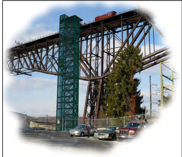
Pier 6 – Along Waterfront
