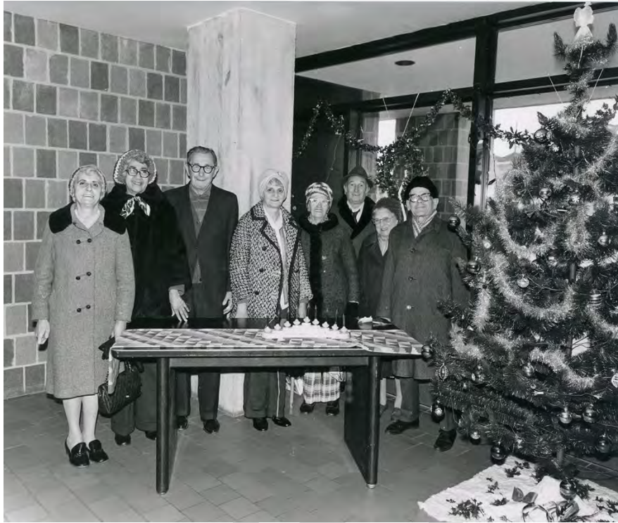
Figure 18: Ca. 1972 interior view of building residents in the lobby. Note the board-formed concrete columns, brick walls, and quarry tile floors. (NYCHA)
