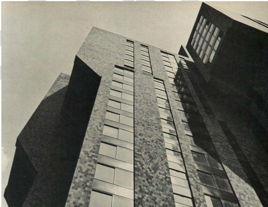
Figure 15: Typical view of the upper floors showing the brown jumbo brick cladding and original sliding windows, 1972. ( Architectural Record )
