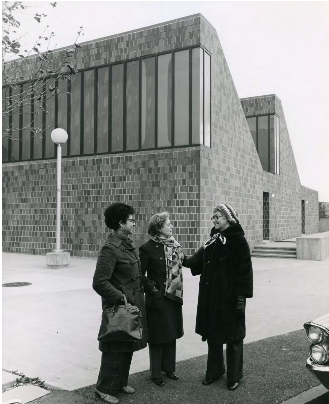
Figure 17: View of the original portion of the community center looking south, ca. 1972. Note the large, north-facing clerestory windows. (NYCHA)
