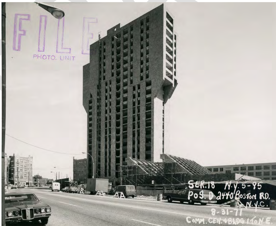
Figure 10: View of the apartment building and community center looking northeast while under construction, August 1971. (NYCHA)
