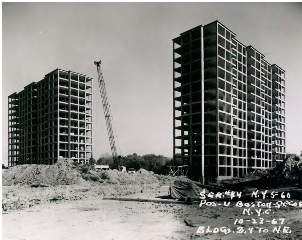
Figure 12: View of Buildings 3 and 4, looking northeast, during construction, October 1967. (NYCHA)
