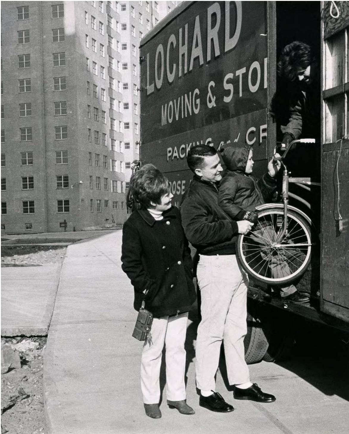
Figure 14: View of a tenant moving into the building, July 1969. (NYCHA)
