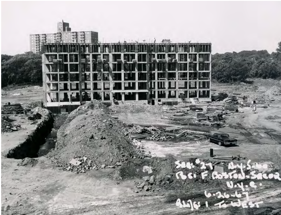
Figure 11: View of Building 1 during construction, June 1967. (NYCHA)
