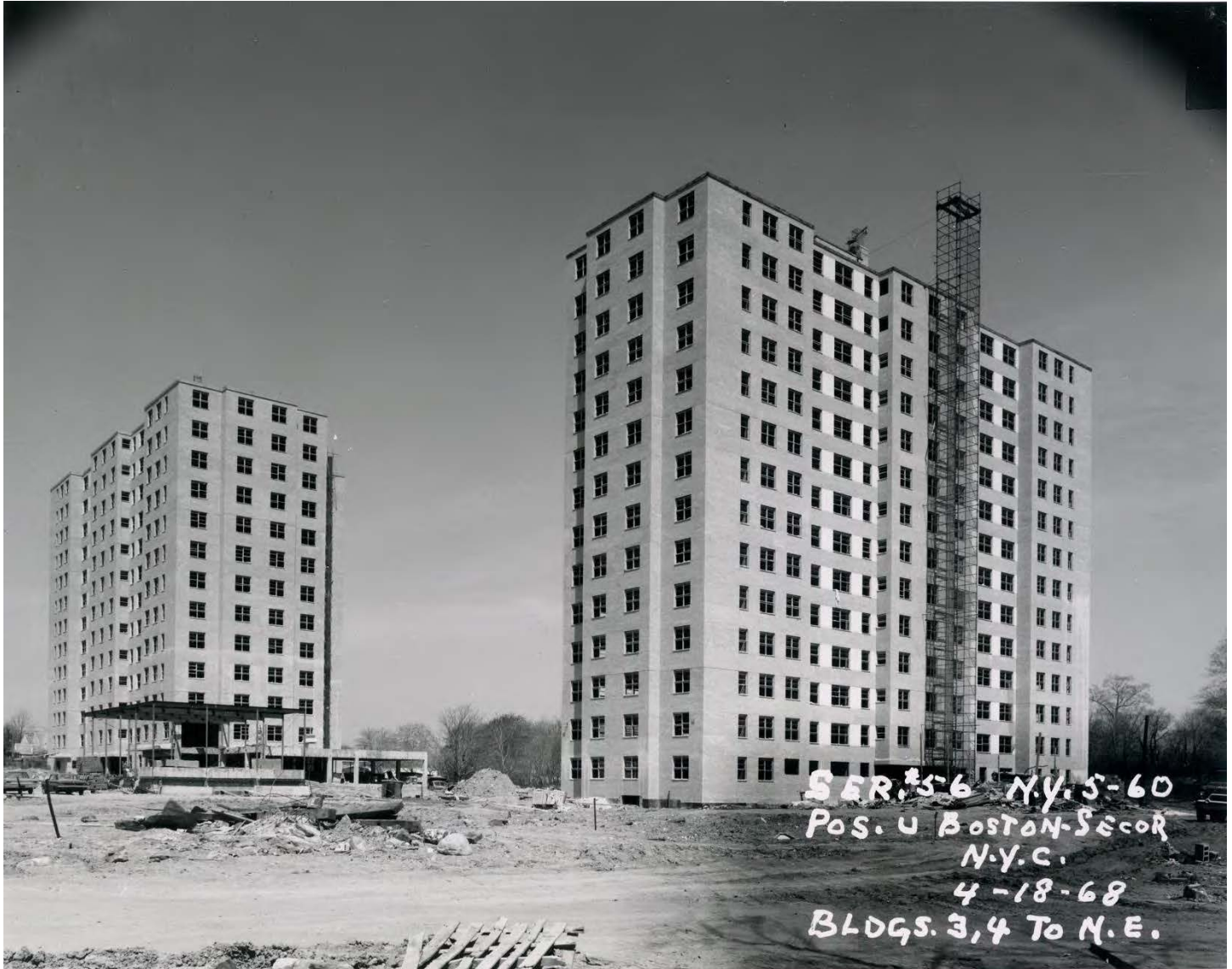
Figure 13: View of Buildings 3 and 4, looking northeast, during construction, April 1968. (NYCHA)
