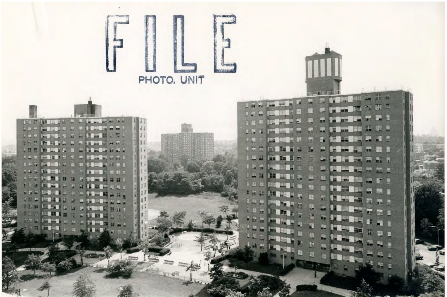
Figure 19: 1978 view of Buildings 1 and 2 looking west. Note the octagonal buff-brick water tower atop Building 2. (NYHCA)
