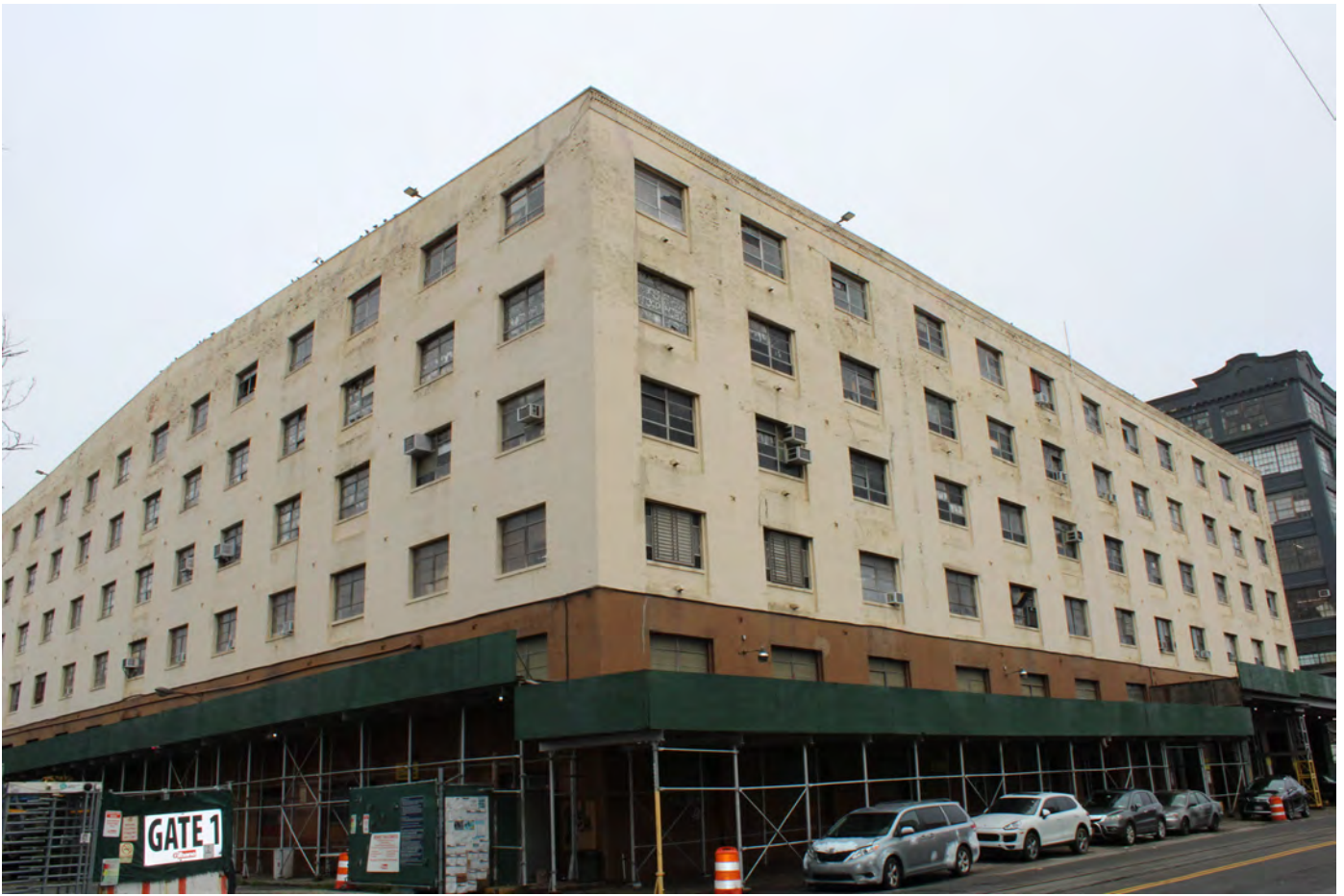
NY_Kings County_Bush Terminal_0055
