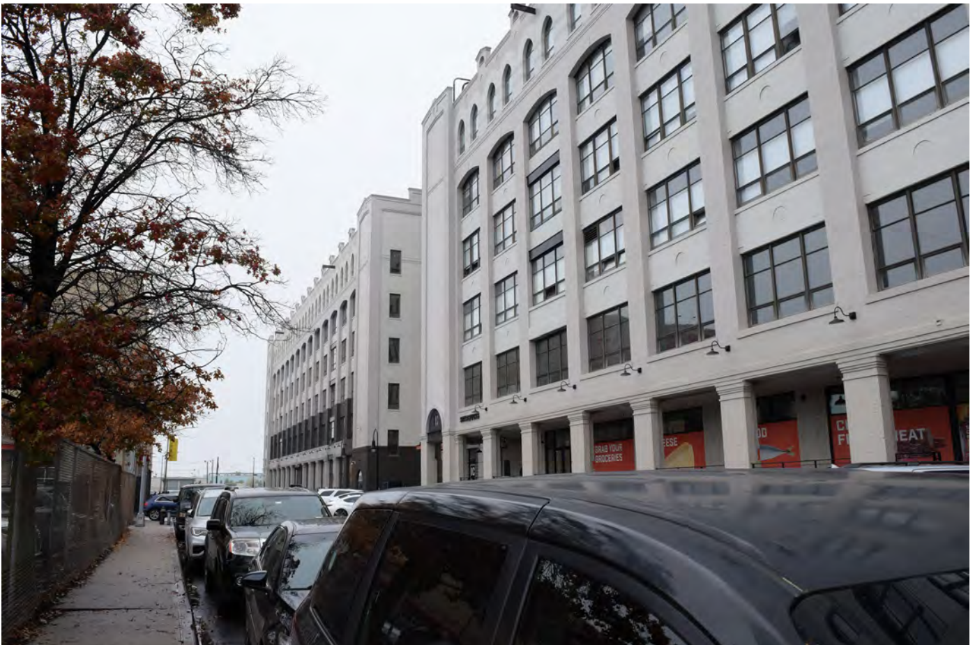
NY_Kings County_Bush Terminal_0064
