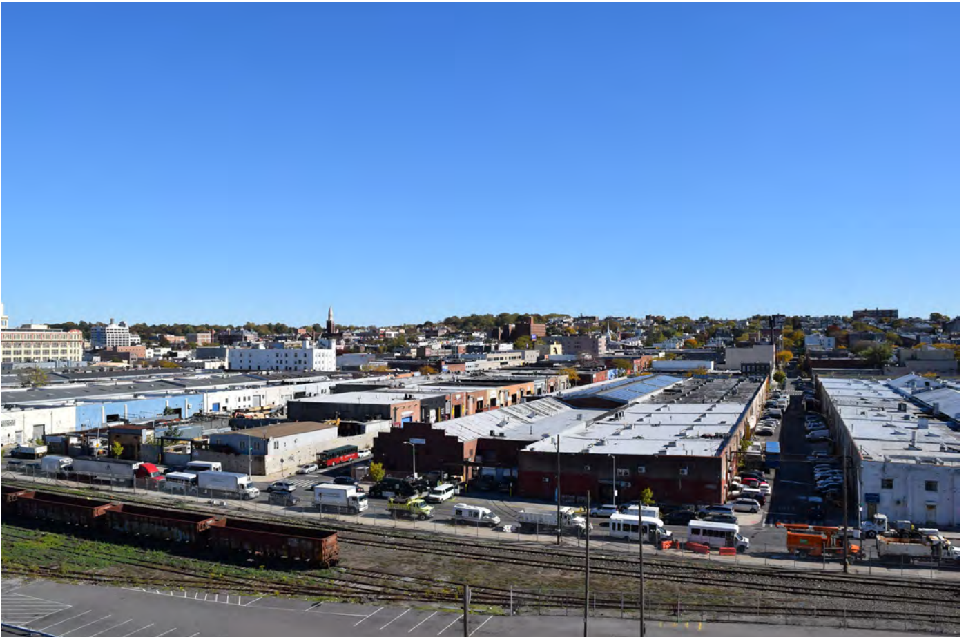
NY_Kings County_Bush Terminal_0036
