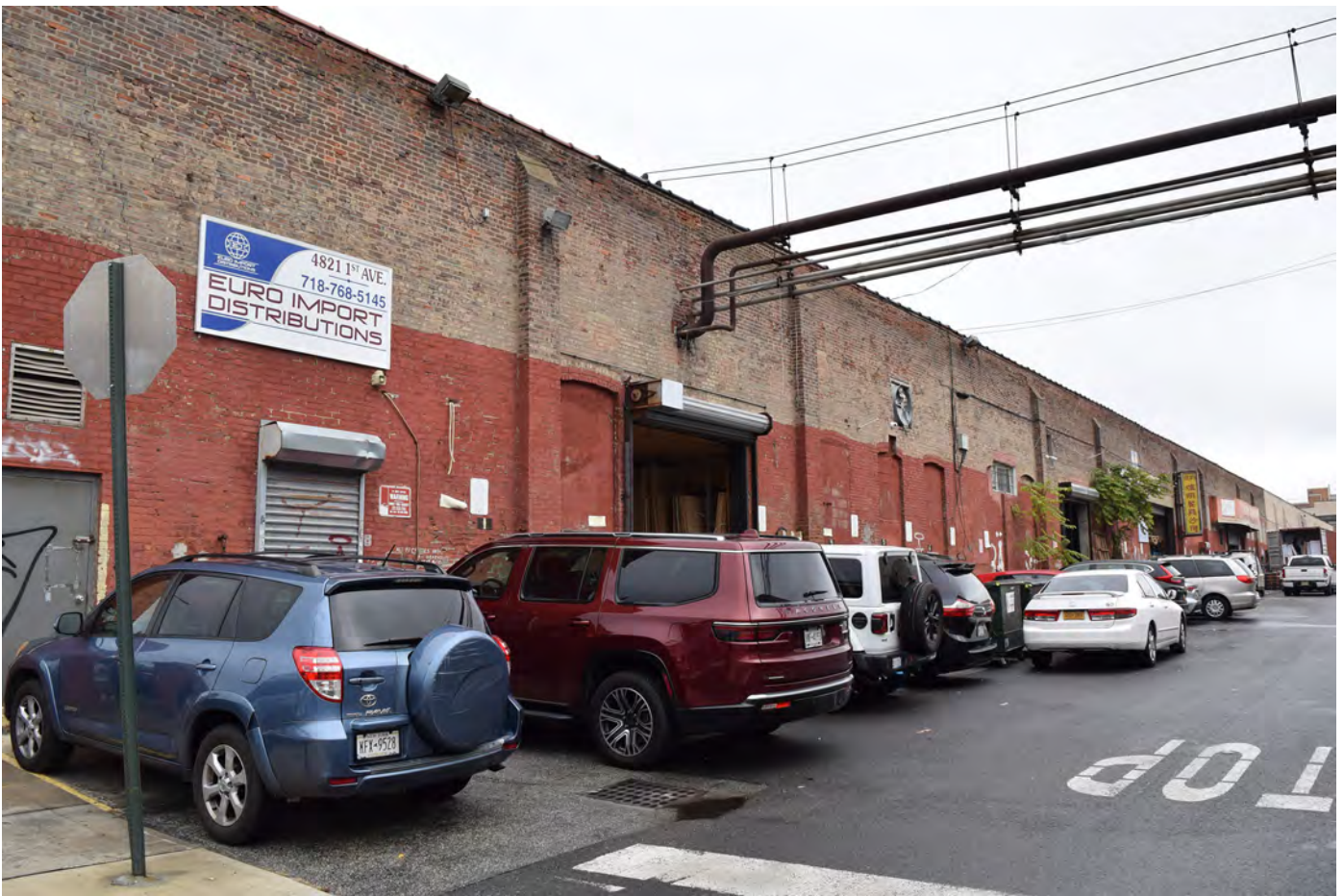
NY_Kings County_Bush Terminal_0005
