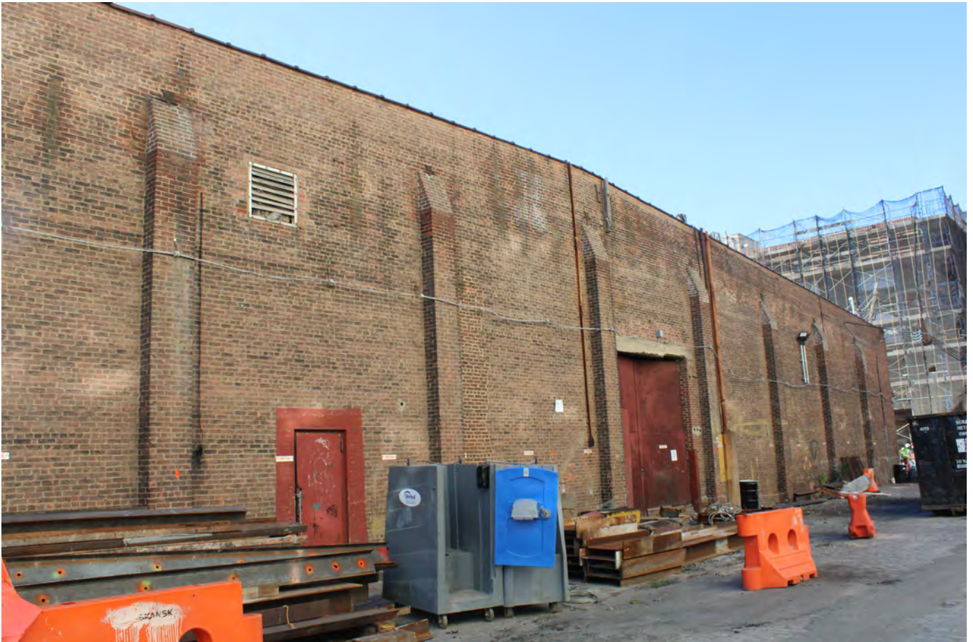
NY_Kings County_Bush Terminal_0054
