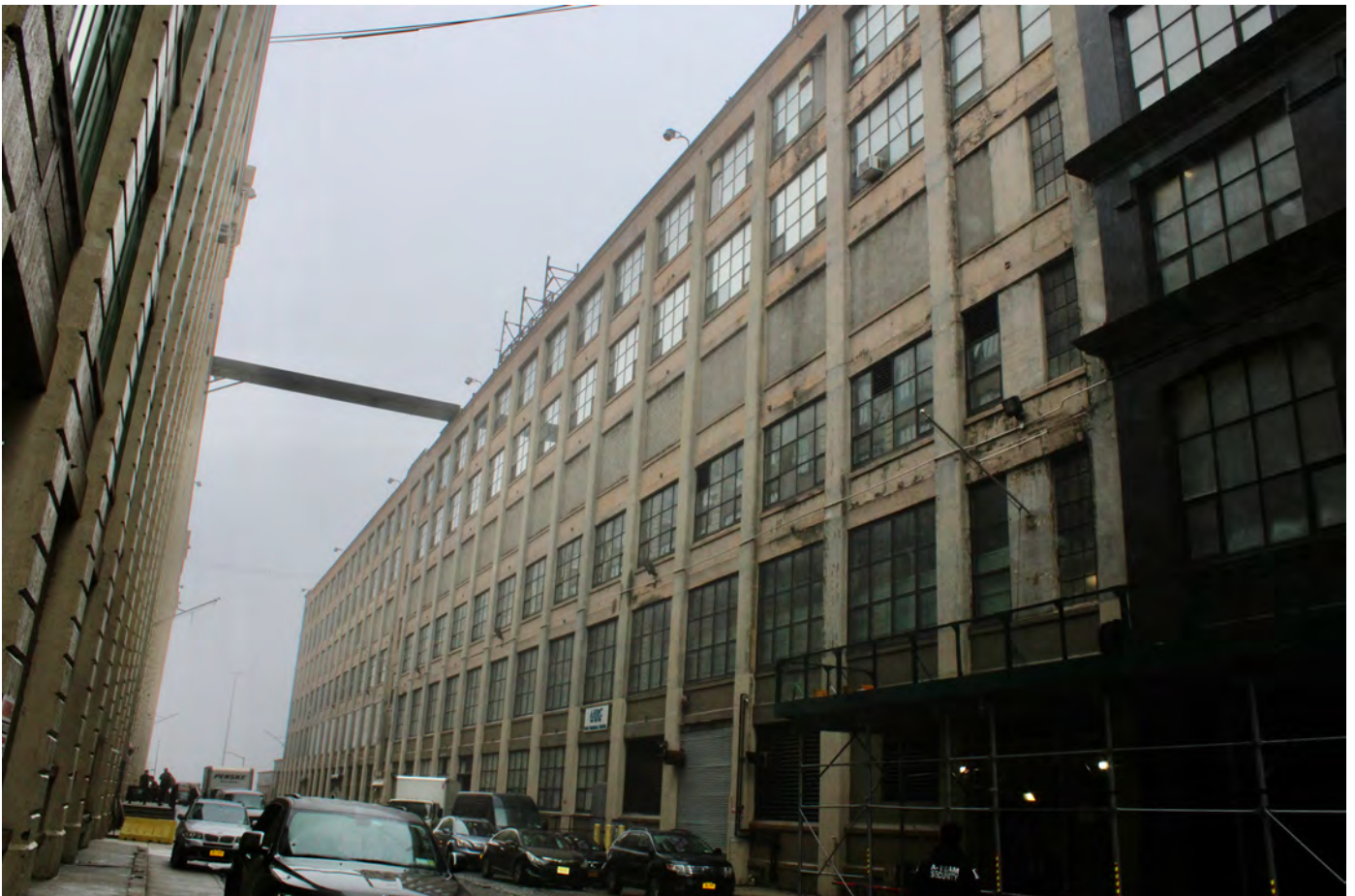
NY_Kings County_Bush Terminal_0074
