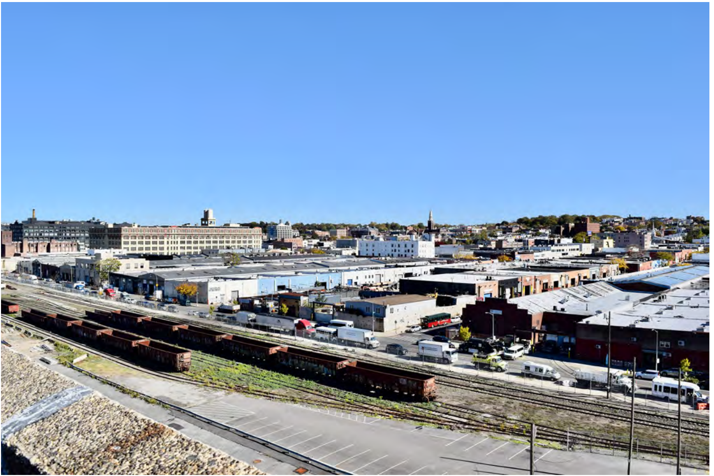
NY_Kings County_Bush Terminal_0035
