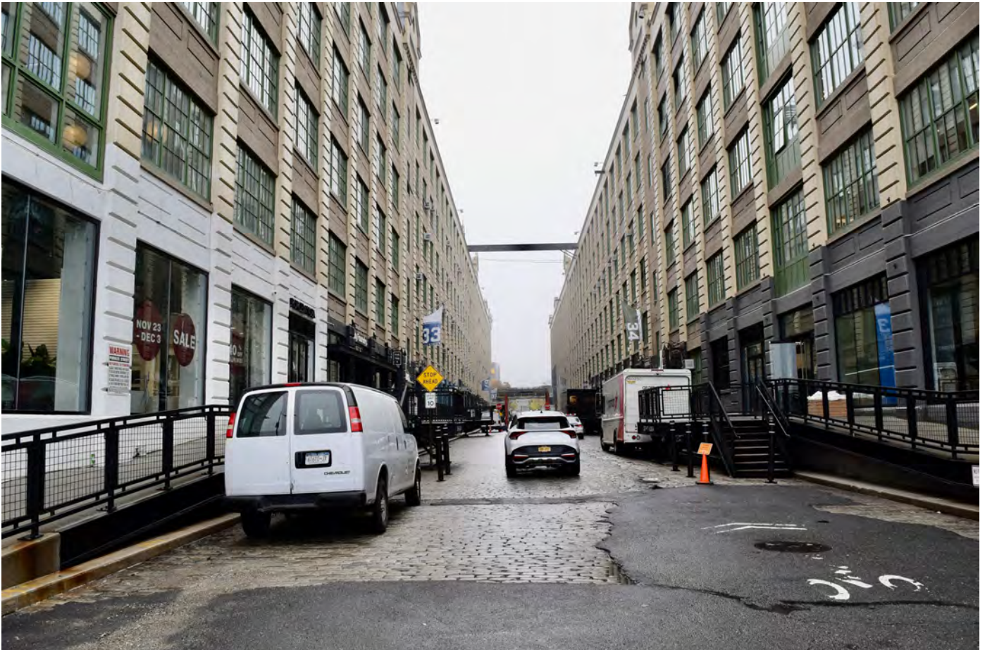
NY_Kings County_Bush Terminal_0070
