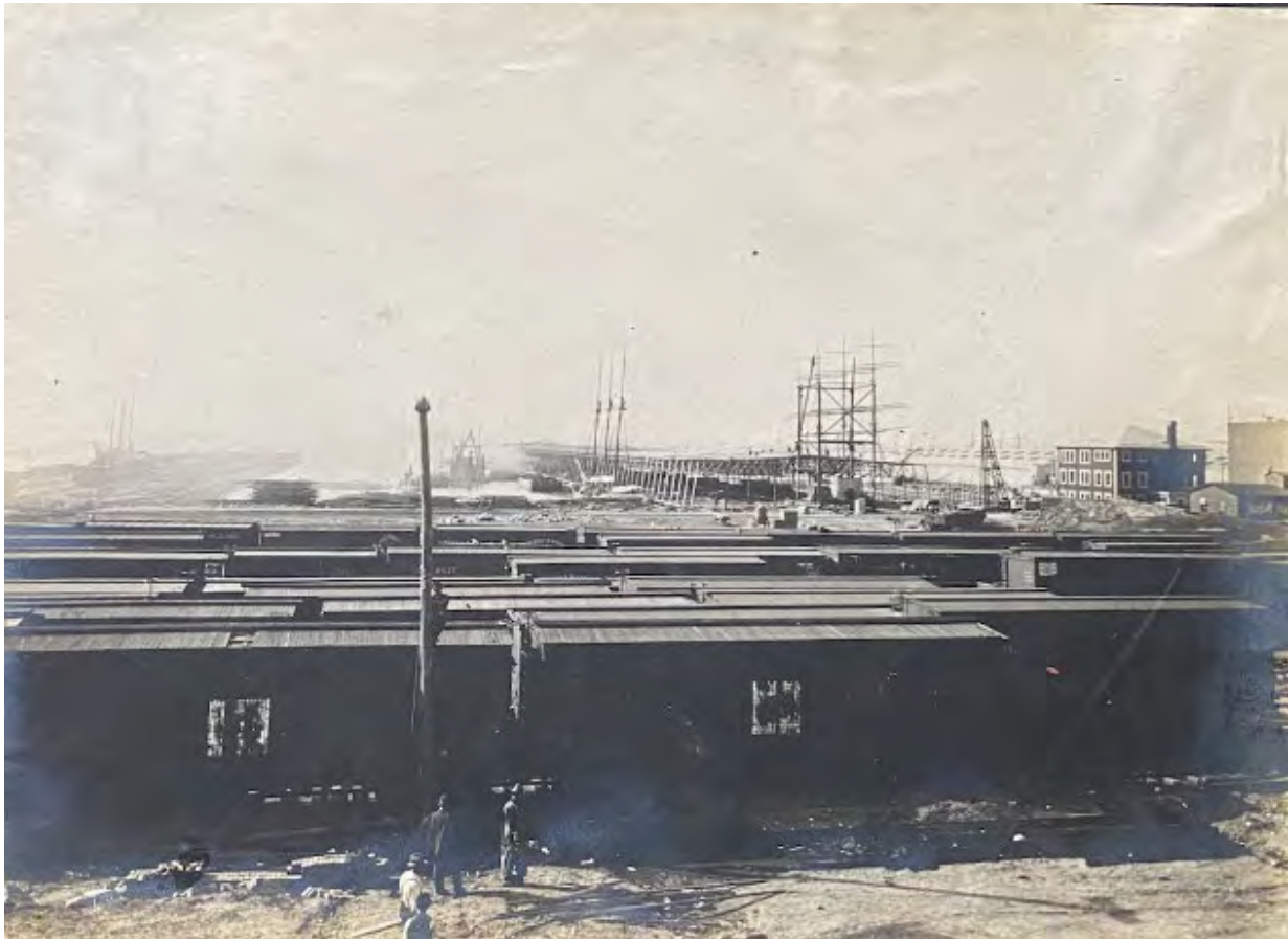
Figure 11. View from the Railroad Yard looking at the construction of Pier 5 April 1, 1903. Courtesy of House of Mirth.
