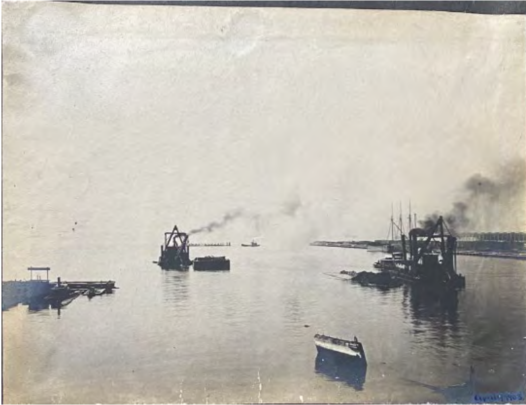
Figure 7. Beginning construction of Pier 3 April 9, 1903. Courtesy of House of Mirth.
