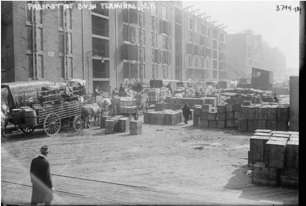
Figure 5. Warehouses along the waterfront, likely Unit E & F ca. 1915. Library of Congress.
