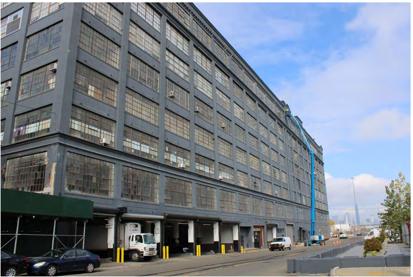
NY_Kings County_Bush Terminal_0057
