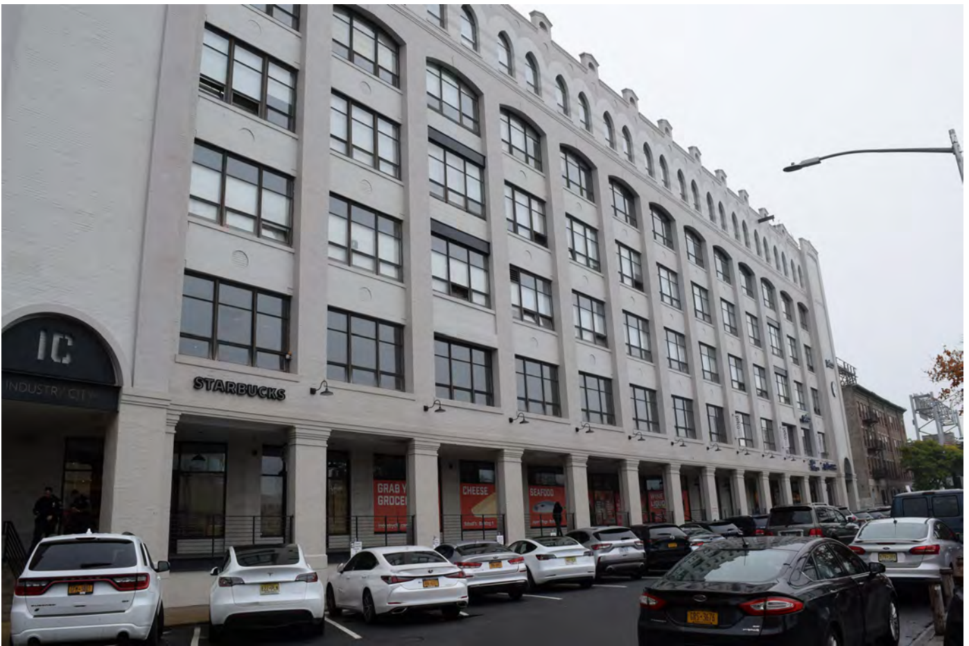
NY_Kings County_Bush Terminal_0063
