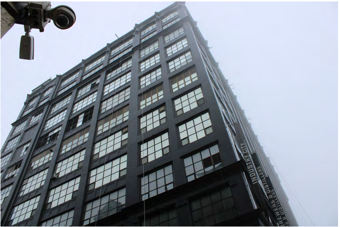
NY_Kings County_Bush Terminal_0079
