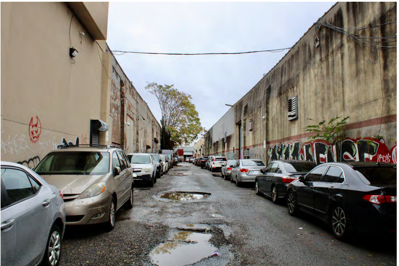
NY_Kings County_Bush Terminal_0033
