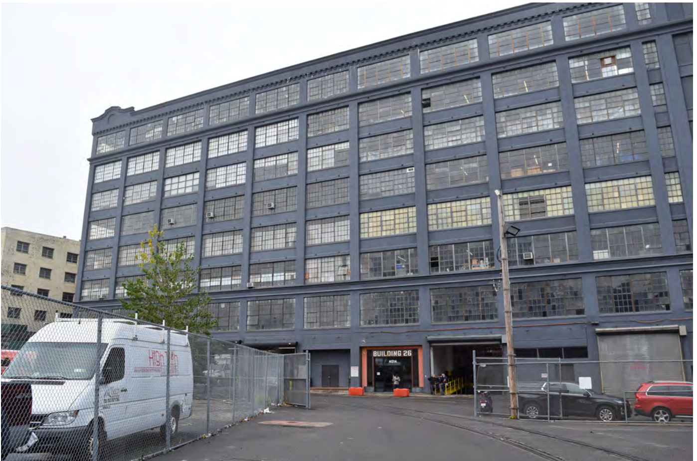
NY_Kings County_Bush Terminal_0058
