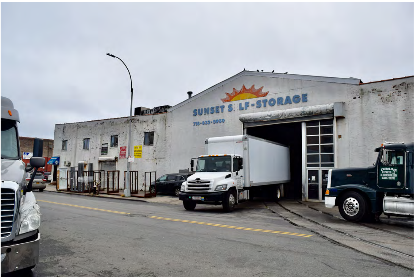
NY_Kings County_Bush Terminal_0003
