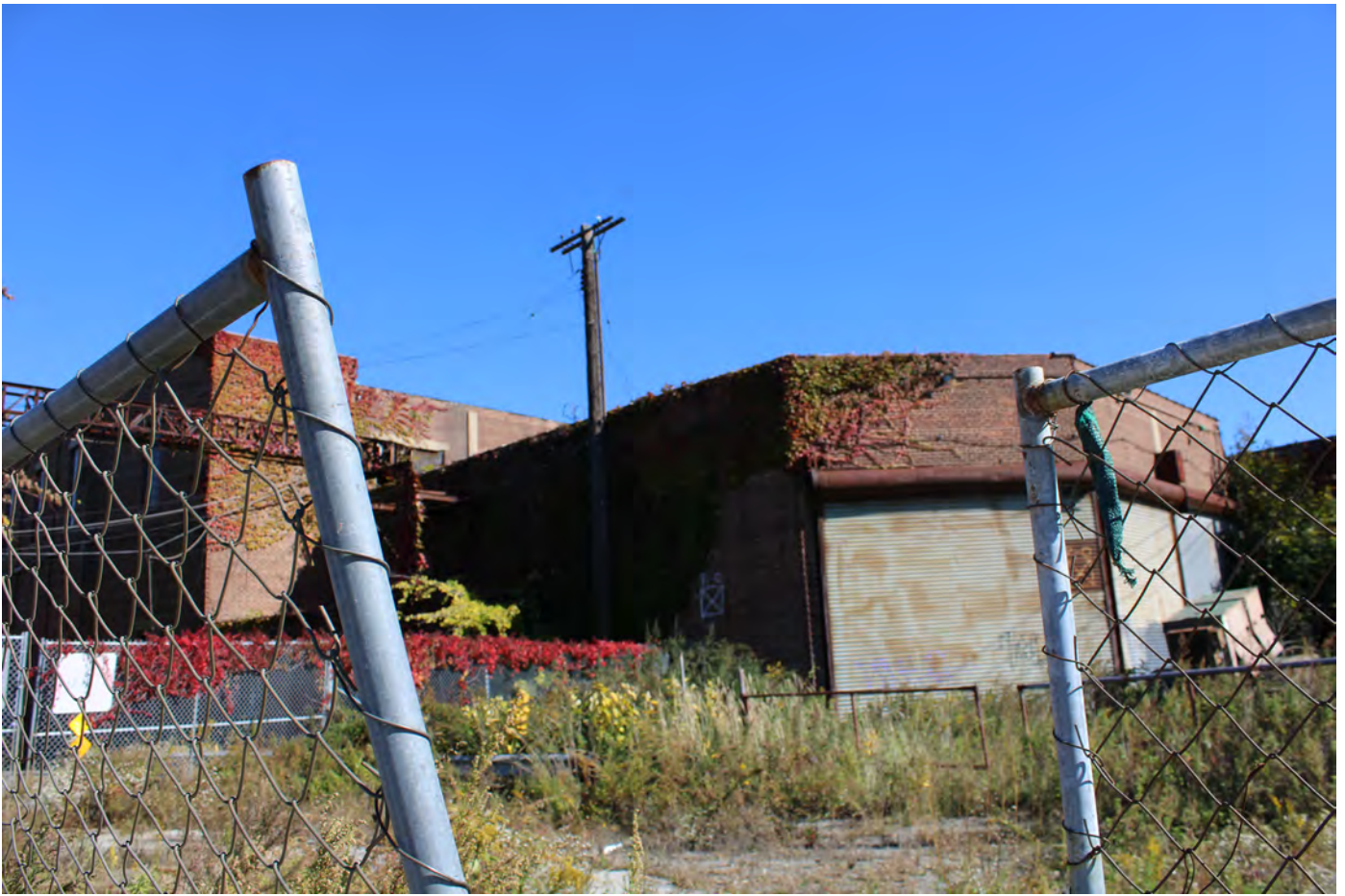
NY_Kings County_Bush Terminal_0037
