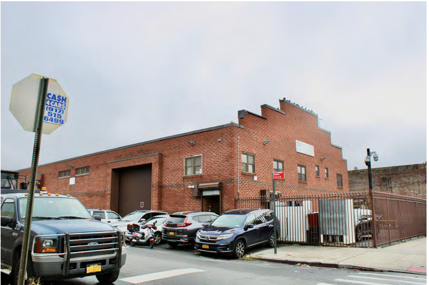
NY_Kings County_Bush Terminal_0017
