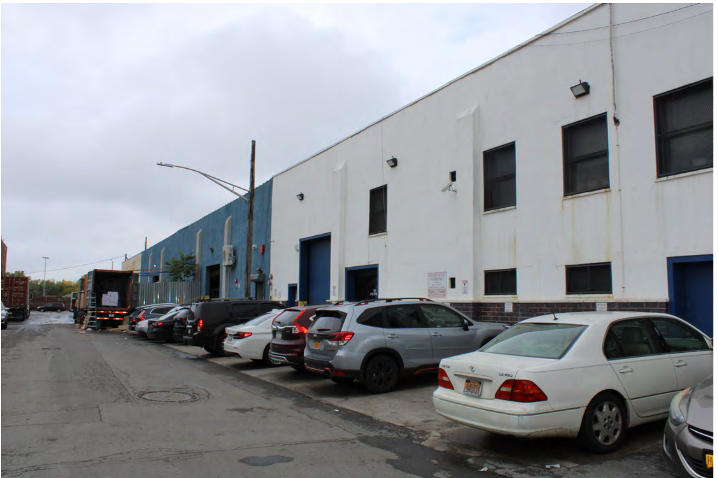
NY_Kings County_Bush Terminal_0023
