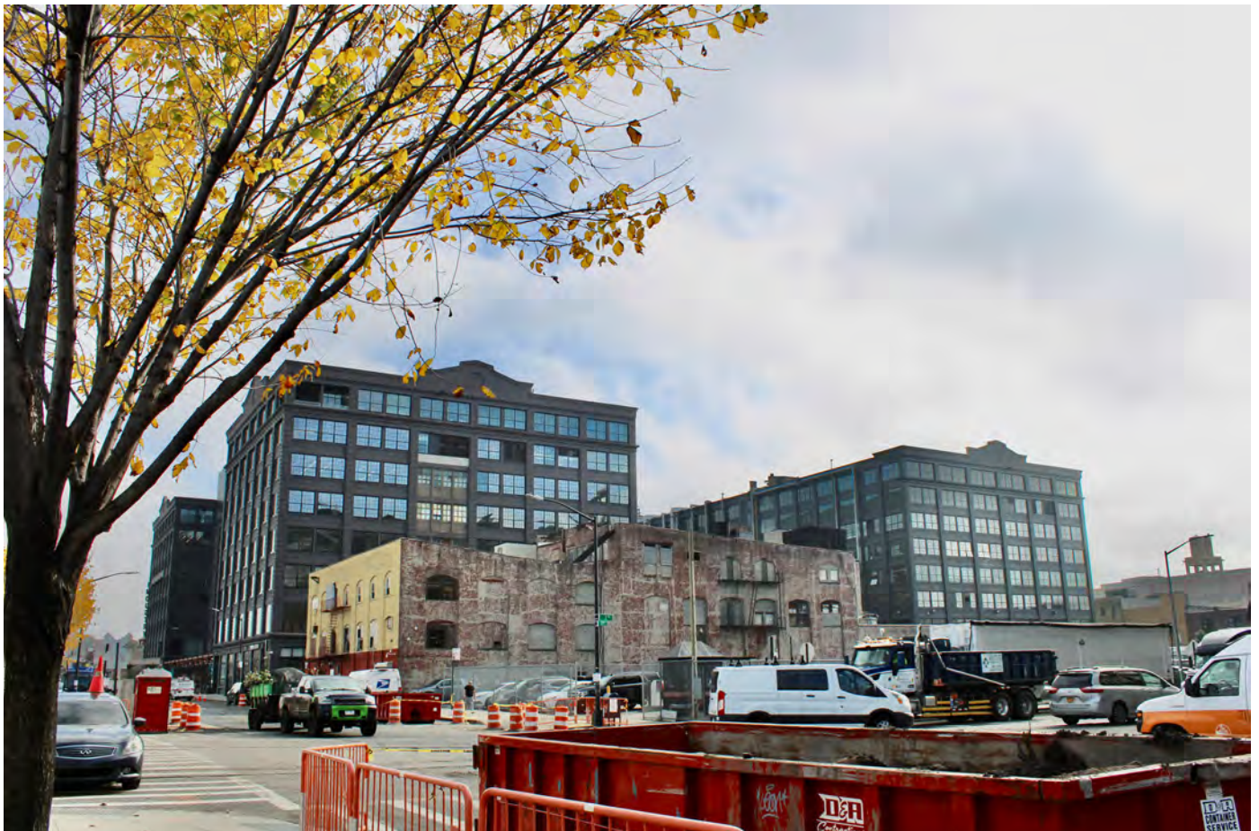
NY_Kings County_Bush Terminal_0060
