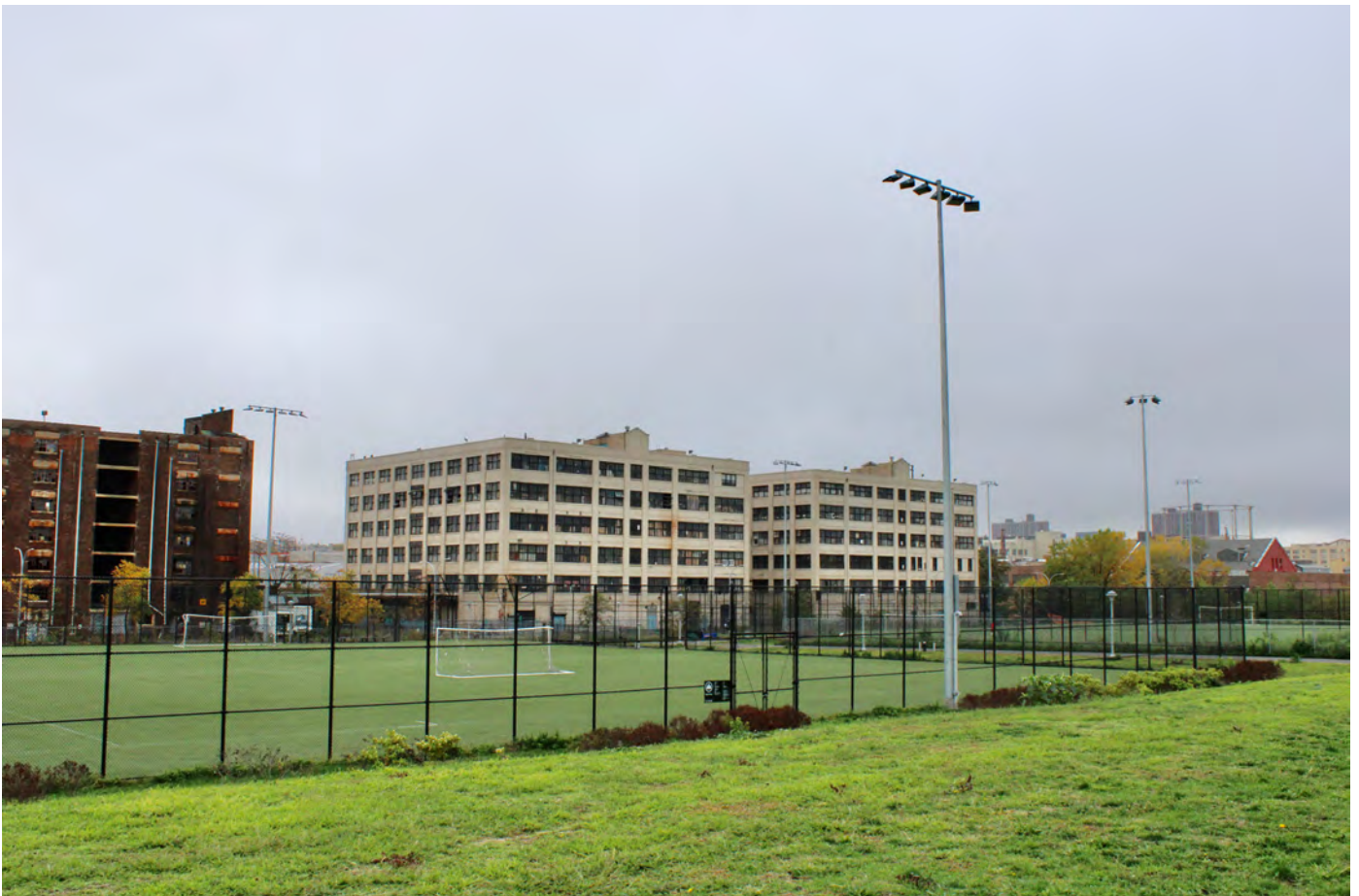
NY_Kings County_Bush Terminal_0040
