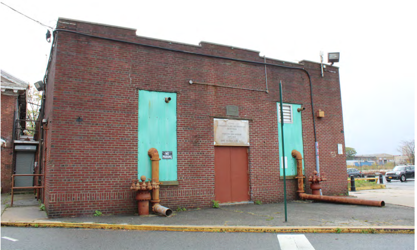
NY_Kings County_Bush Terminal_0044
