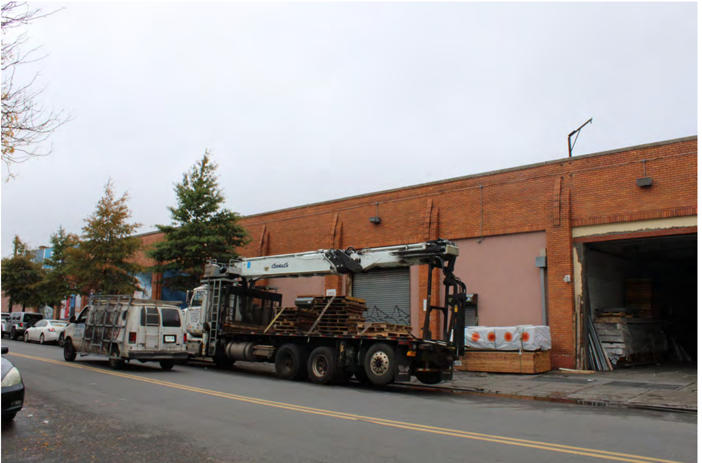
NY_Kings County_Bush Terminal_0026
