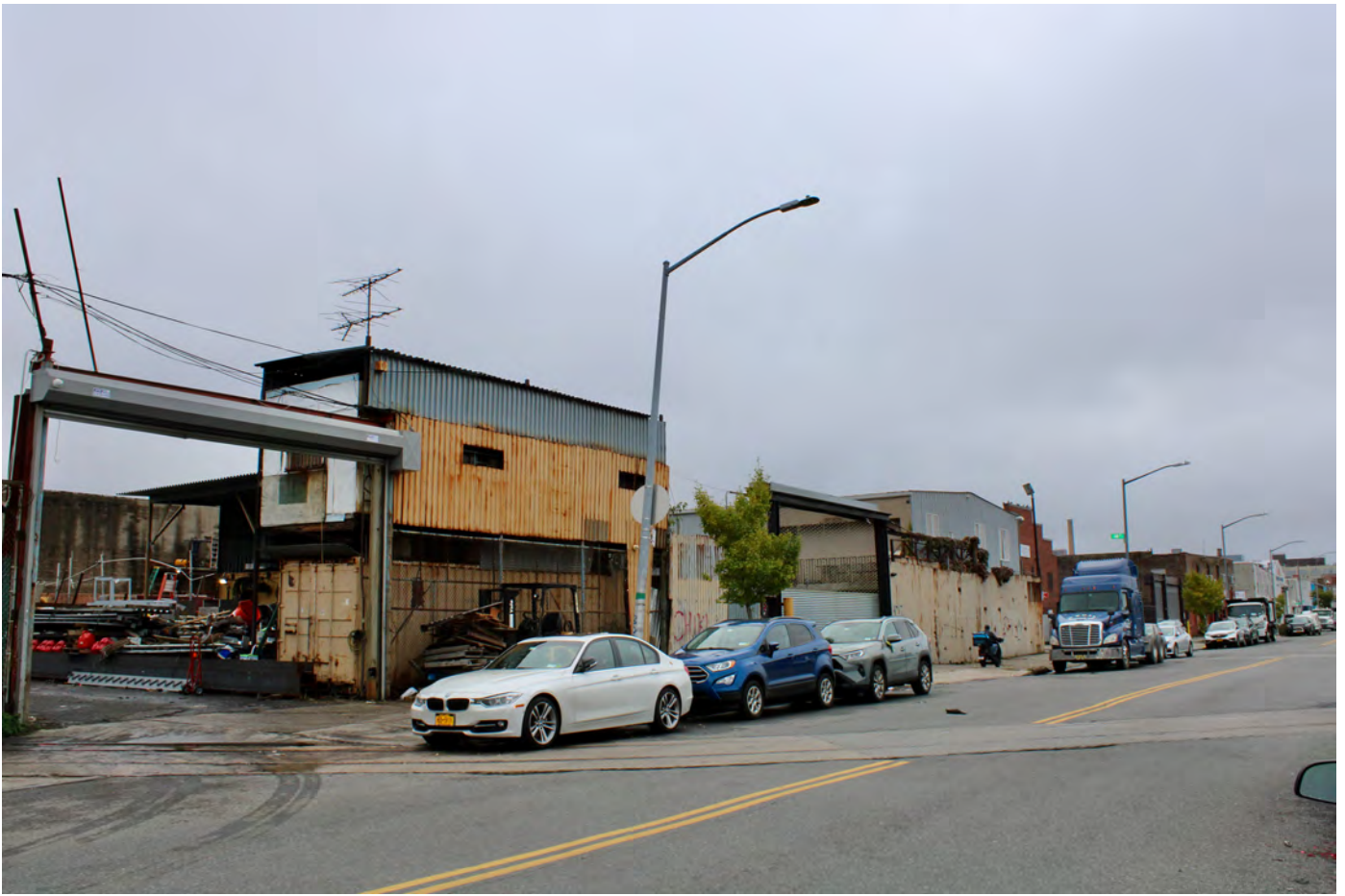
NY_Kings County_Bush Terminal_0019
