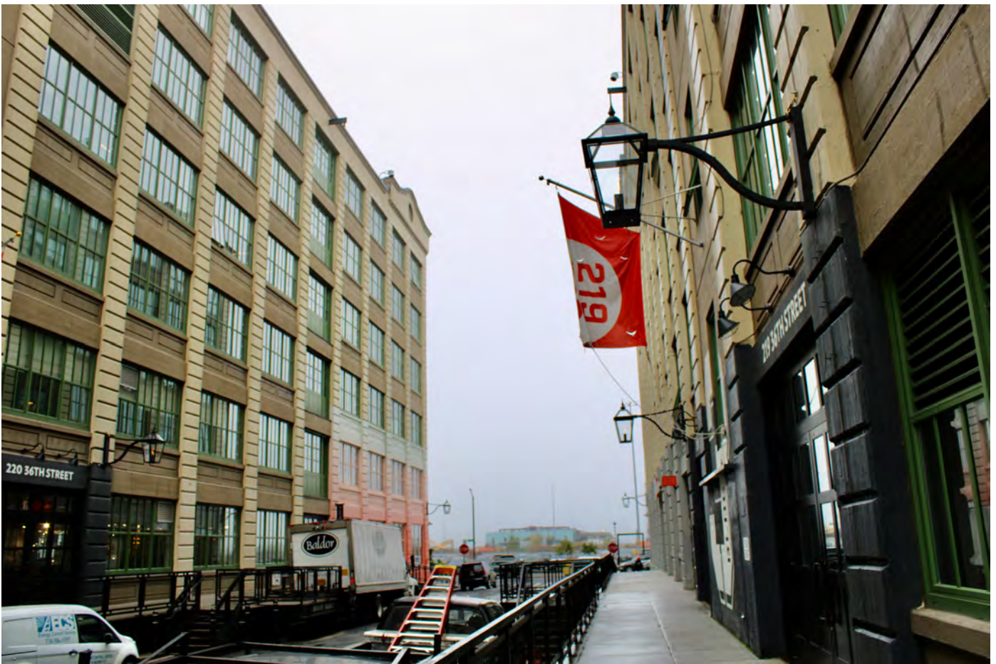
NY_Kings County_Bush Terminal_0075
