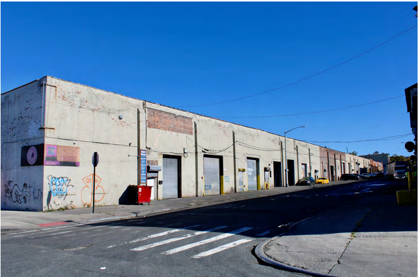
NY_Kings County_Bush Terminal_0002
