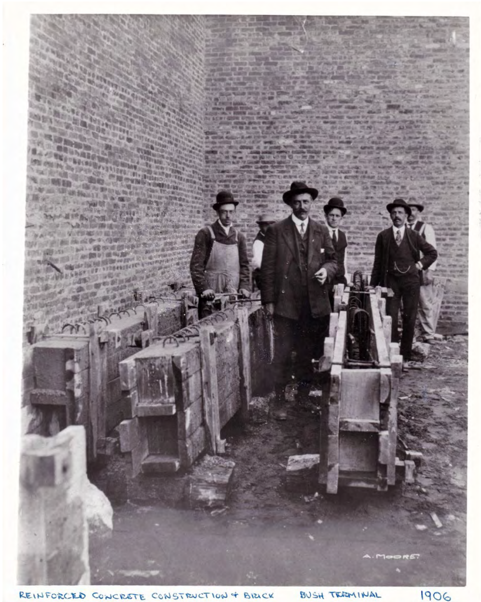
Figure 14. Reinforced Concrete Construction 1906. Courtesy of Sunset Park History.
