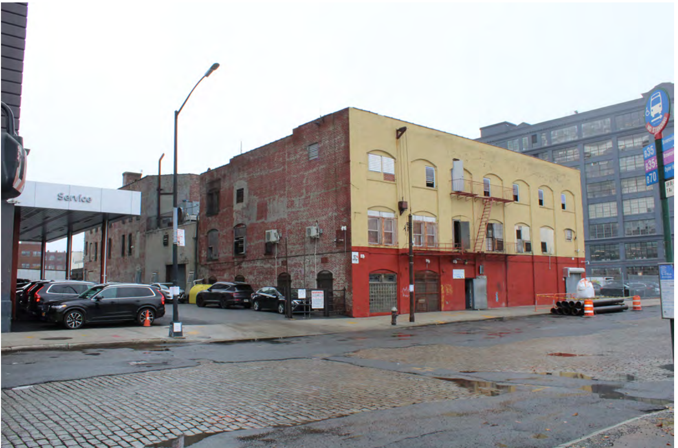
NY_Kings County_Bush Terminal_0062
