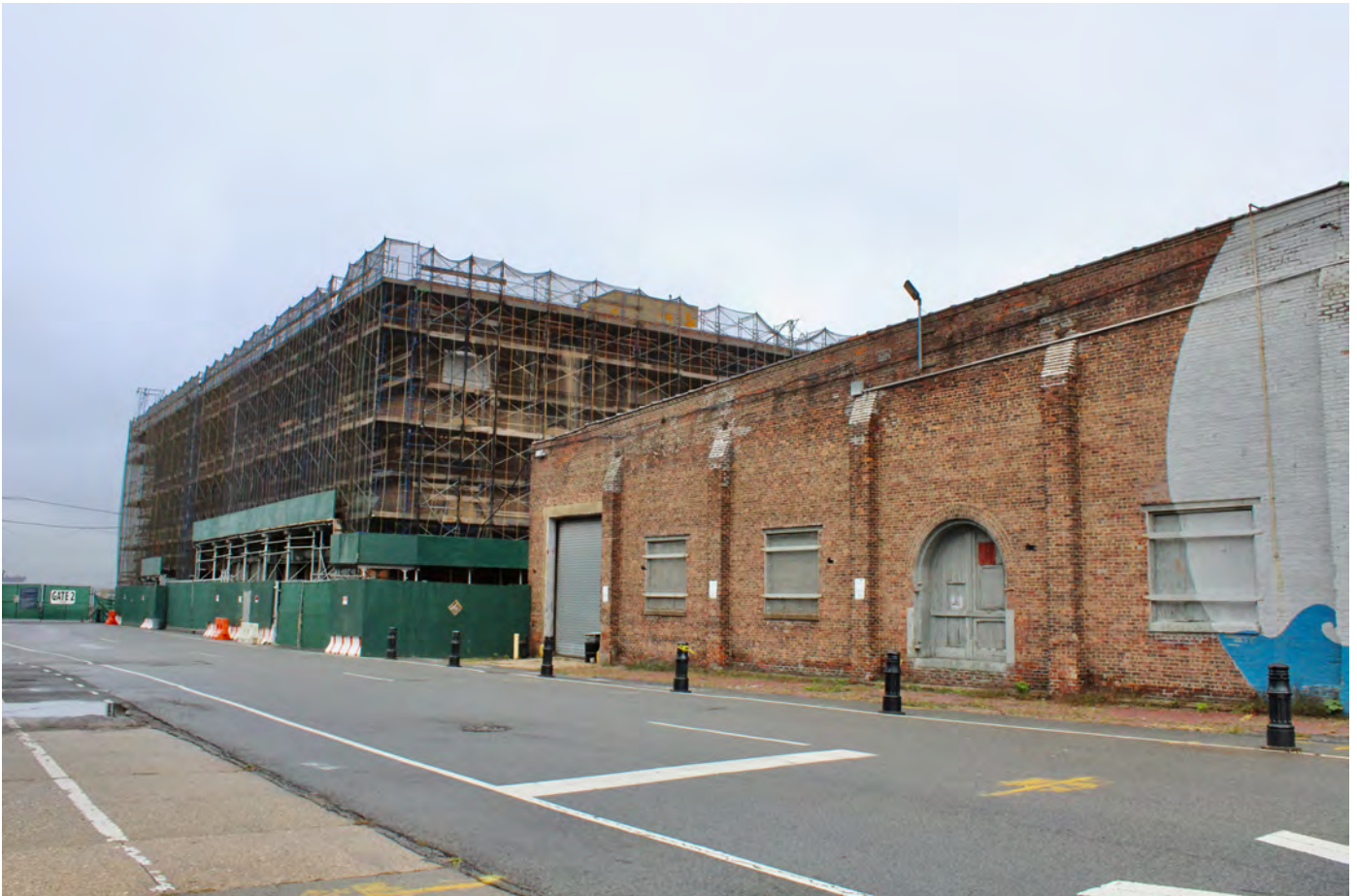
NY_Kings County_Bush Terminal_0056
