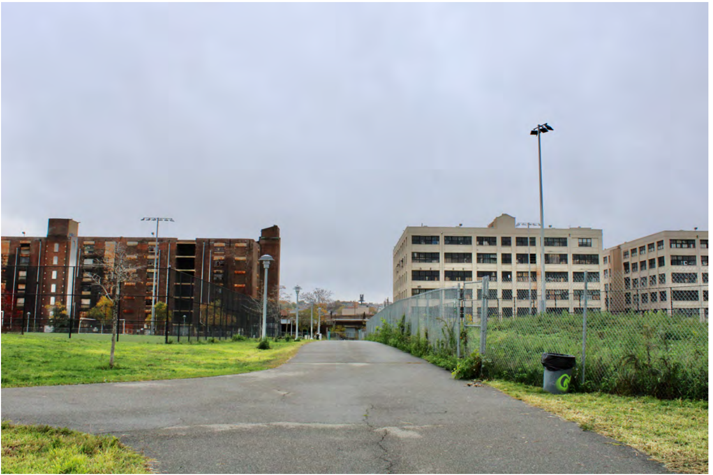
NY_Kings County_Bush Terminal_0039
