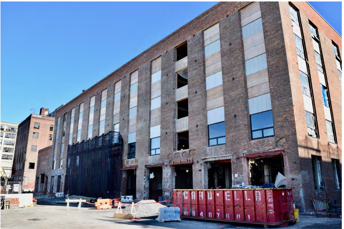
NY_Kings County_Bush Terminal_0053
