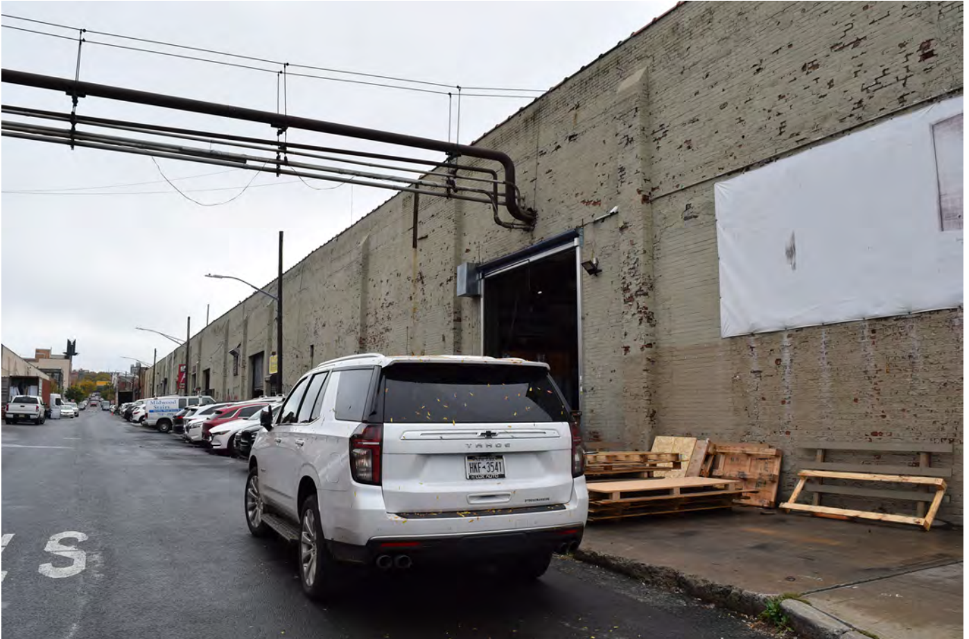
NY_Kings County_Bush Terminal_0006
