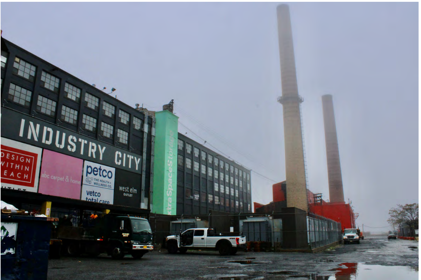
NY_Kings County_Bush Terminal_0081
