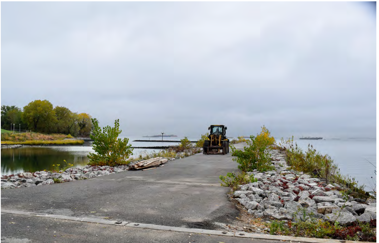
NY_Kings County_Bush Terminal_0050
