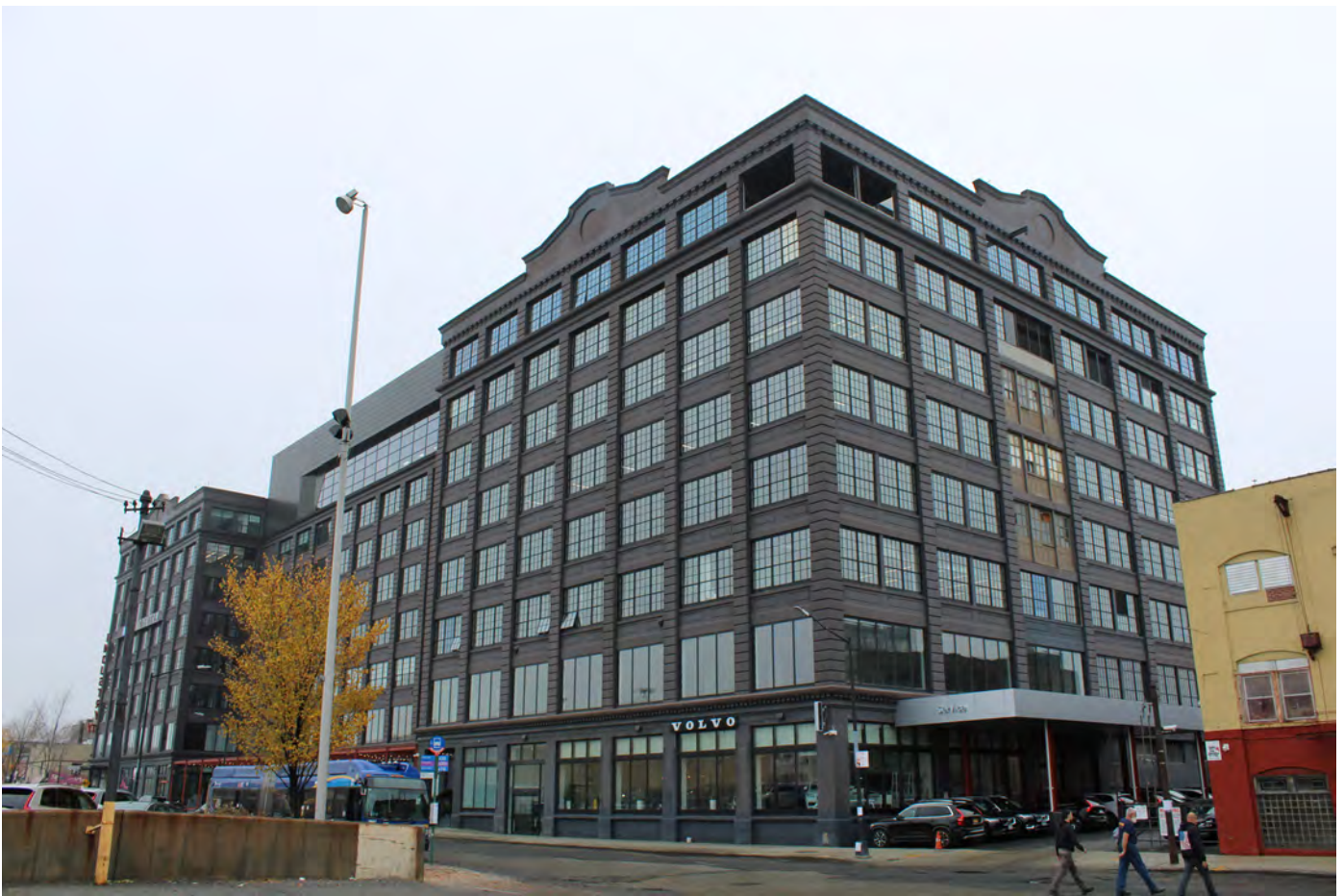
NY_Kings County_Bush Terminal_0061
