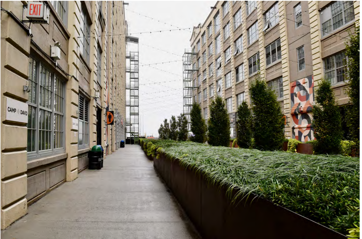
NY_Kings County_Bush Terminal_0072
