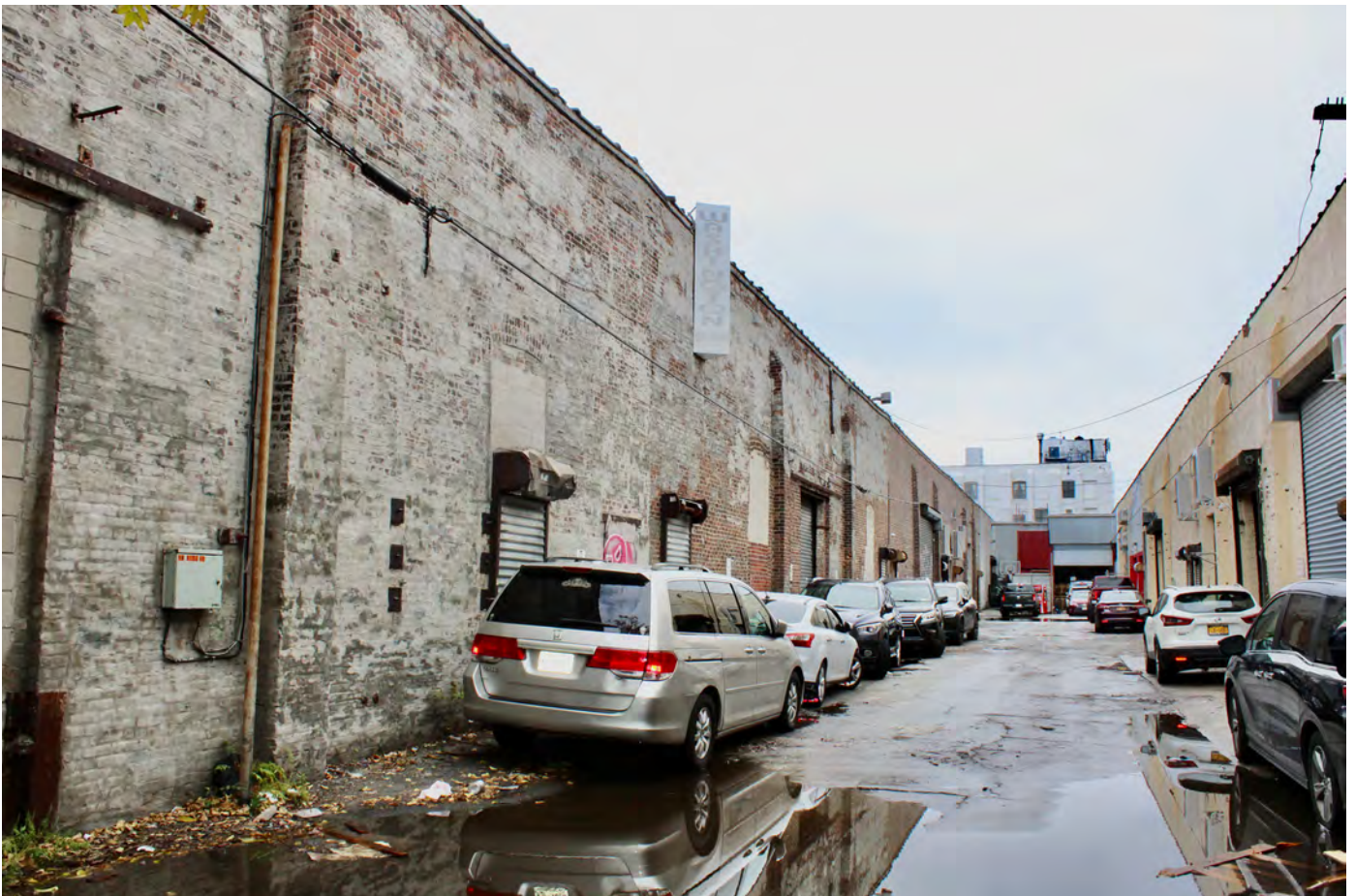
NY_Kings County_Bush Terminal_0032
