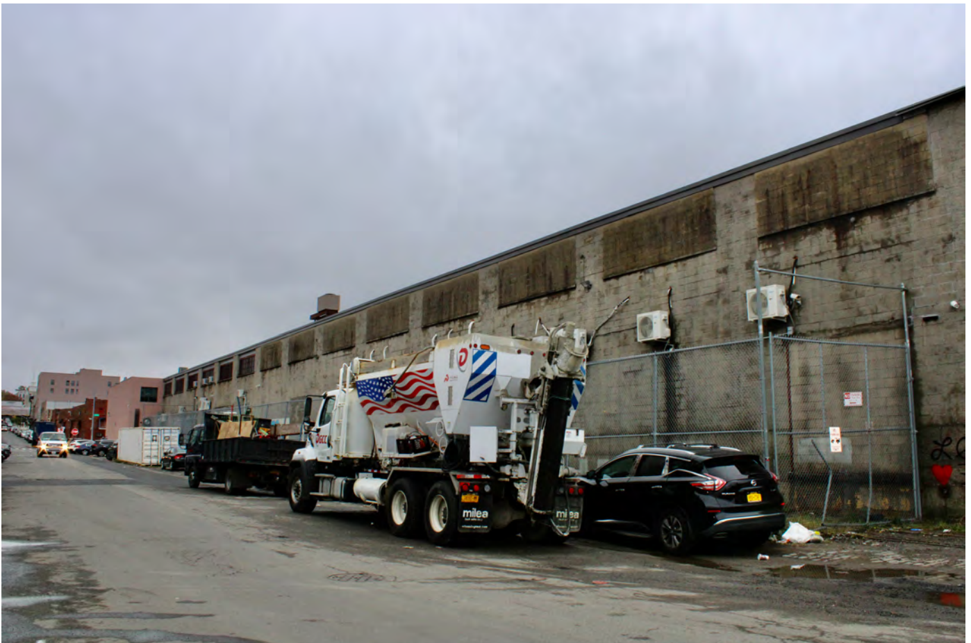
NY_Kings County_Bush Terminal_0022
