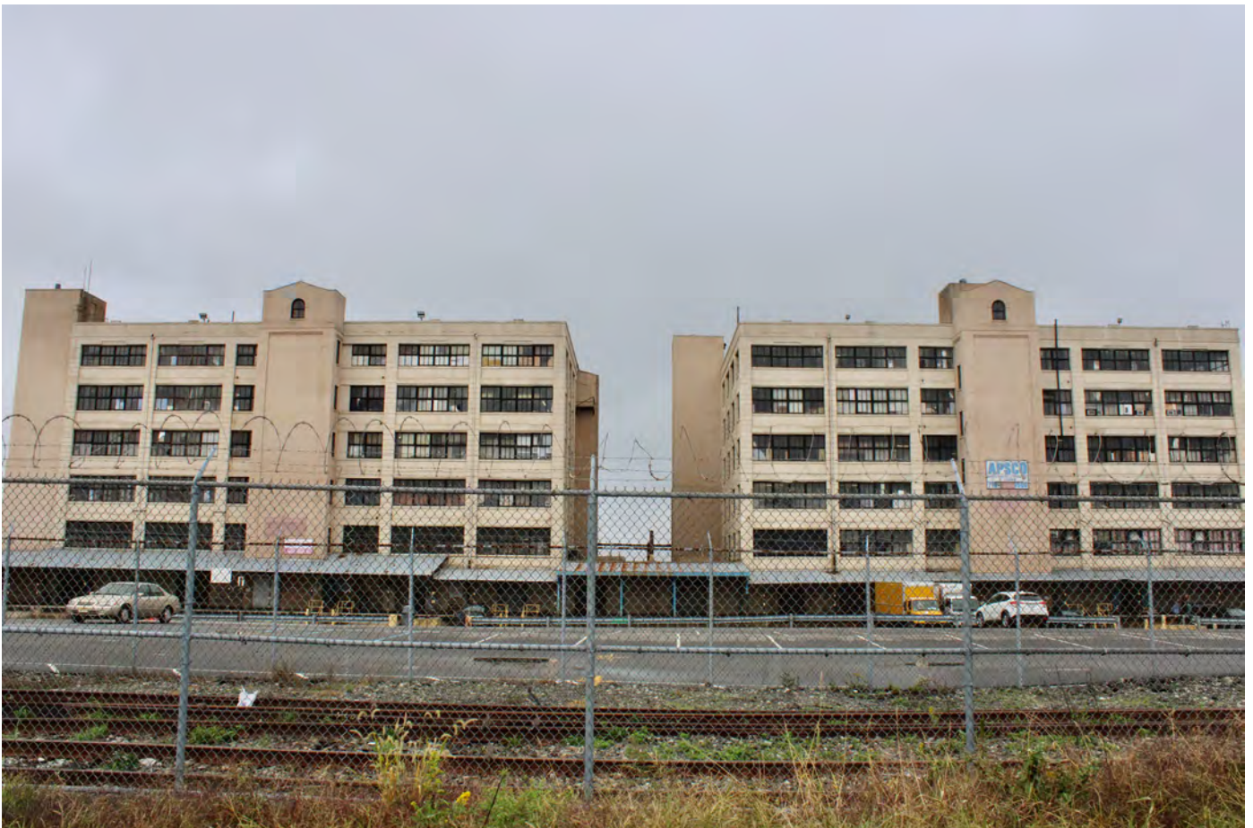
NY_Kings County_Bush Terminal_0038
