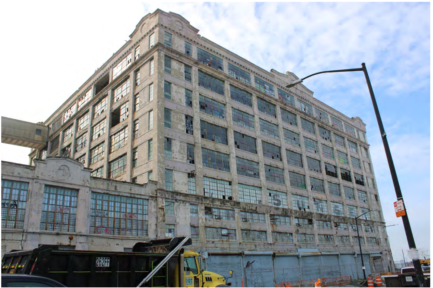
NY_Kings County_Bush Terminal_0059
