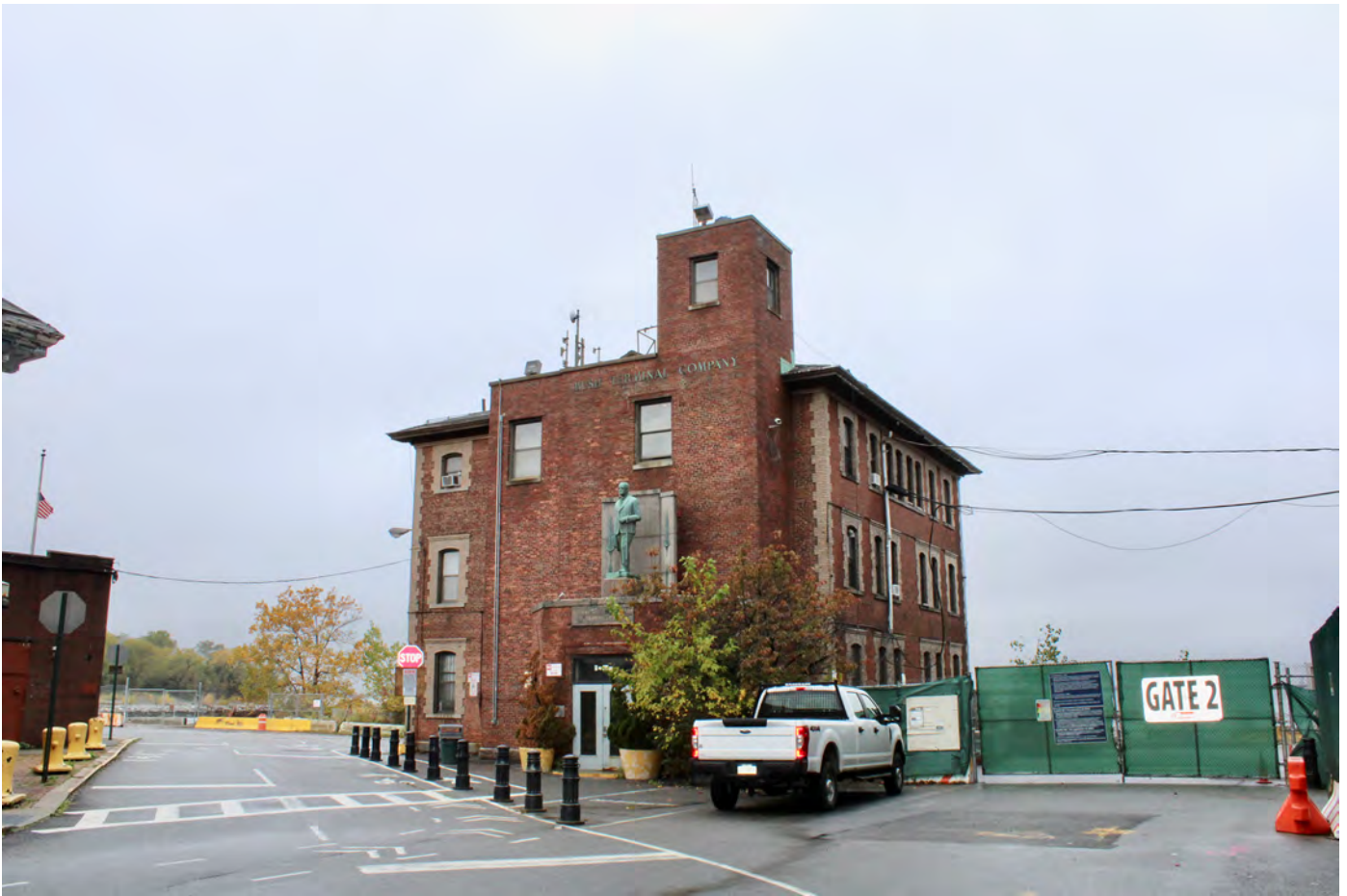
NY_Kings County_Bush Terminal_0043
