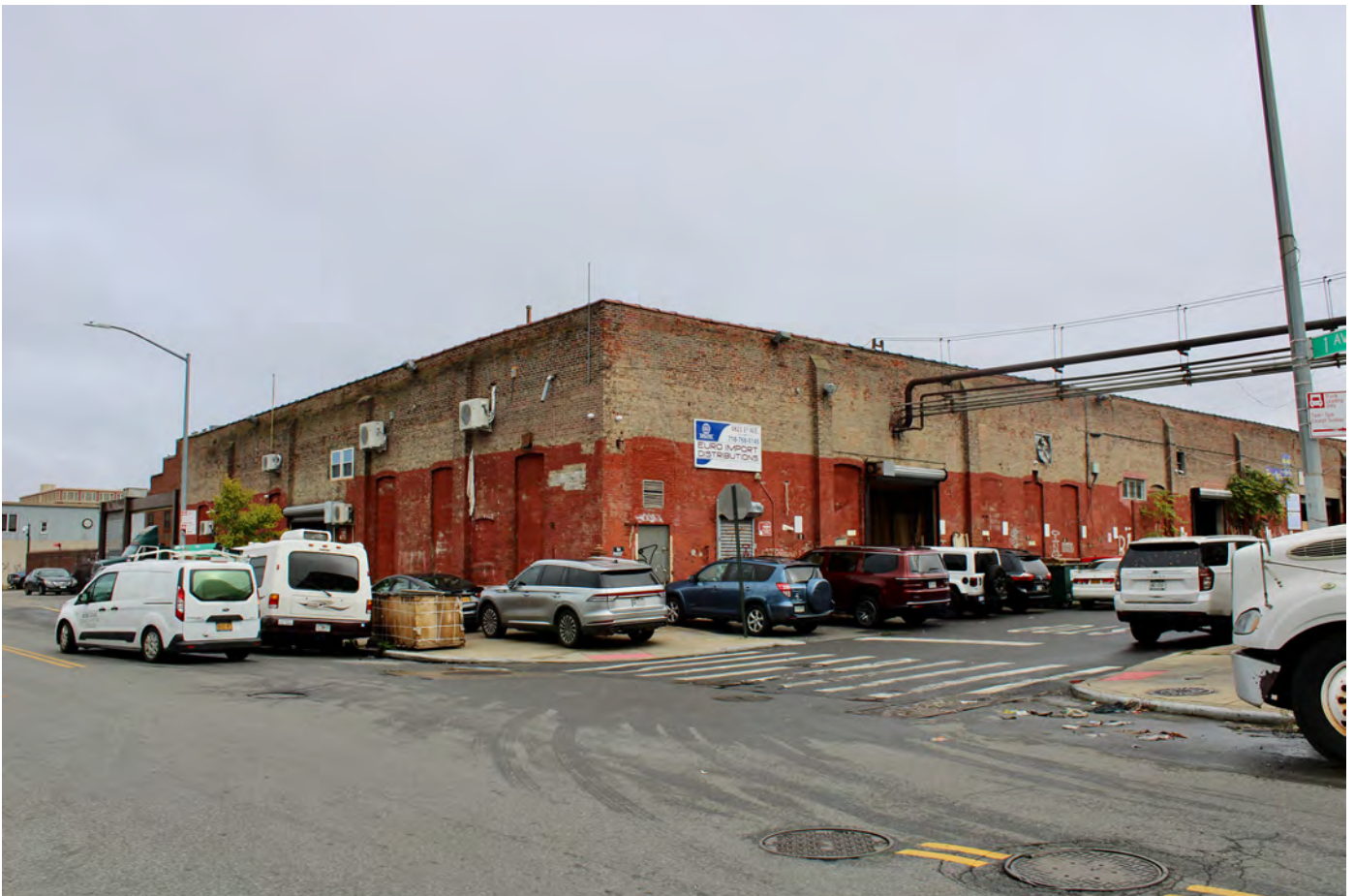
NY_Kings County_Bush Terminal_0004
