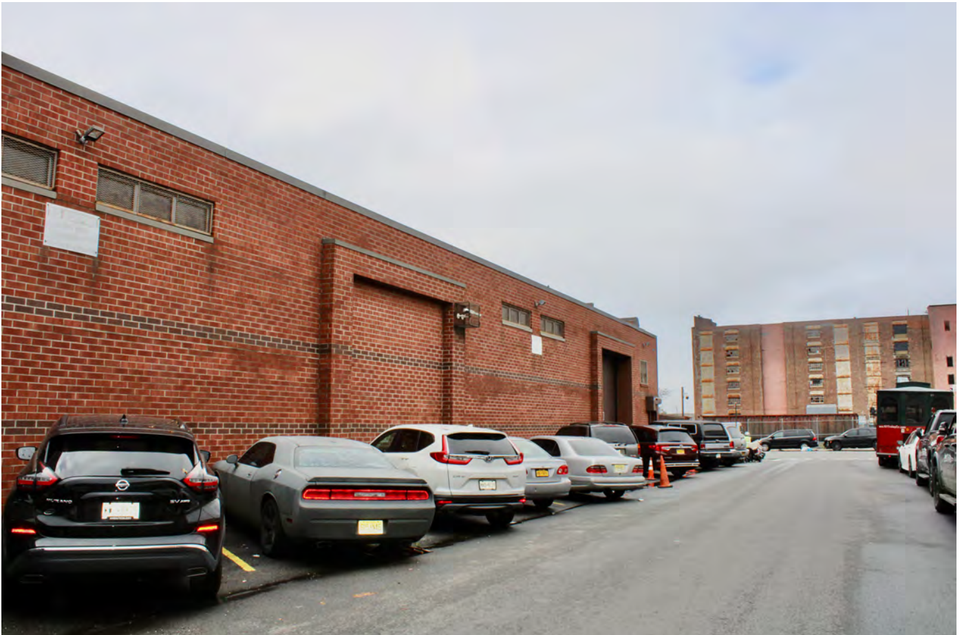
NY_Kings County_Bush Terminal_0018
