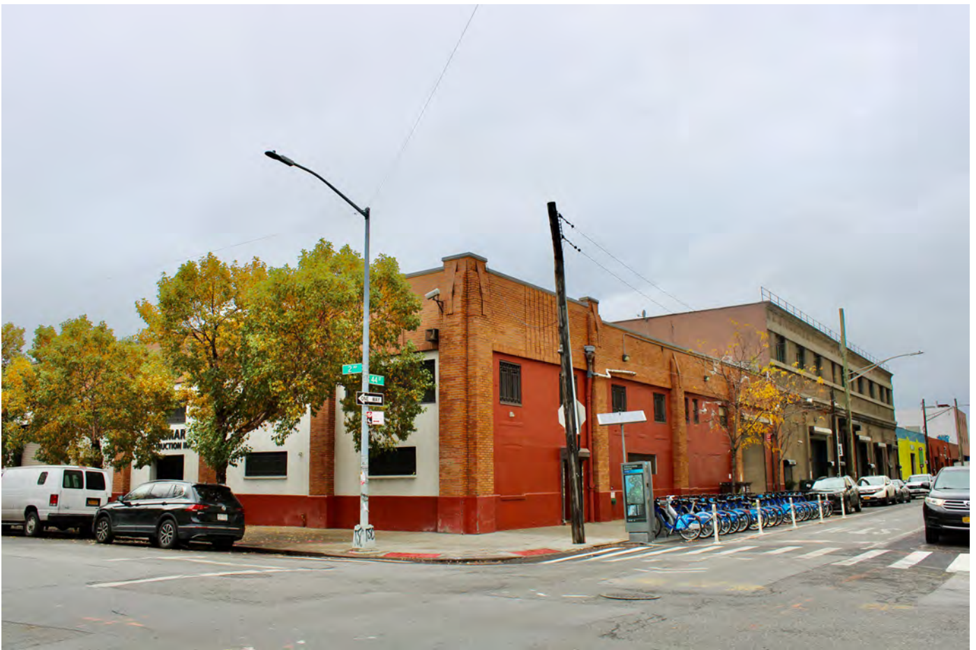
NY_Kings County_Bush Terminal_0027
