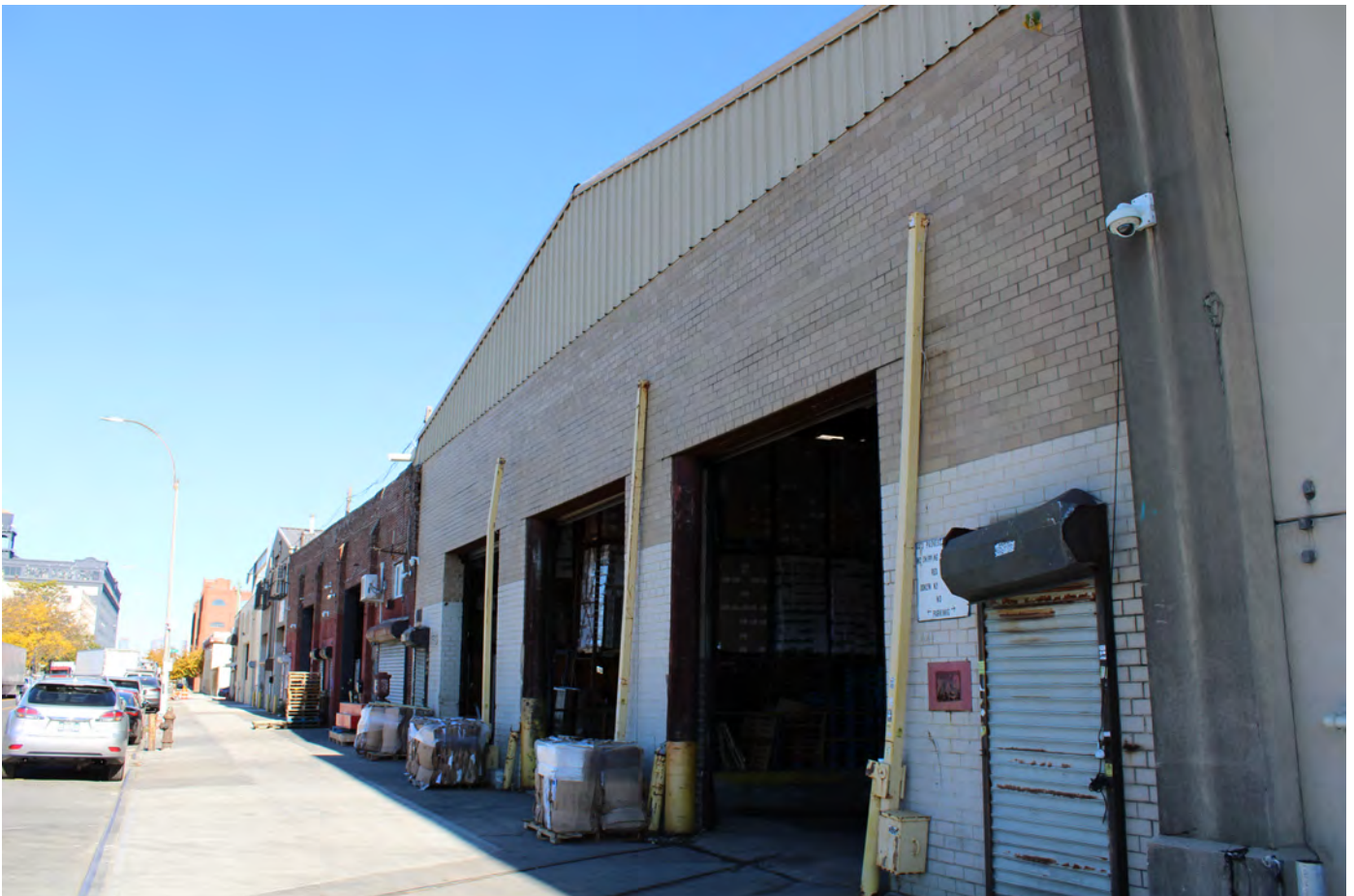
NY_Kings County_Bush Terminal_0034
