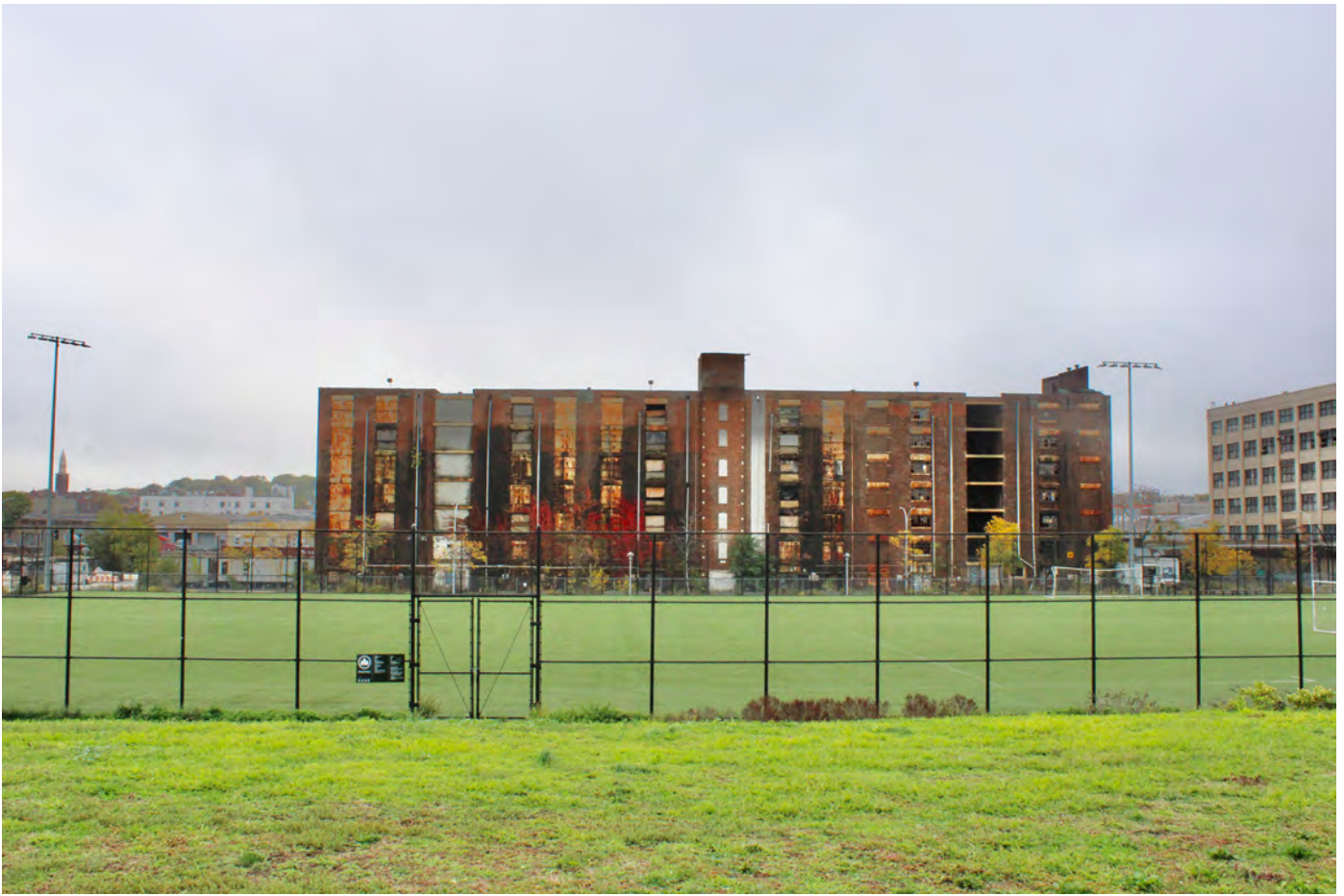
NY_Kings County_Bush Terminal_0041
