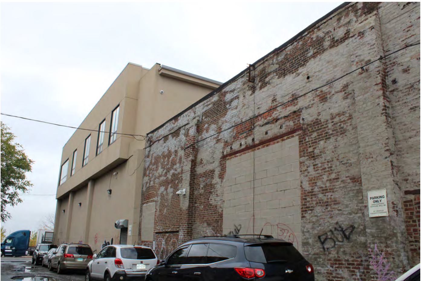
NY_Kings County_Bush Terminal_0031
