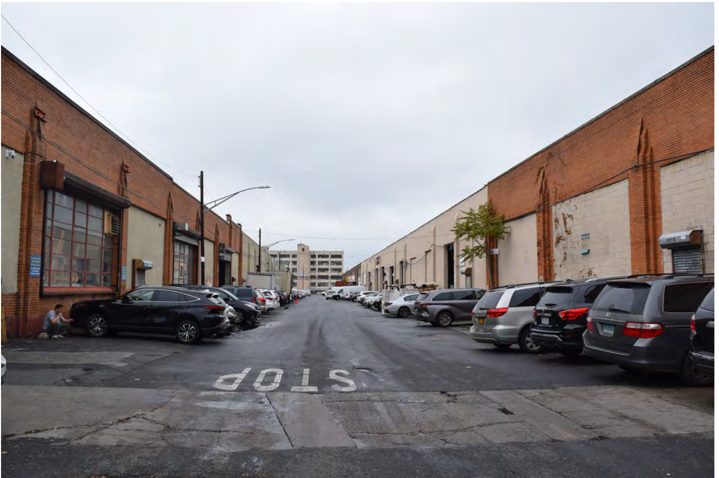
NY_Kings County_Bush Terminal_0009
