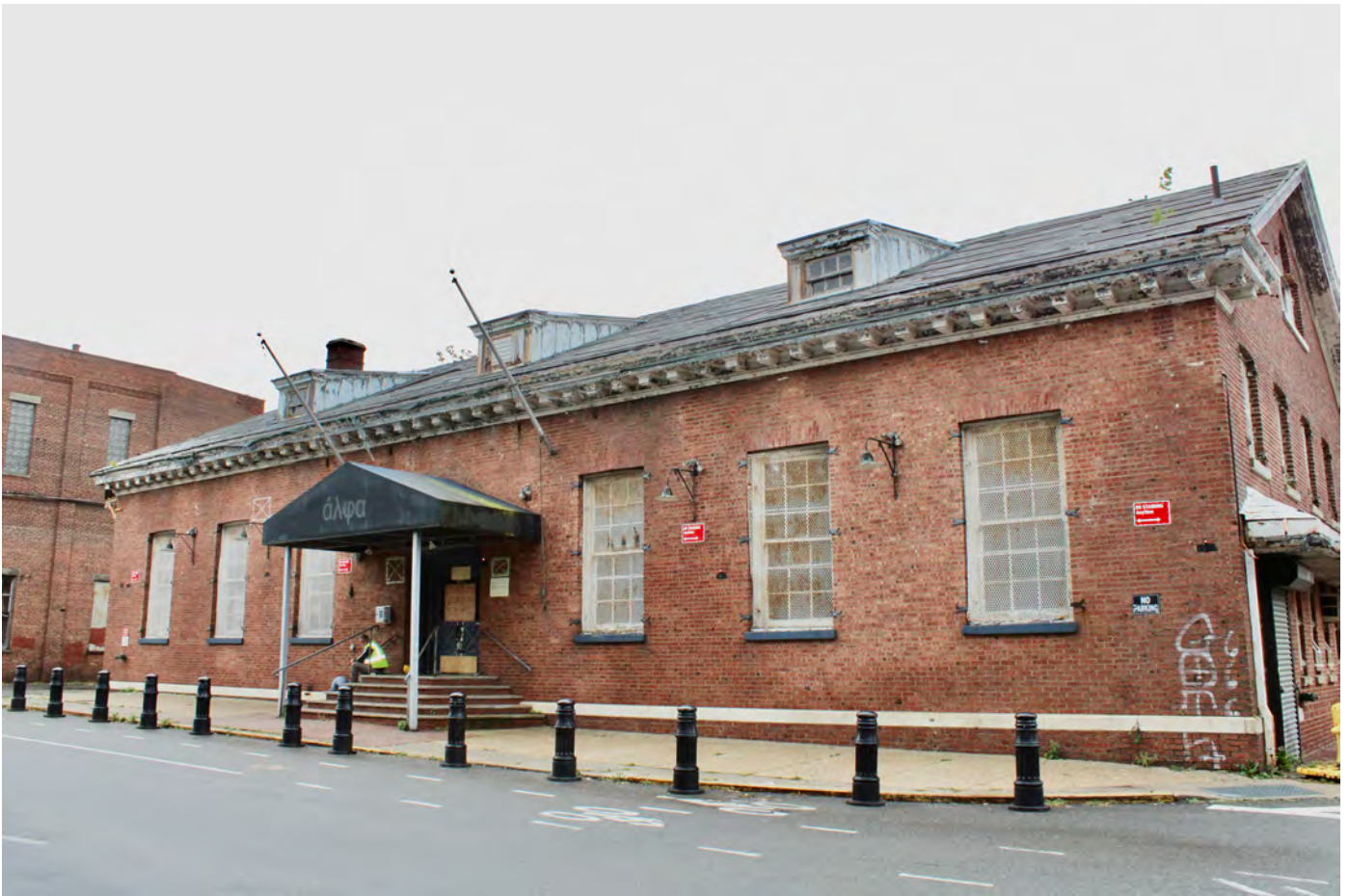
NY_Kings County_Bush Terminal_0045
