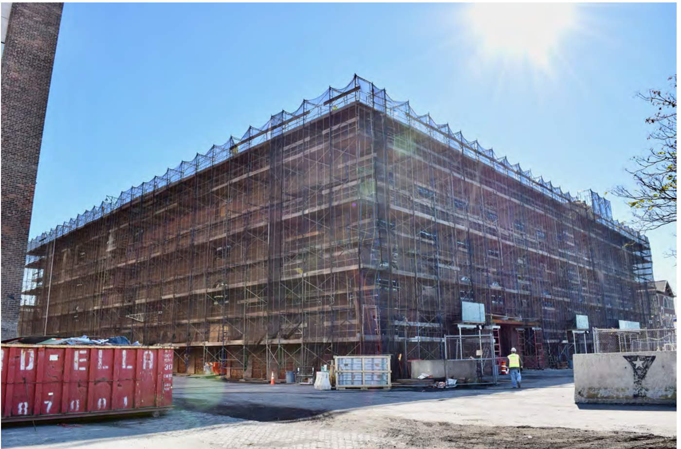
NY_Kings County_Bush Terminal_0052
