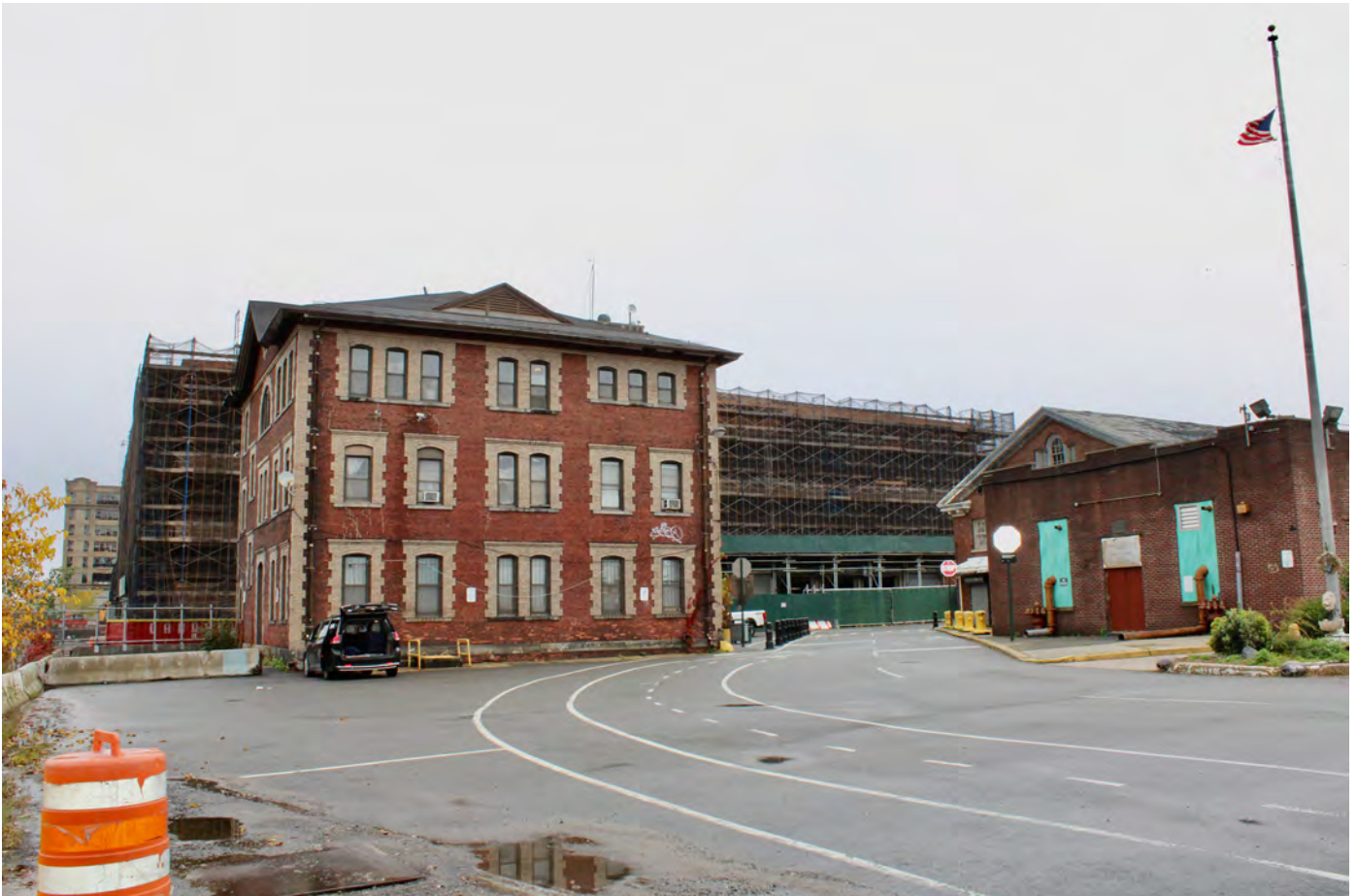
NY_Kings County_Bush Terminal_0042
