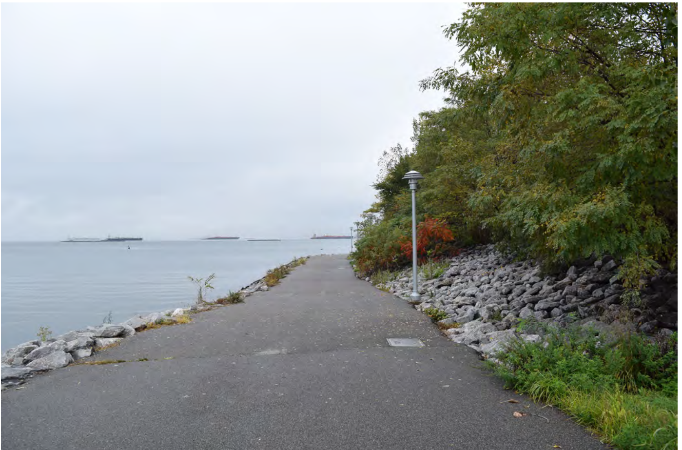
NY_Kings County_Bush Terminal_0046
