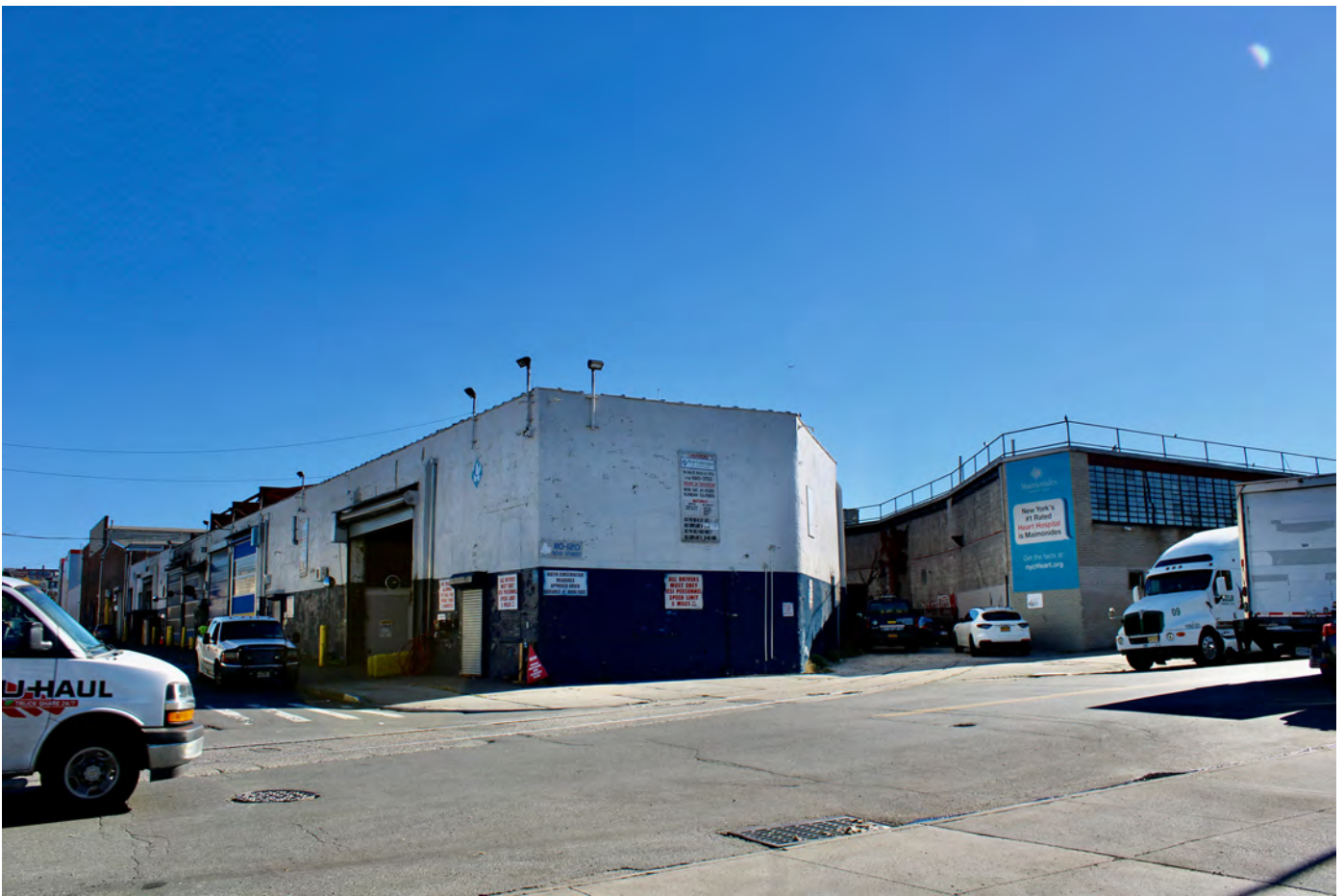
NY_Kings County_Bush Terminal_0001
