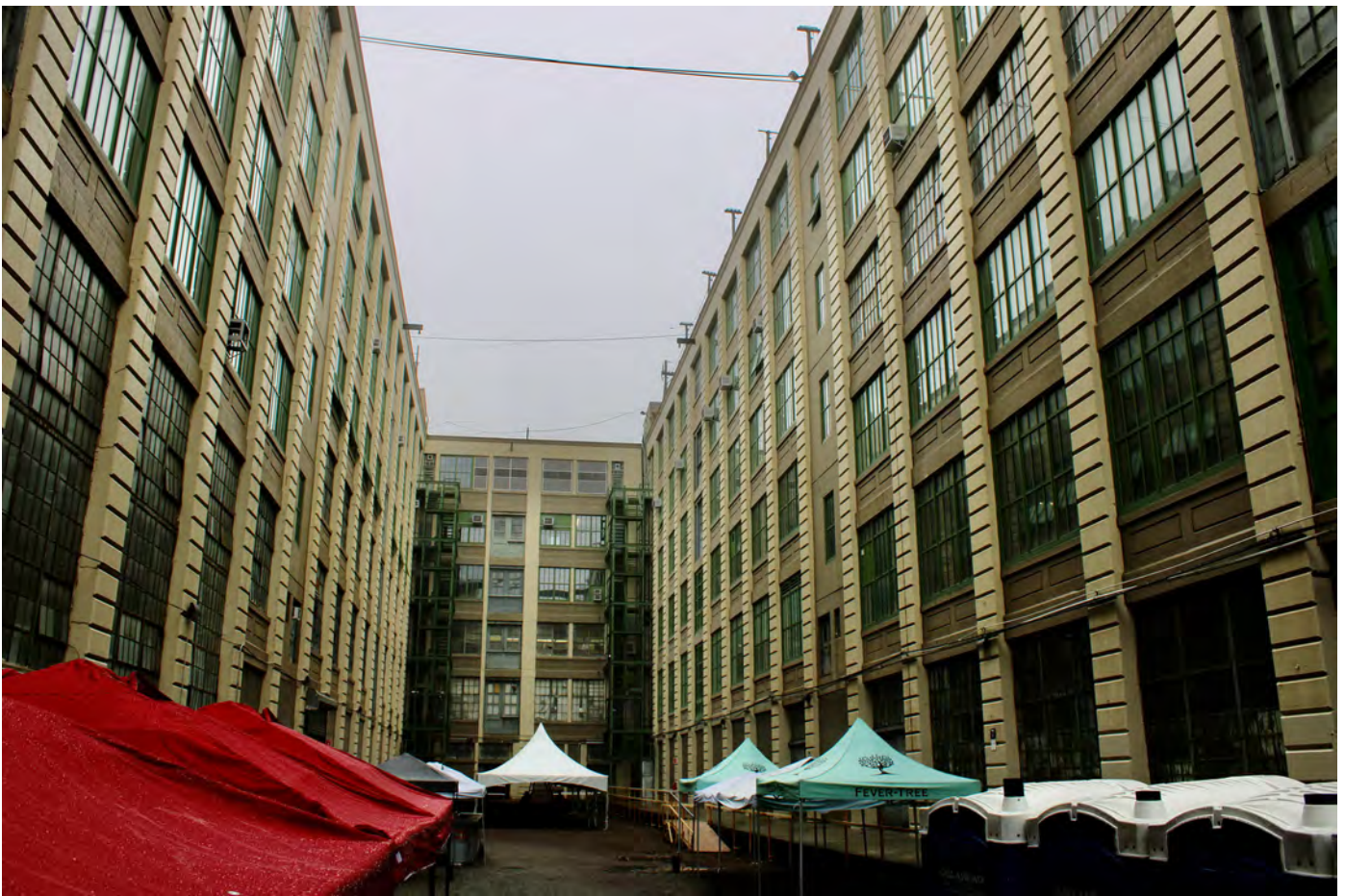
NY_Kings County_Bush Terminal_0077
