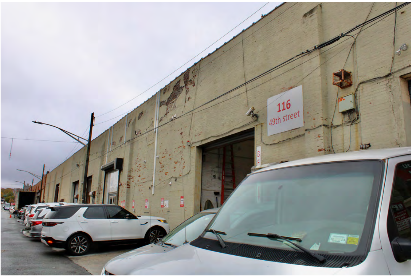
NY_Kings County_Bush Terminal_0007
