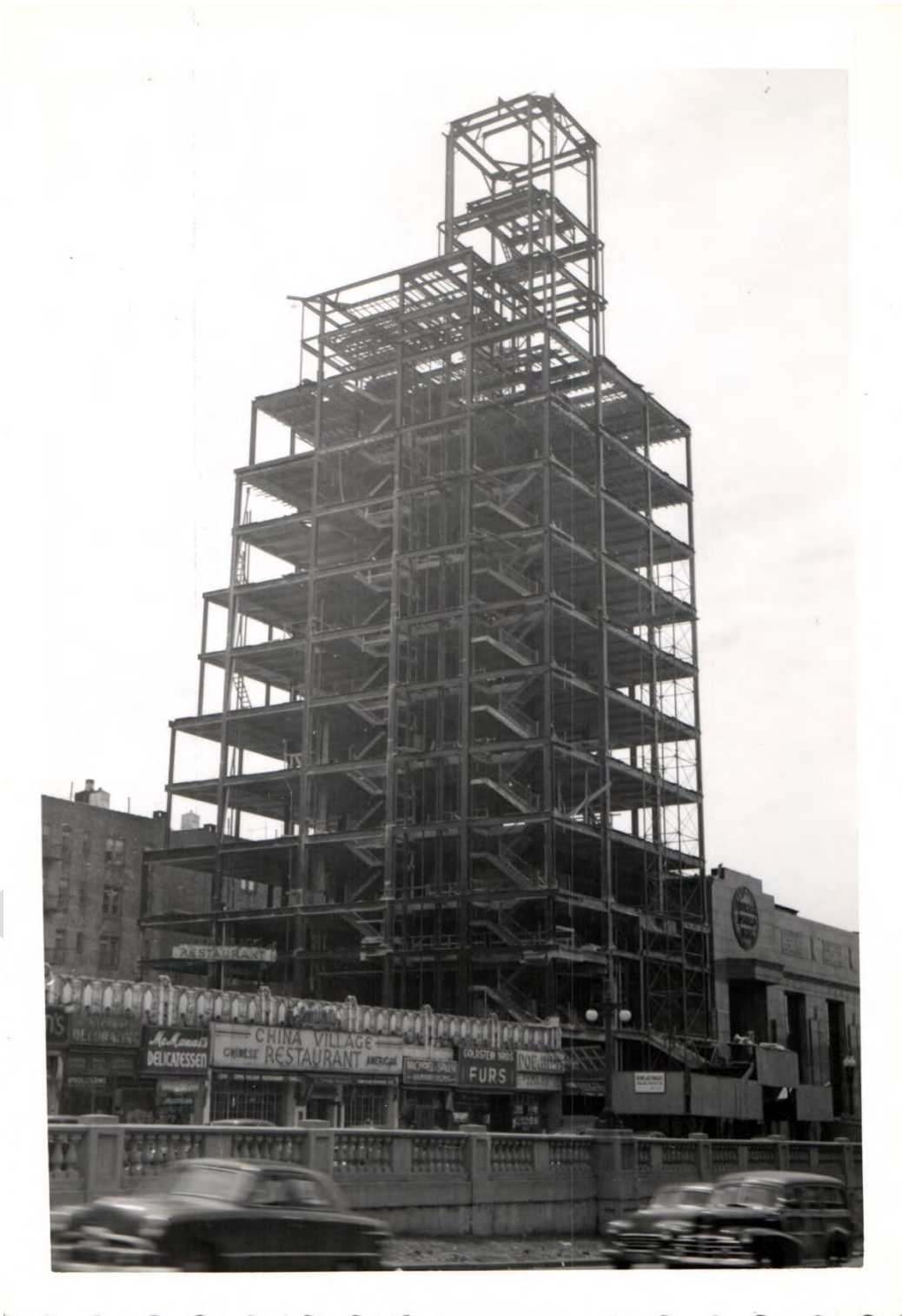
Figure 9: Ca. 1949 view of the office tower being constructed. (Bronx County Historical Society)
