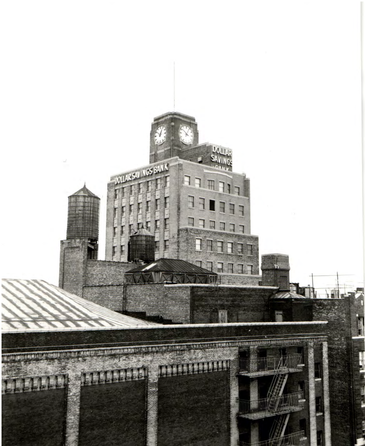
Figure 12: 1983 view of the building's east and south elevations. (Bronx County Historical Society)
