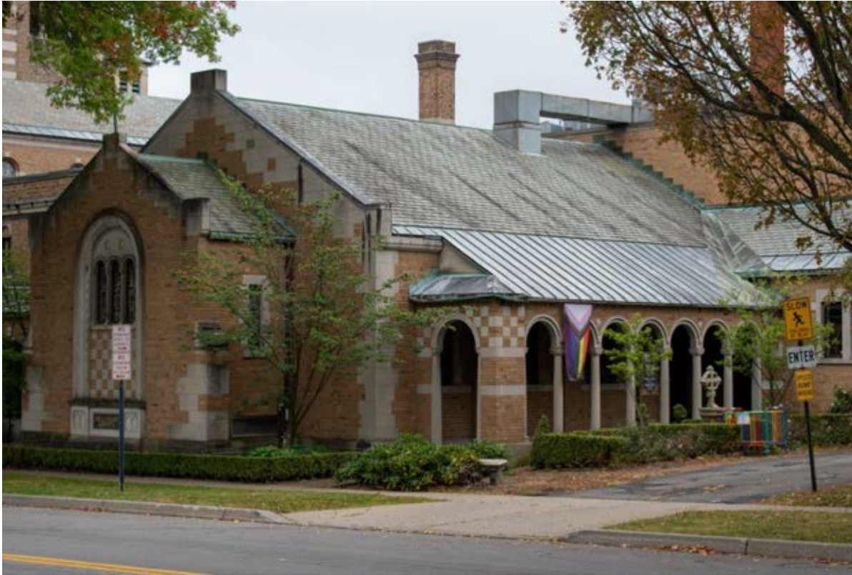
0013 of 0025: East elevation, First Presbyterian Church, view looking southwest.
