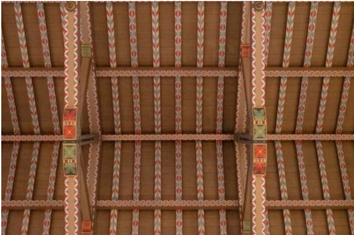
006 of 0025: Sanctuary ceiling, First Presbyterian Church, view looking up.
