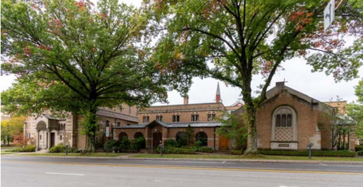
0001 of 0025: East elevation, First Presbyterian Church, view looking west.
