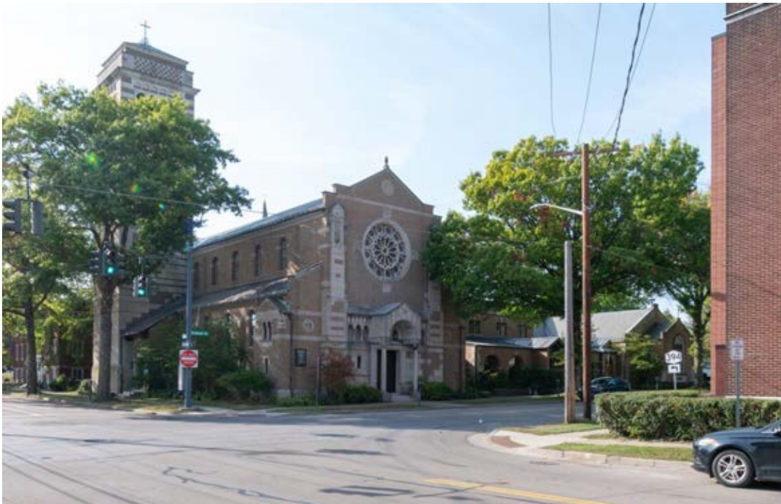
0002 of 0025: East elevation, First Presbyterian Church, view looking west.
