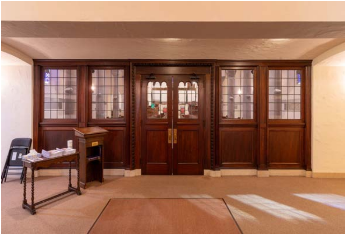
0008 of 0025: Narthex, First Presbyterian Church, view looking west.
