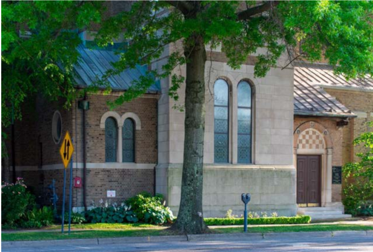
0003 of 0025: South elevation, First Presbyterian Church, view looking north.
