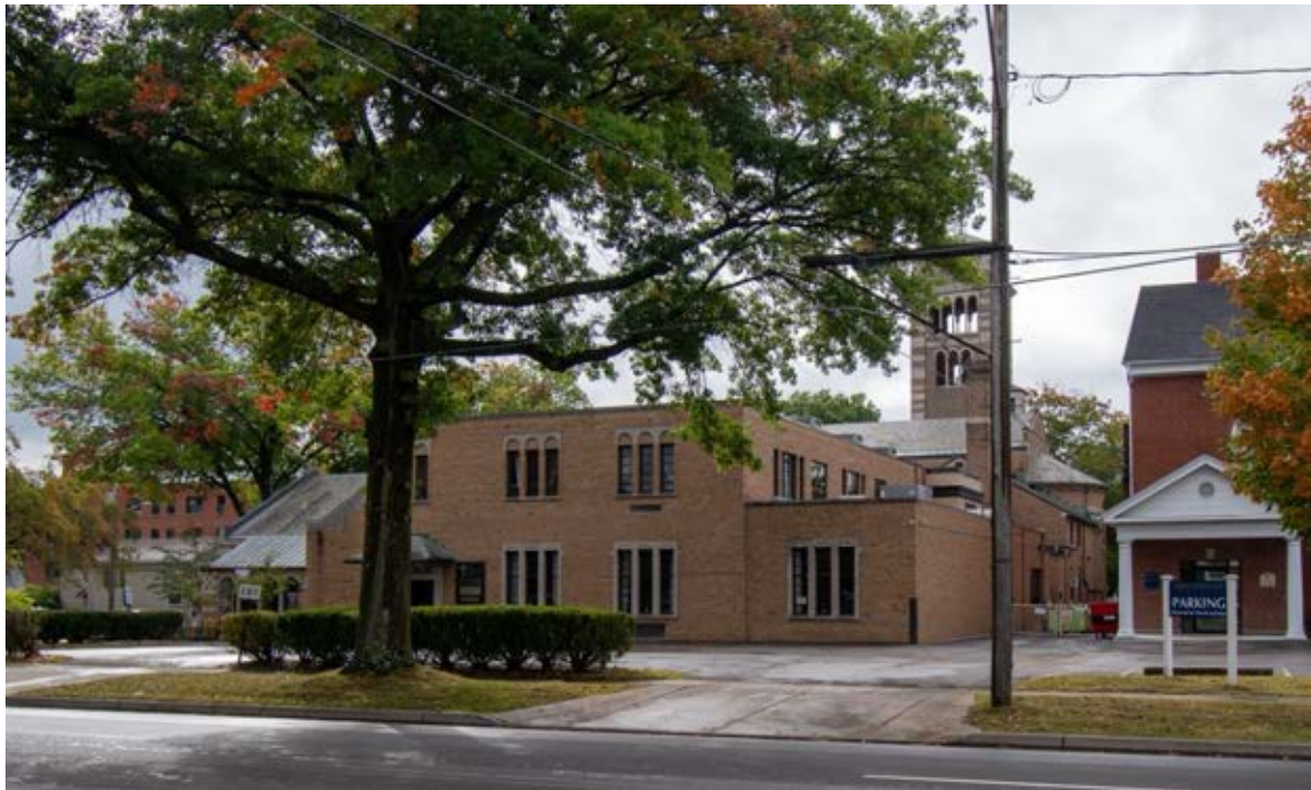
0014 of 0025: North elevation, First Presbyterian Church, view looking south.
