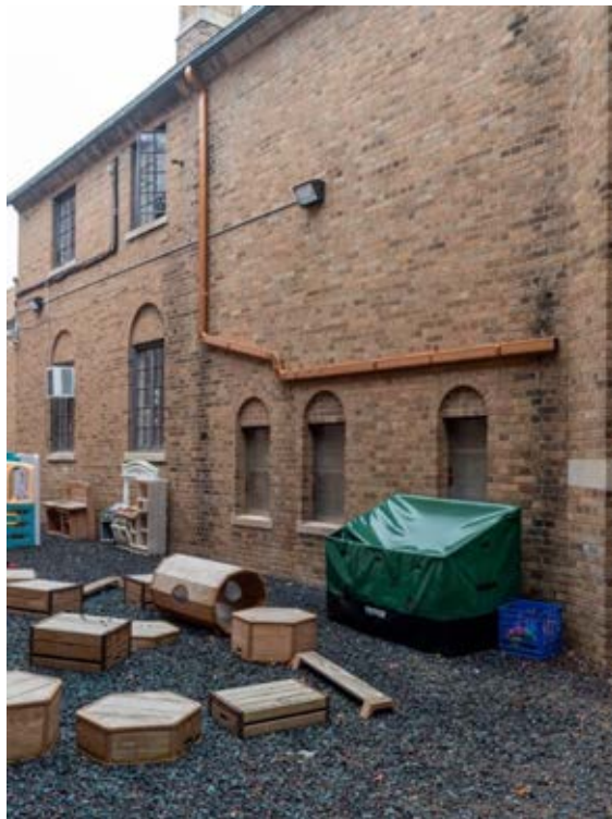
0004 of 0025: West elevation, First Presbyterian Church, view looking east.
