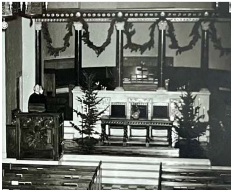
Figure 6: Historic photograph of the chancel showing the original linoleum floor tiles and wooden platform under the communion table and chairs
