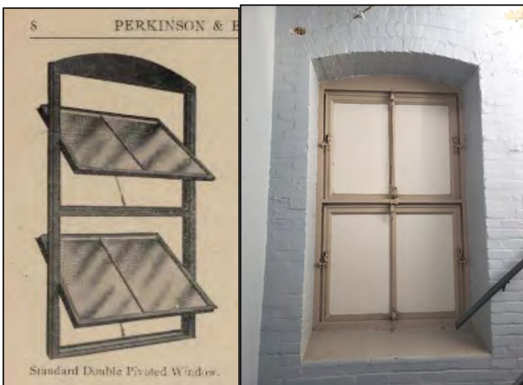
"Standard Double Pivoted Window" from the 1906 Perkins & Brown Fireproof Window catalog and its corresponding extant example at GE Building 32.
