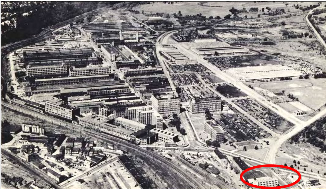
Photo from page 2 of the 1949 Schenectady Works Welcomes You! souvenir booklet published by General Electric. The booklet stated that there were 240 buildings at this time. Note G.E. Building 32 circled in lower right corner, showing the building already painted. https://www.schenectadyhistory.org/ge/swwu/index.html .
