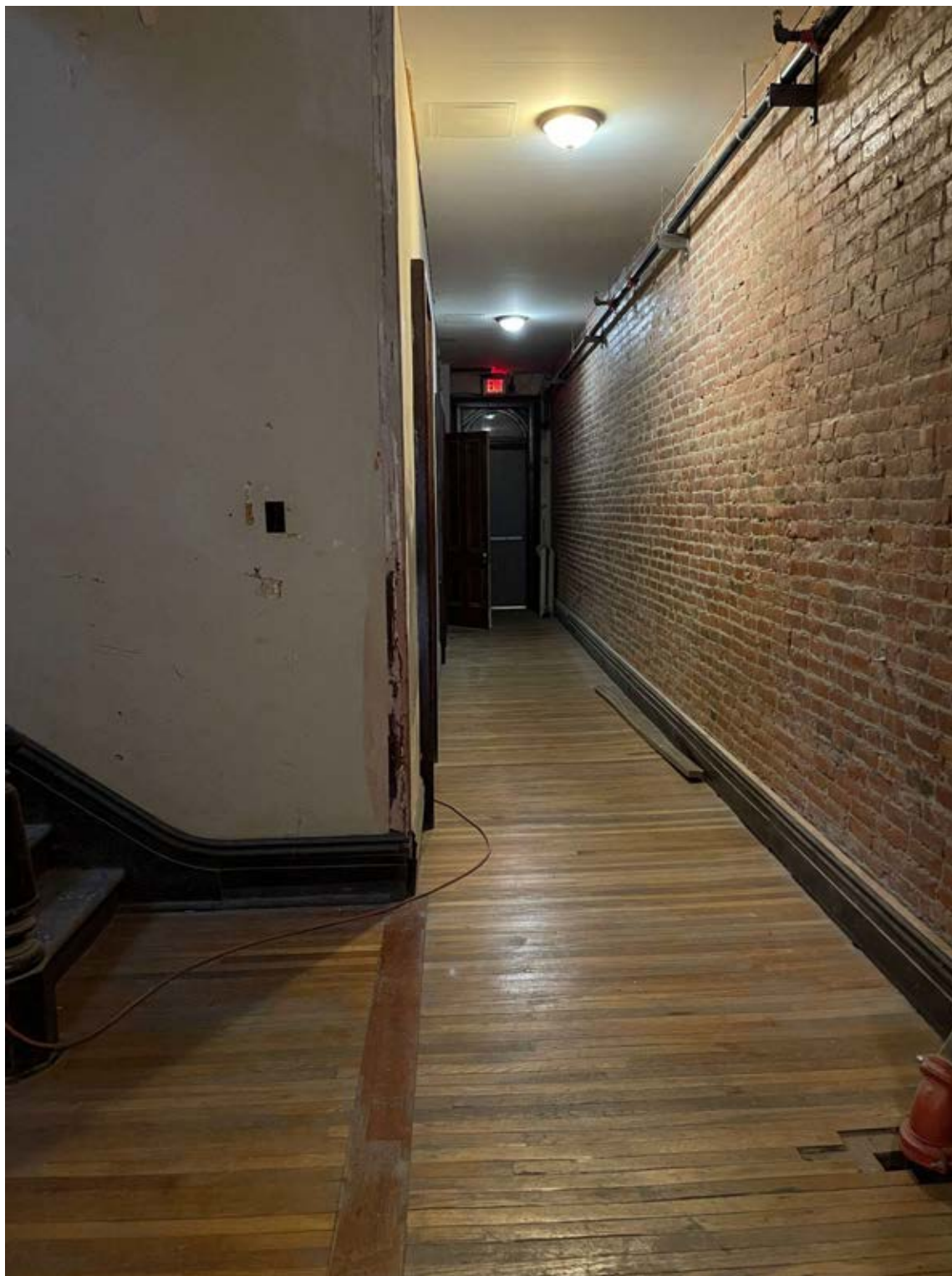
Figure 2.7. Second floor hallway of 141 East State Street (141 The Commons), looking south. Photo by Jeff Iovannone, April 18, 2023.
