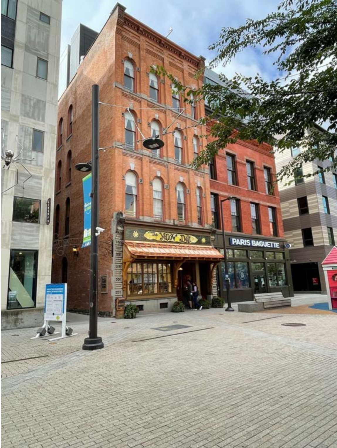
Figure 2.1. North elevation (front) view of 141-143 East State Street, looking south. Photo by Jeff Iovannone, May 15, 2023.
