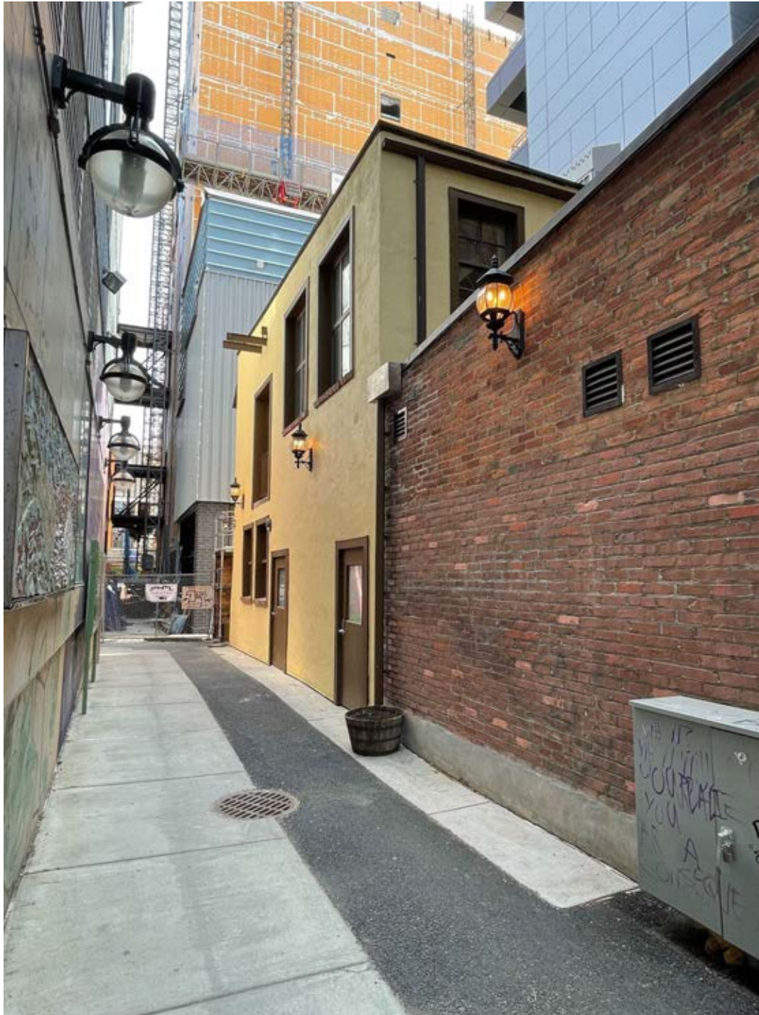
Figure 2.4. East elevation view of 143 East State Street depicting the two-story addition on the south, rear, elevation, looking southwest. Photo by Jeff Iovannone, May 15, 2023.
