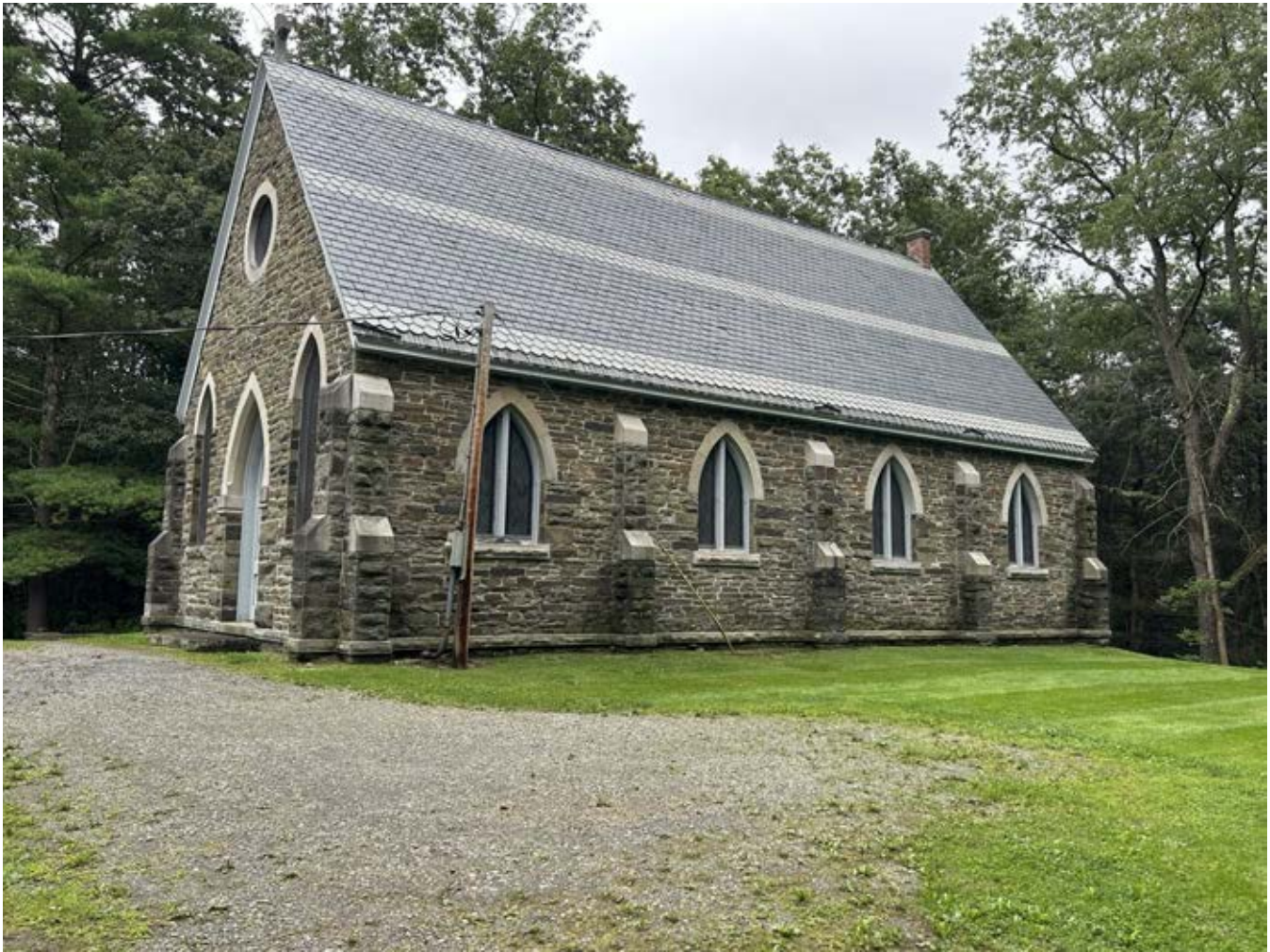
0005 Exterior View West
