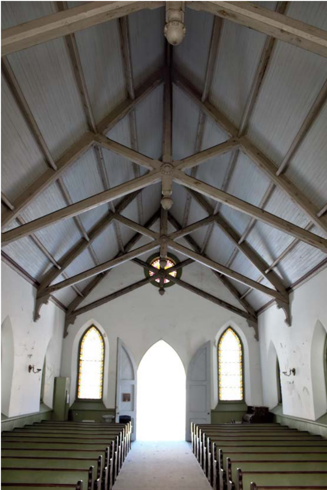
0011 Interior View Northwest Toward Entrance
