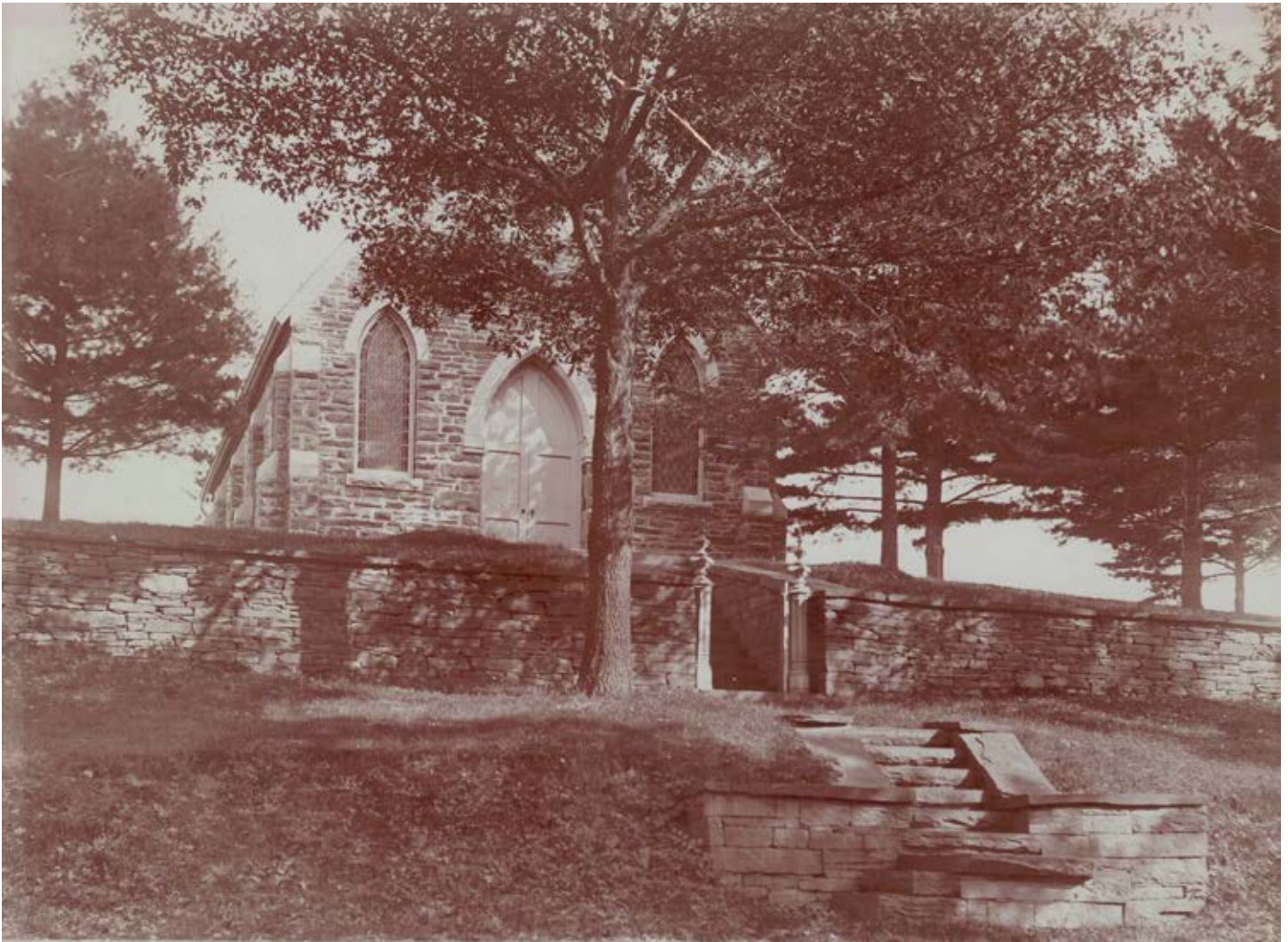
Figure 3: Photograph 1949, View South
