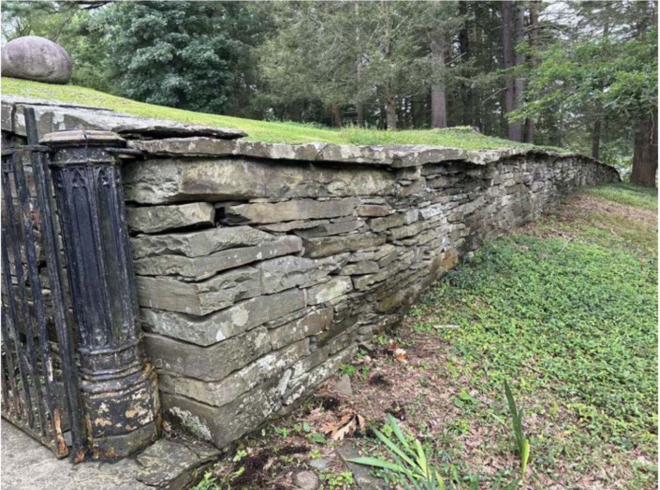
0018 West Wall Along SR 228
