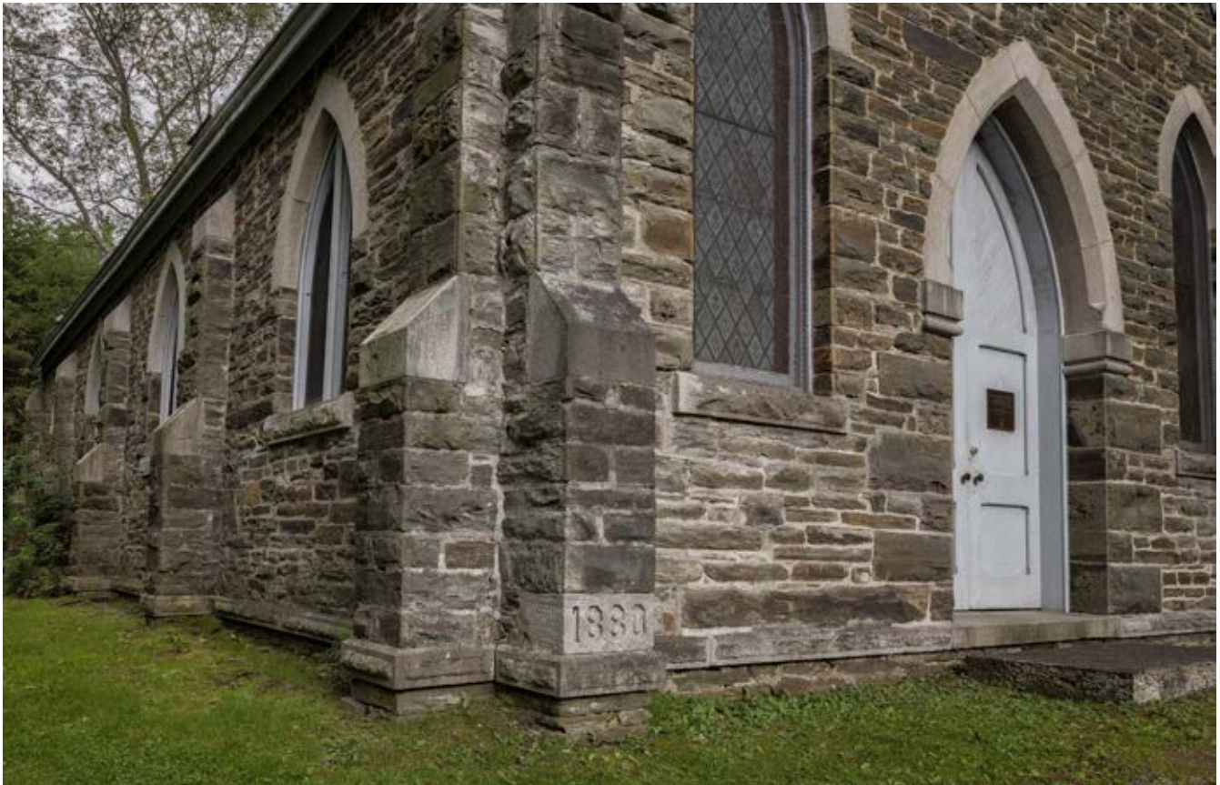
0006 Exterior View South Showing Date
