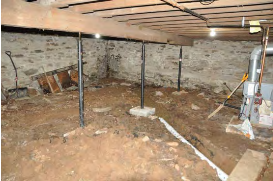
0013 of 0028: Basement with fieldstone foundation and dirt floor, looking southeast.
