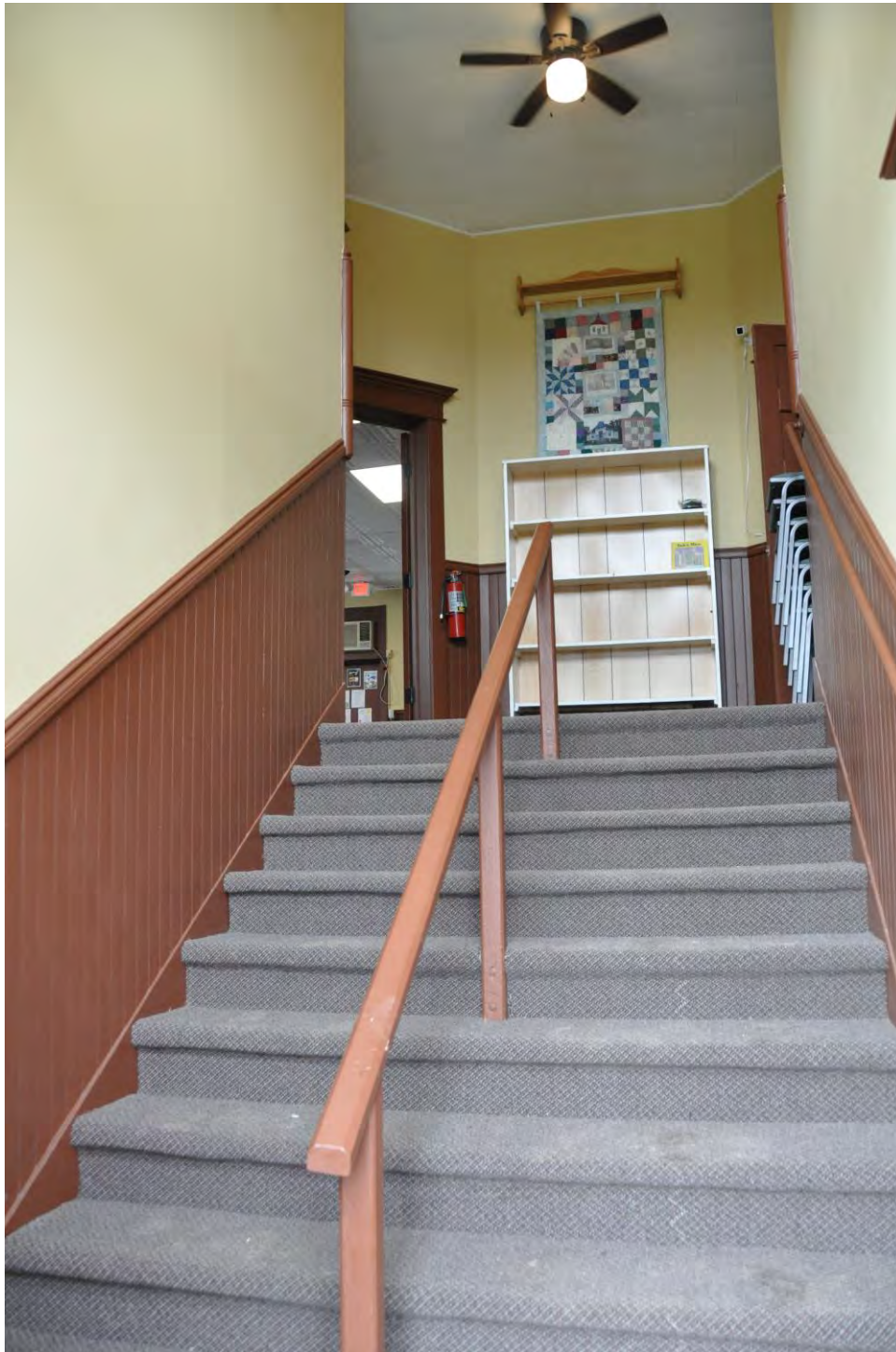
0007 of 0028: Front foyer with stairs to first floor, looking south.
