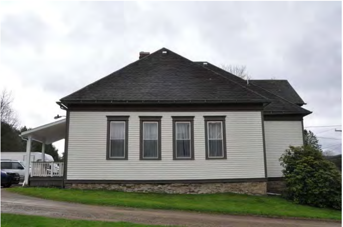
0006 of 0028: East elevation, looking west.
