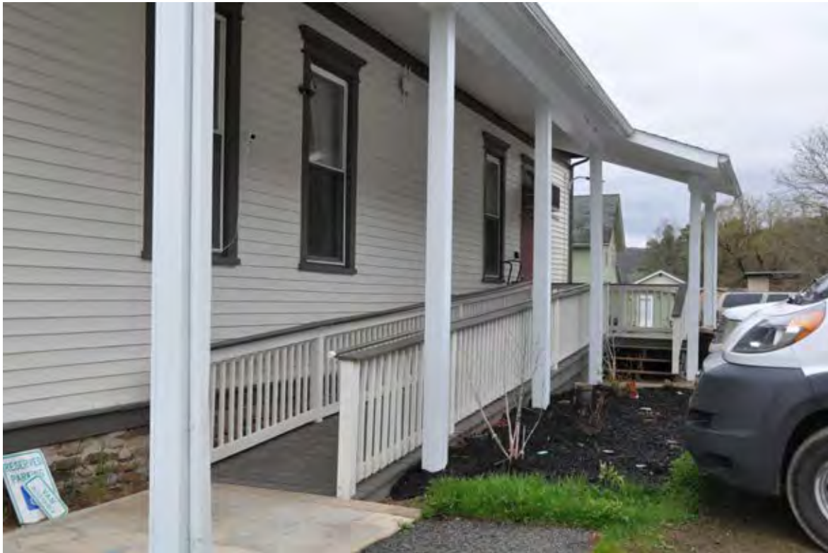
0004 of 0028: Rear/south elevation with ADA compliant ramp and non-historic porch, looking east.
