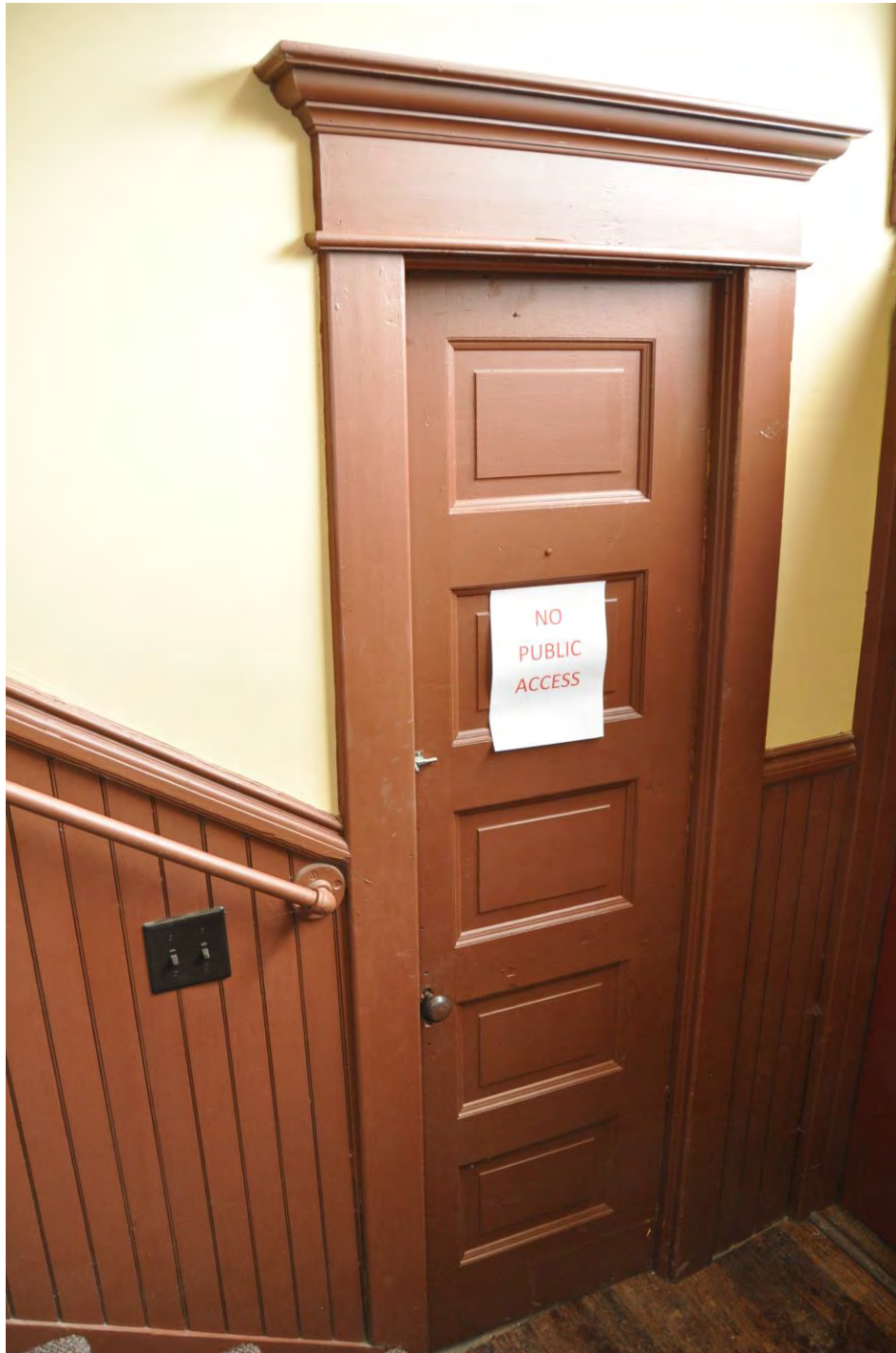
0008 of 0028: Original door to basement and attic access, looking northwest.
