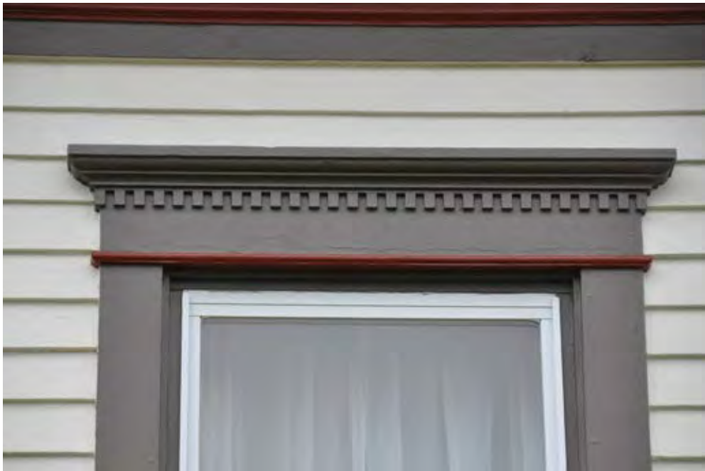
0002 of 0028: Detail of dentil trim on lintel, looking west.
