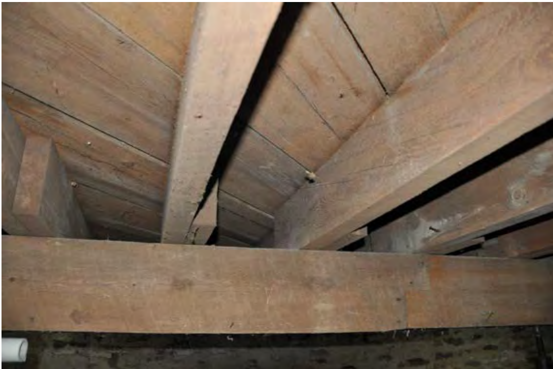
0014 of 0028: Exposed wood floor joists in basement, looking up and east.
