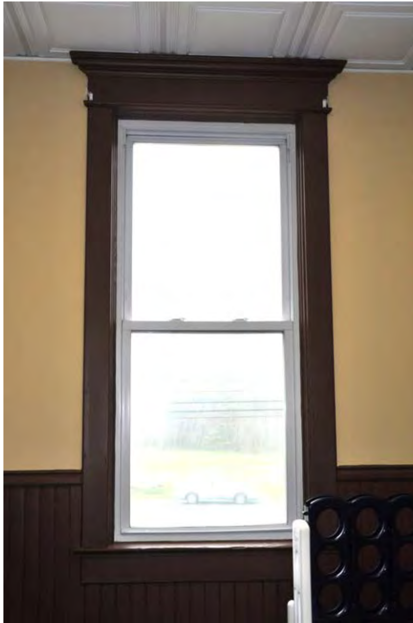
0026 of 0028: Detail of interior window trim, from children's room looking north.
