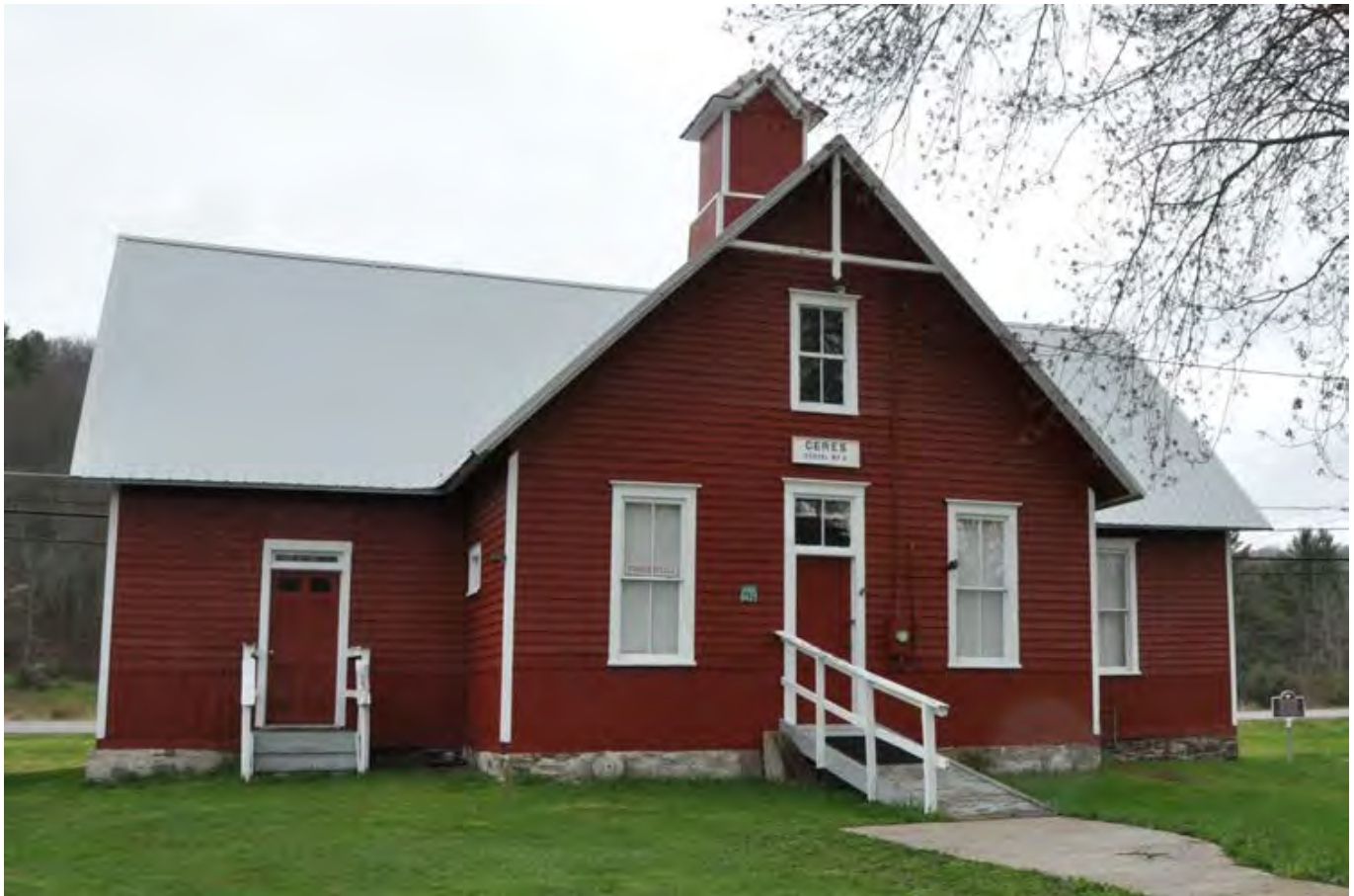
0028 of 0028: Ceres Schoolhouse/Genesee District No. 6 School in Ceres, New York serves as a museum today and was listed in the National Register in 2010, looking north.
