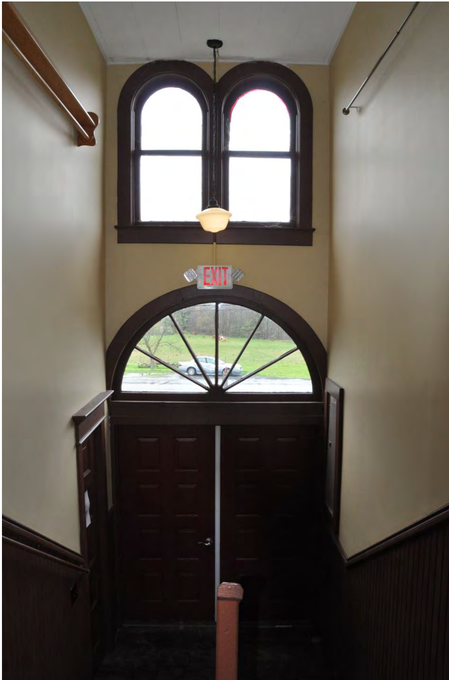
0009 of 0028: Front doors, fanlight and round arched windows, original school light, looking north.
