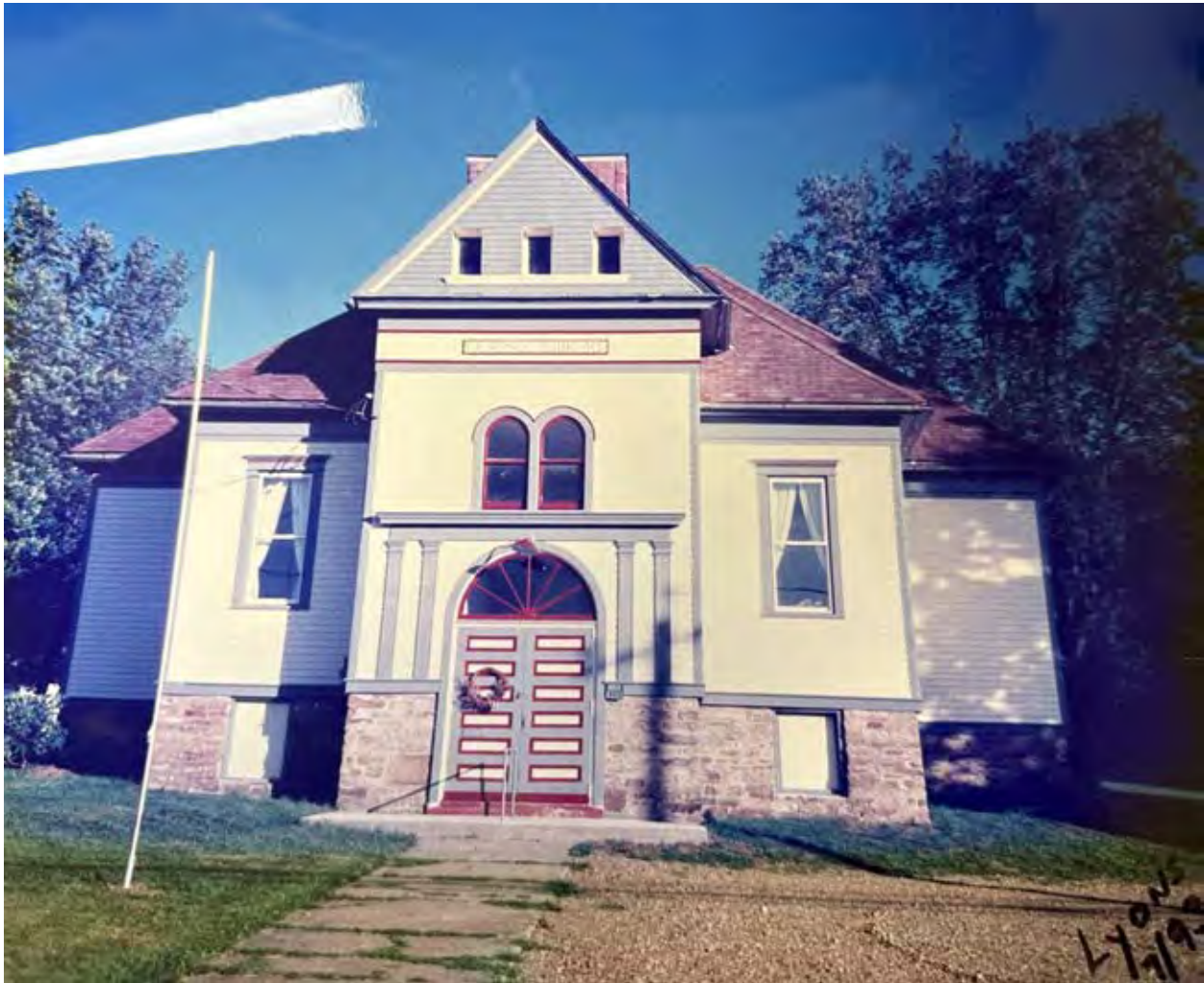
Figure 31: Genesee Library, ca. 1993. Note the one-over-one replacement windows. Courtesy of the Genesee Library. Bolivar-Richburg-Allentown-Genesee Historical Preservation Society.
