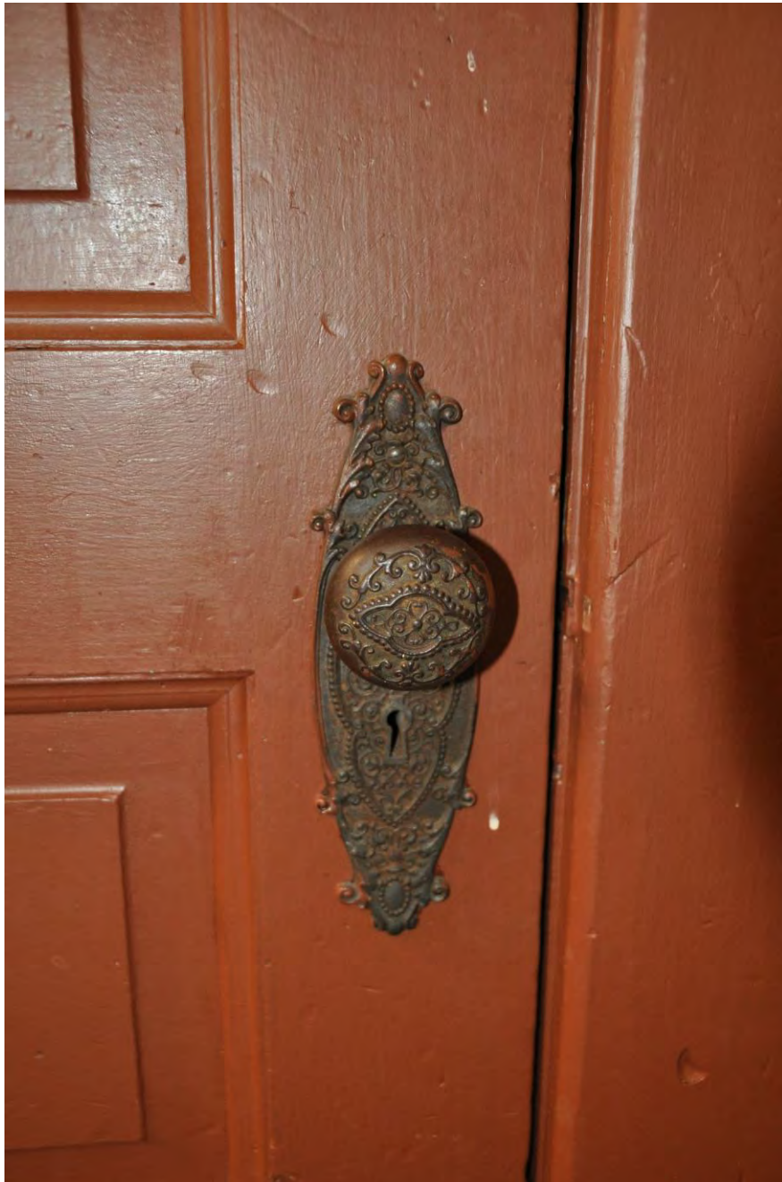
0011 of 0028: Original hardware on original door, looking east.
