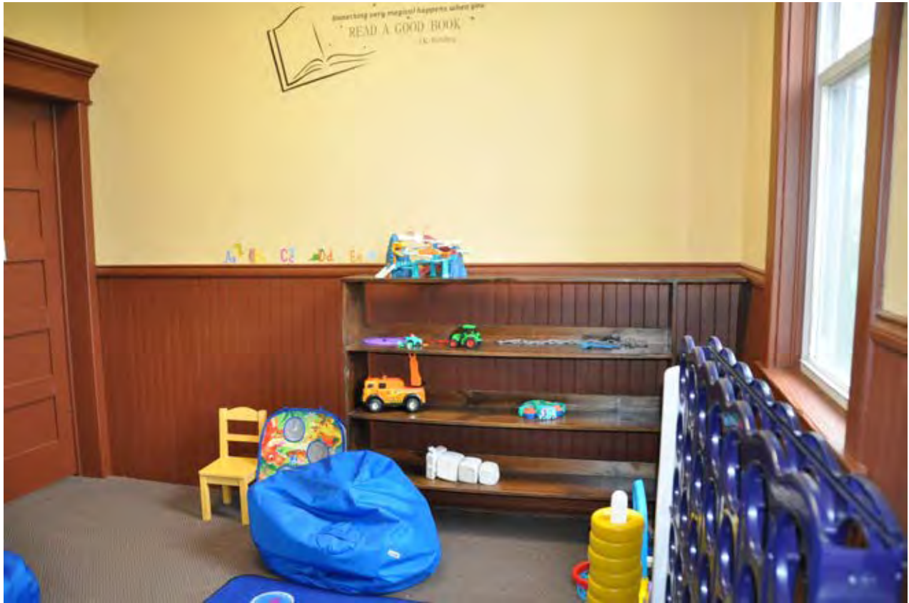
0025 of 0028: Original wainscoting can be found throughout the building, from children's room looking west.
