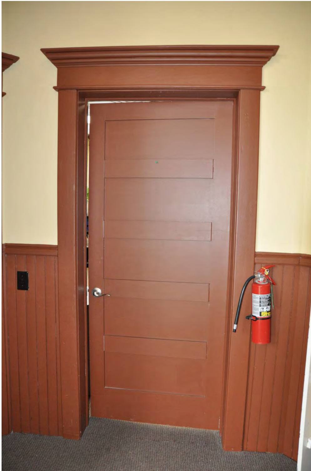
0012 of 0028: New classroom door and trim, looking south.
