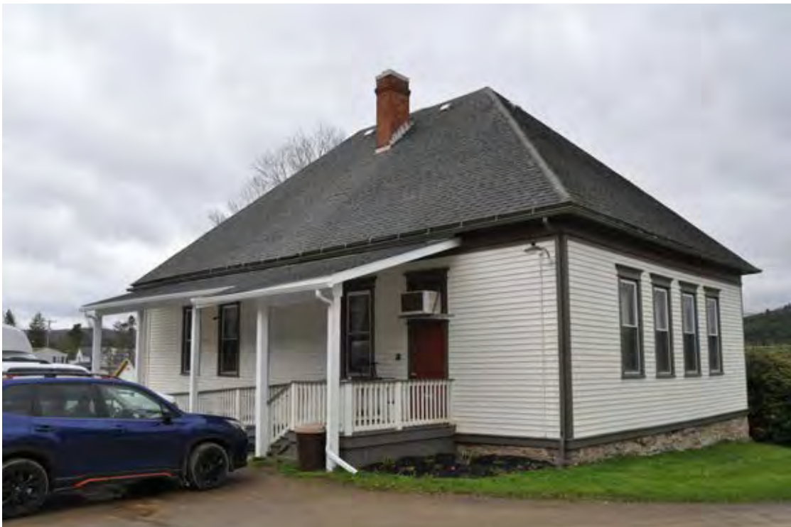
0003 of 0028: Rear/south elevation and east elevation, view looking northwest.
