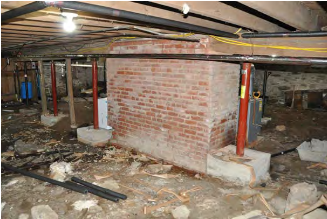
0015 of 0028: Brick chimney and steel and wood posts, looking northeast.
