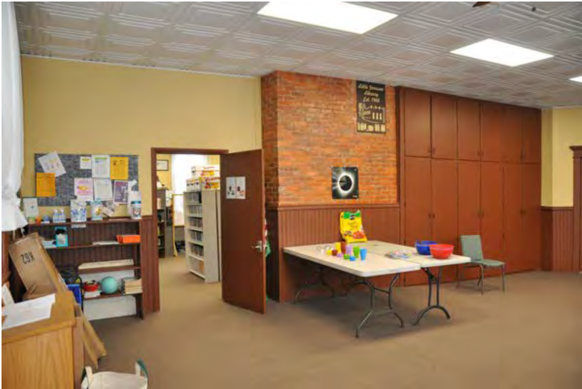
0019 of 0028: East classroom/community room with entrance to west classroom/library room, exposed brick wall from chimney and built-in cabinets, looking west.
