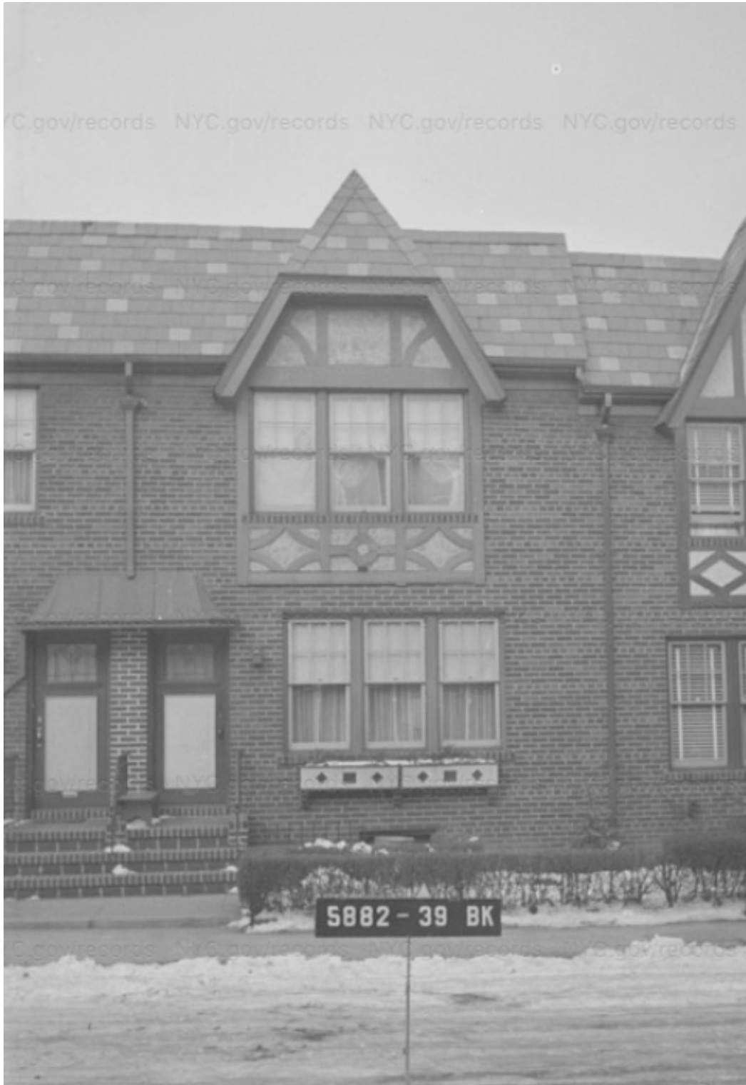
Figure 12: Ca. 1940 view of 7016 Louise Terrace, a typical example of house Type C features decorative half-timbering with orthogonal and curved wood members and a jerkinhead gable (NYC Municipal Archives).
