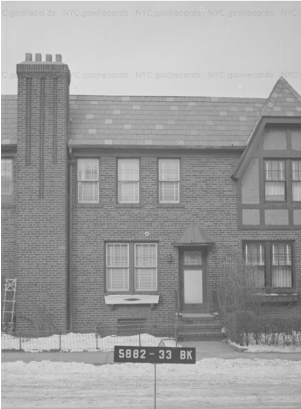
Figure 11: Ca. 1940 view of 7004 Louise Terrace, a typical example of house Type B. Type B is the simplest design type and features a pitched slate roof and shares a tall projecting brick chimney with its neighbor (NYC Municipal Archives).
