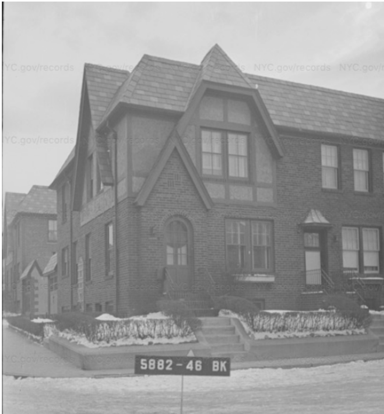
Figure 10: Ca. 1940 view of 7001 Louise Terrace, a typical example of house Type A. Type A is located at the corners and has two street-facing facades and features an asymmetrically placed, round-arched entrance, multiple gables, and decorative half-timbering with stucco (NYC Municipal Archives).
