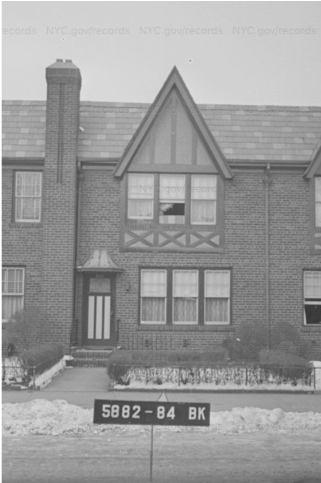
Figure 13: Ca. 1940 view of 7010 Colonial Road, a typical example of house Type D. Type D features decorative half-timbering with orthogonal wood members and a steep pointed gable. The north Type D house shares a tall projecting brick chimney with its neighbor (NYC Municipal Archives).
