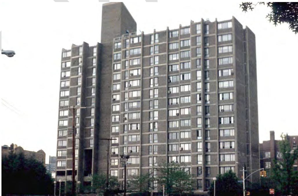
Figure 15: 1973 photo taken shortly after completion. (Photo by Lauren Soth via the Paul Rudolph Institute: https://www.paulrudolph.institute/196711-middletown-plaza )
