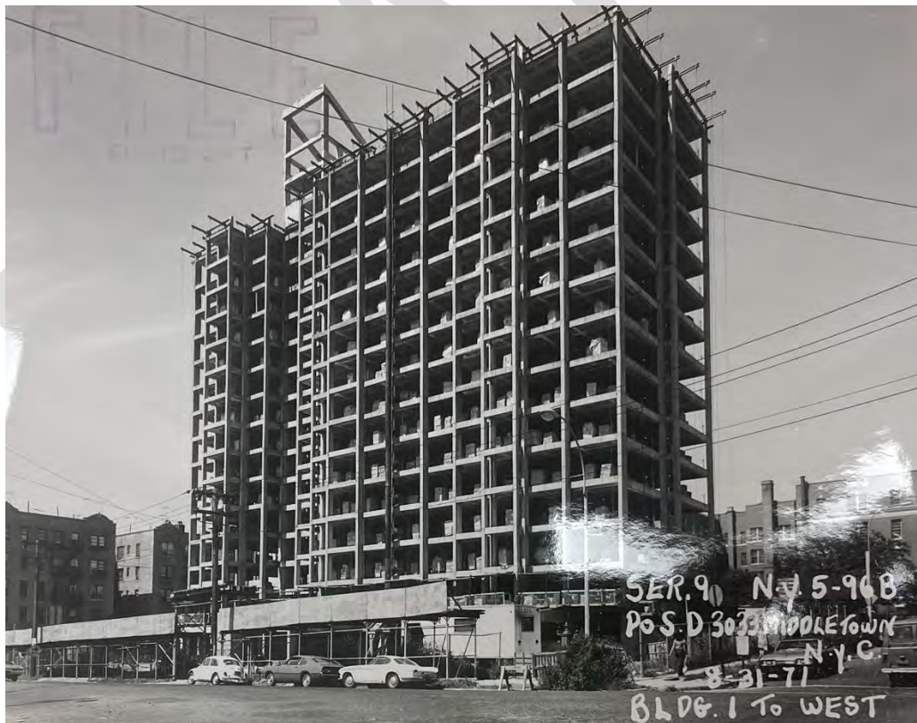
Figure 13: 1971 view of Middletown Plaza while under construction. (NYCHA)
