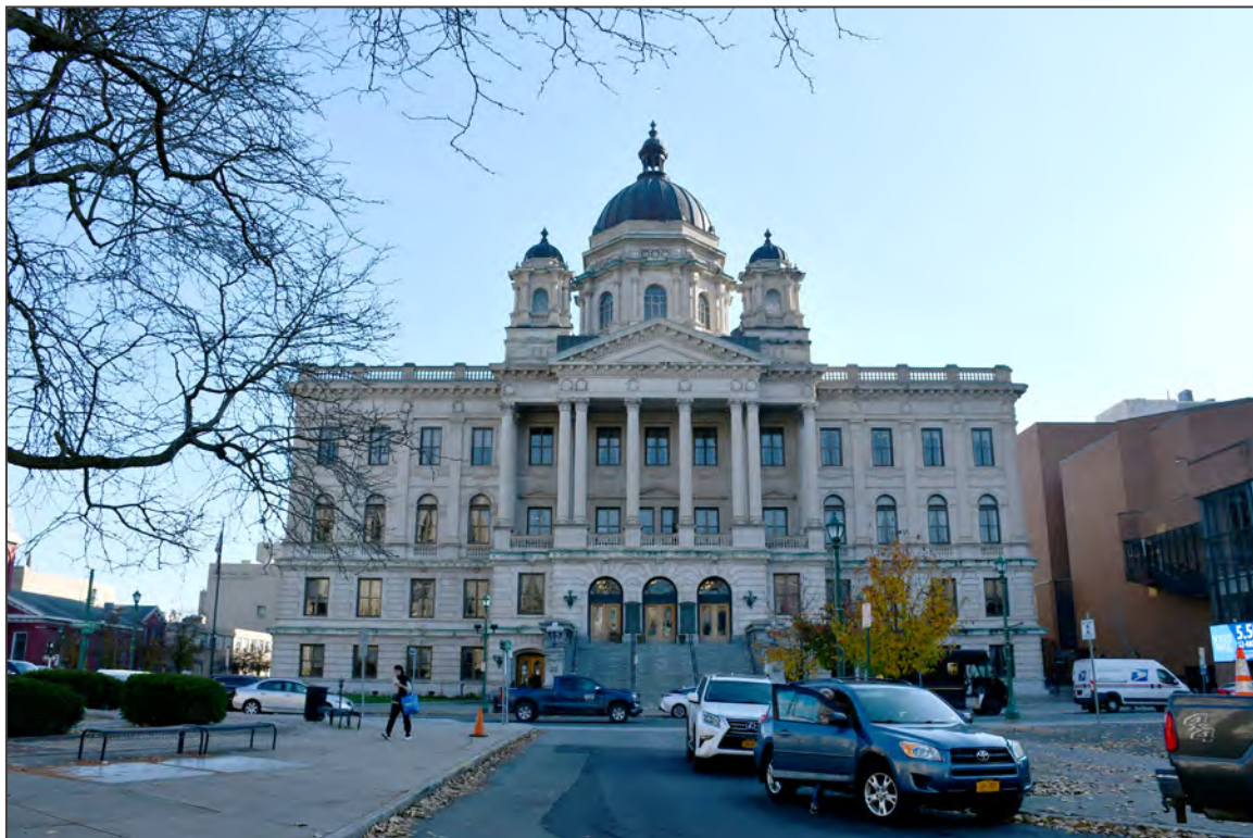
8. Fourth Onondaga County Courthouse (1904-1906), facing east
