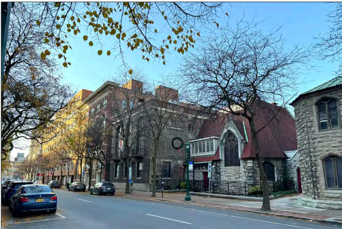
4. Montgomery Street, west side between E. Fayette and E. Jefferson streets, facing southwest
