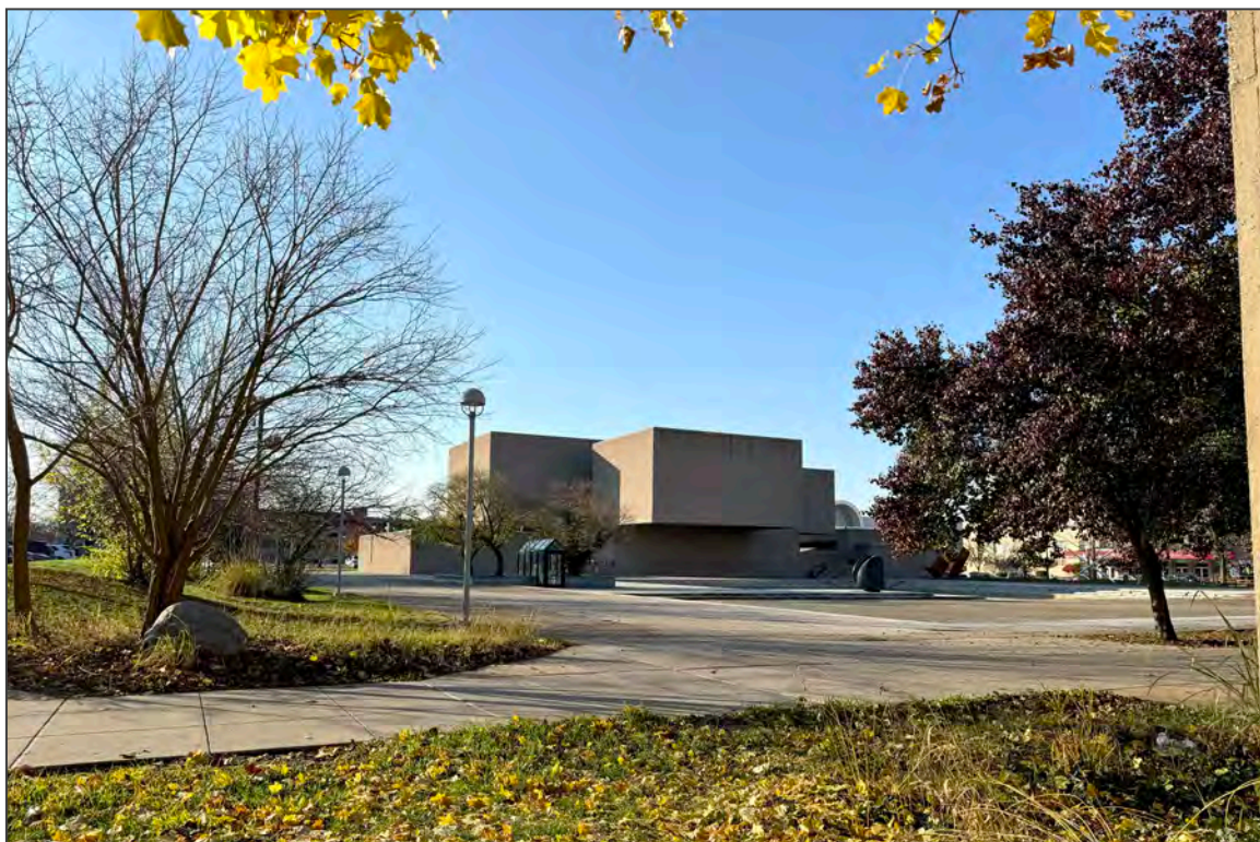
14. Community Plaza/Everson Garage (1966), Everson Museum of Art (1968), facing southwest
