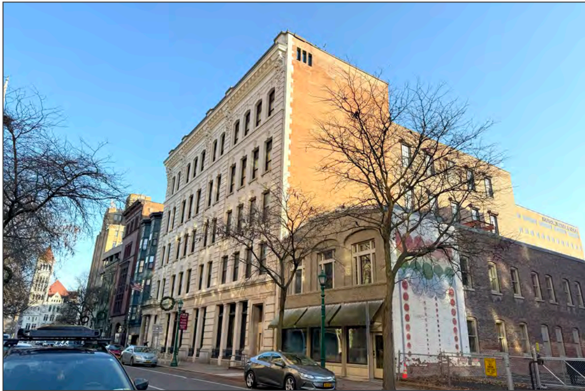
7. Montgomery Street, east side between E. Fayette and E. Jefferson streets, facing northeast
