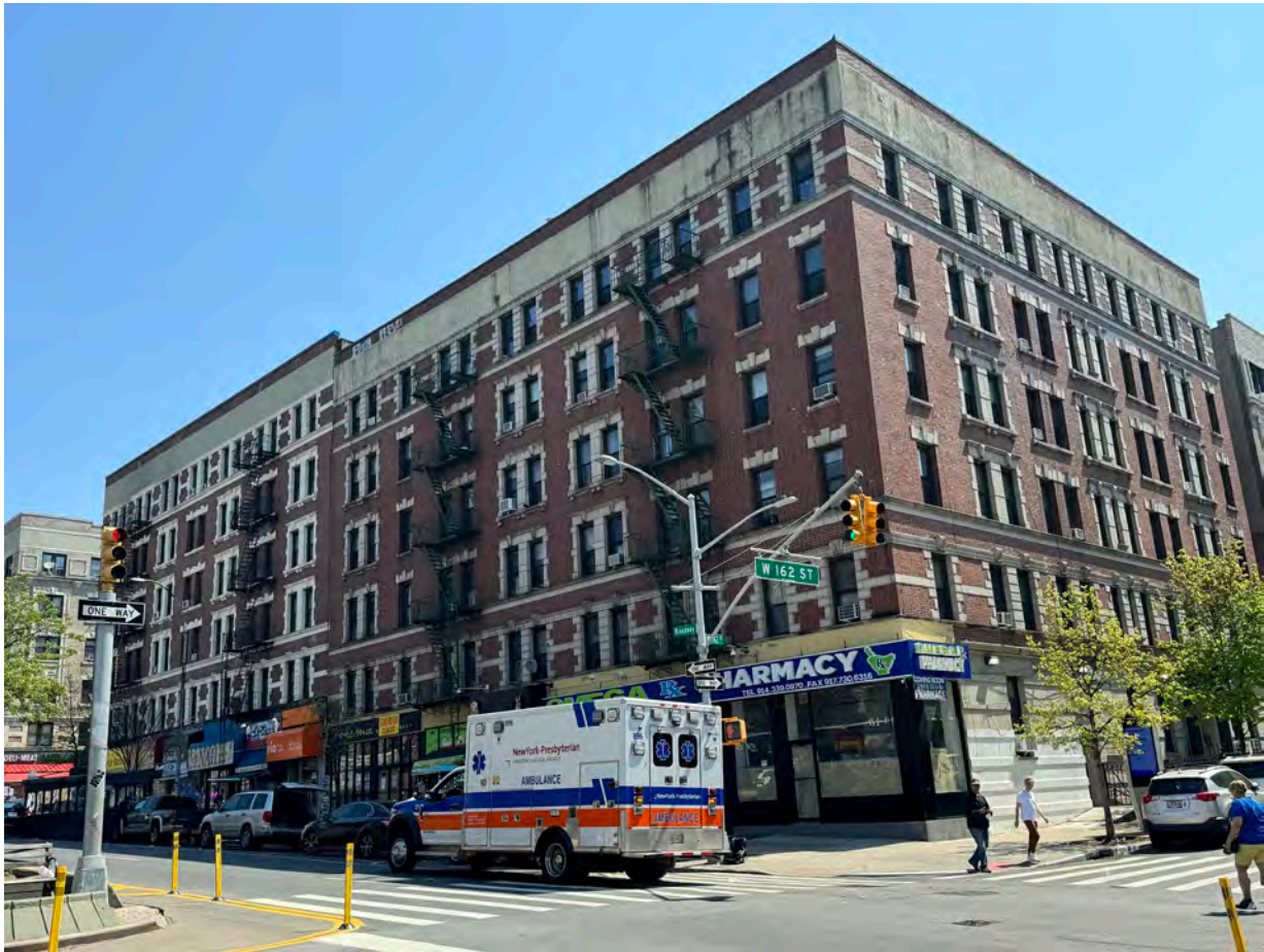
Figure 9: Piaewonsky Building, current image
