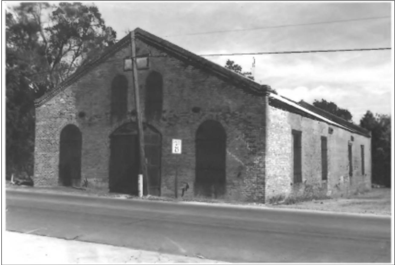
1882 Lutzenberger Foundry and Pattern Shop, 2007 Photograph, Historic American Engineering Record.
