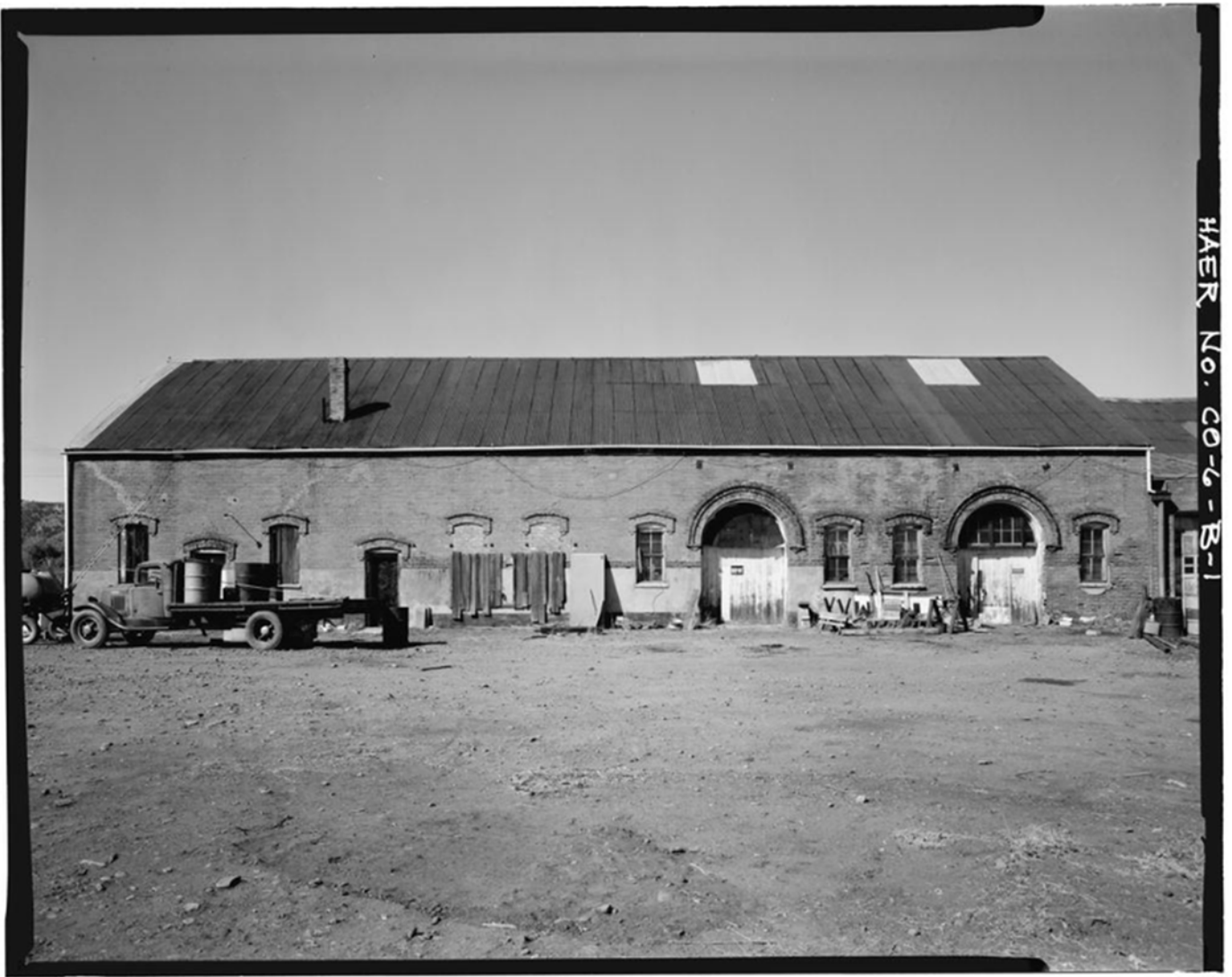
1890 Trinidad Foundry & Machine Company, 1968 Photograph, Historic American Building Record.
