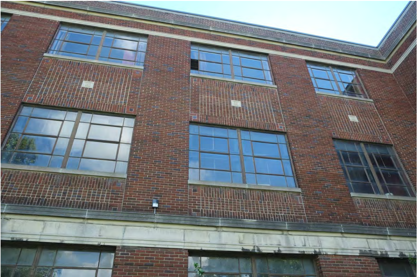
Figure 3. North elevation windows. Site visit photograph, Preservation Studios LLC, September 9, 2021.
