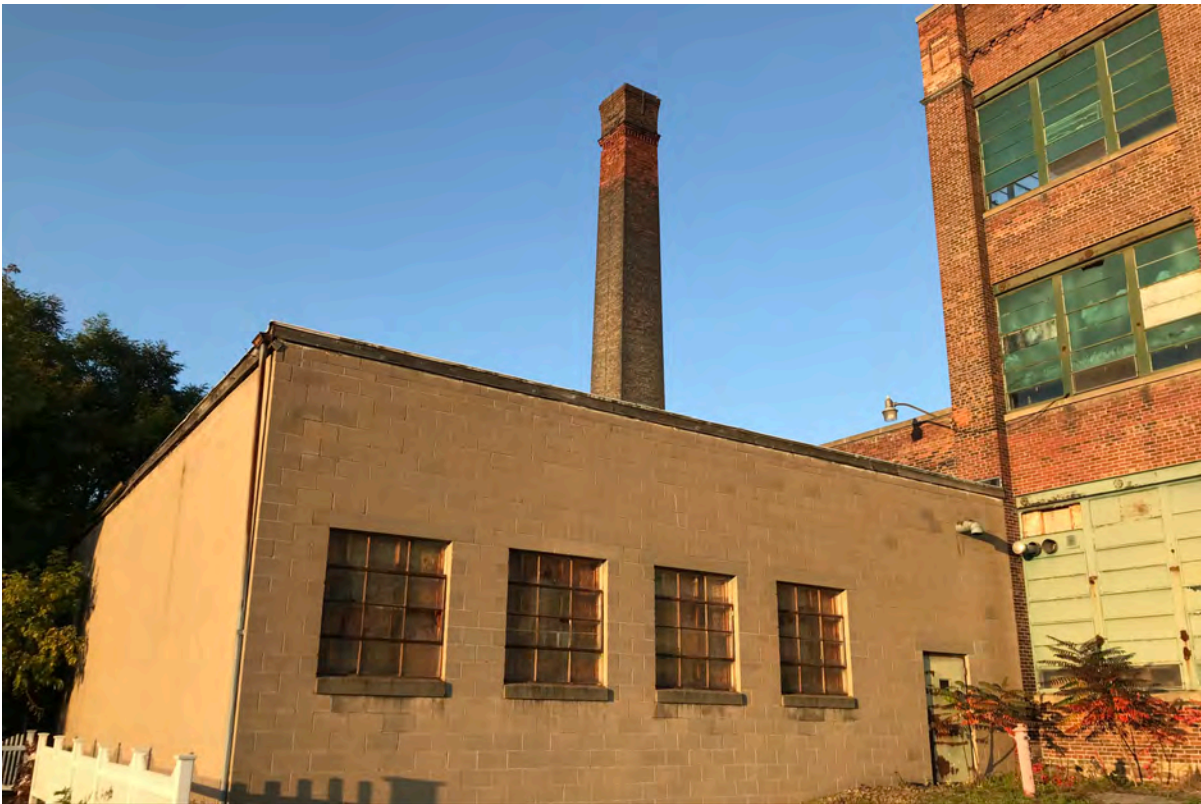
22 West wing partial west and south facades.JPG
