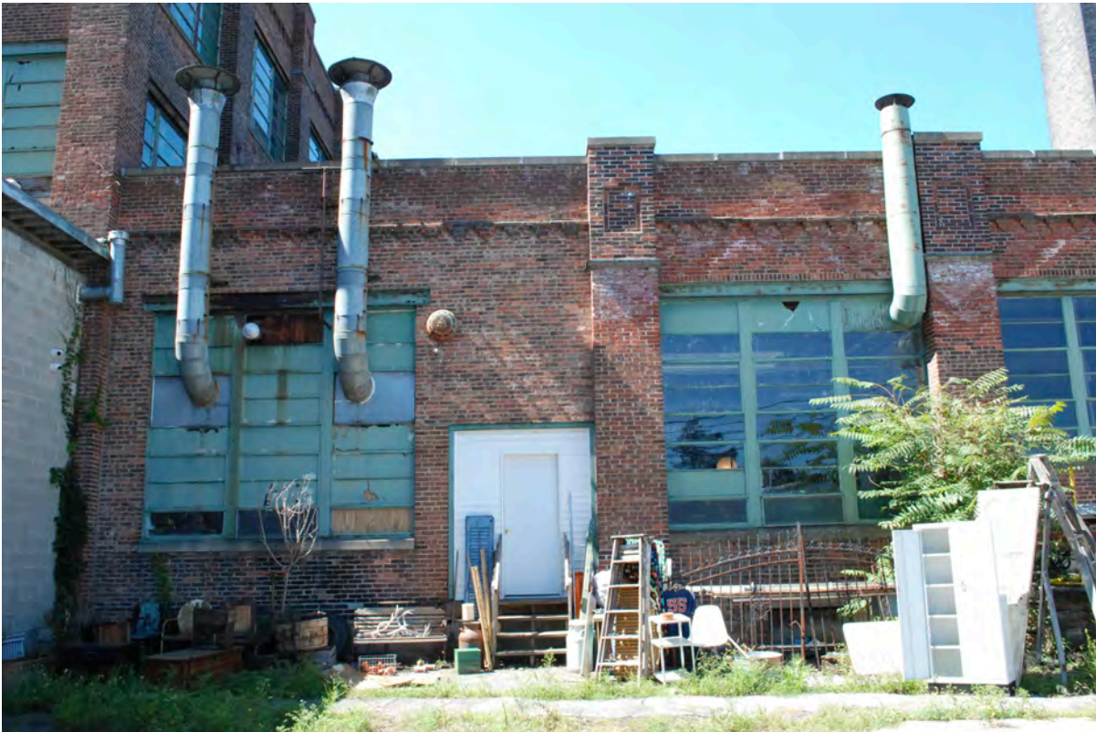
17 Additions linking factory to boiler house, looking west.JPG
