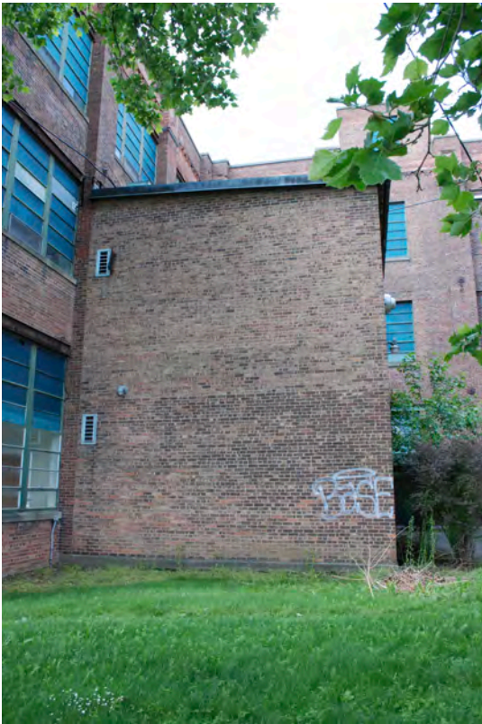
7 South courtyard vault looking north.JPG
