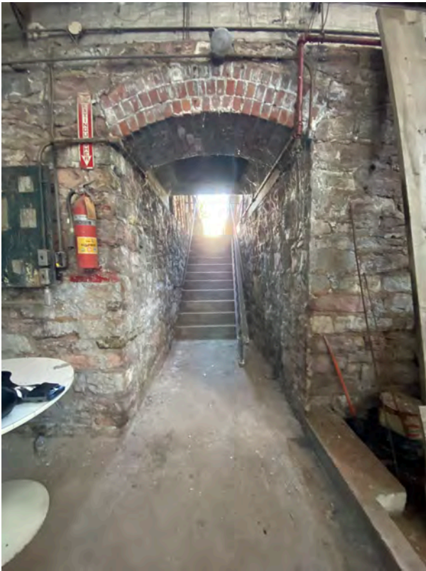
19 Boiler house exit stair basement level.JPEG
