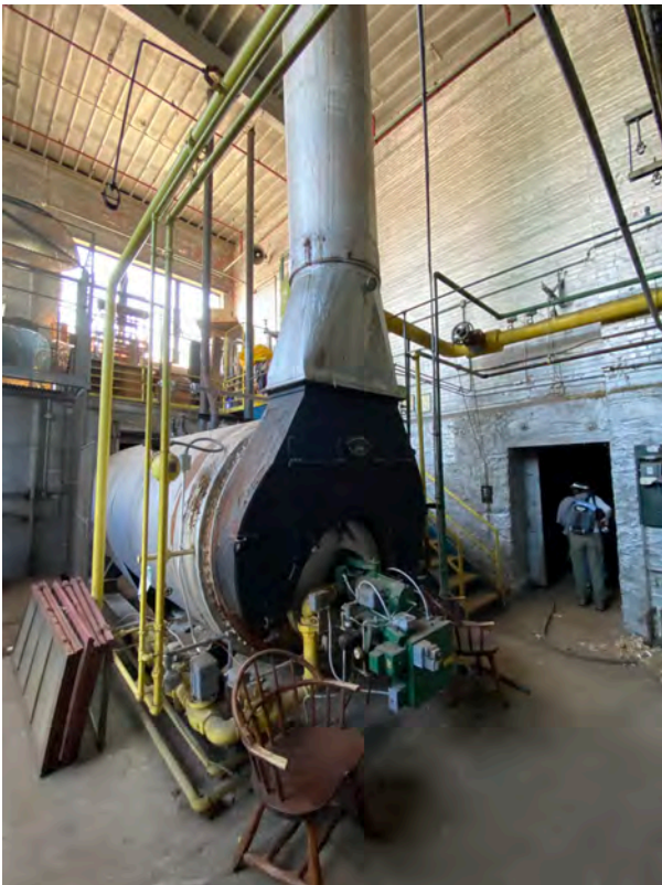
18 Boiler house interiorJPEG.JPEG
