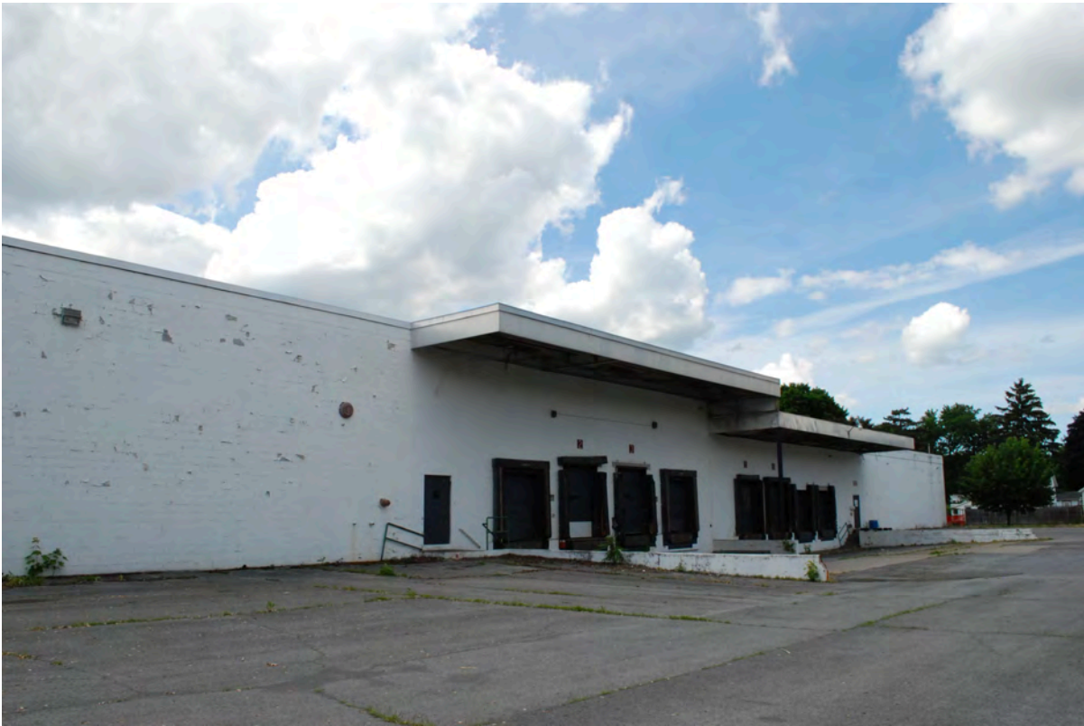
23 East warehouses east facade.JPG
