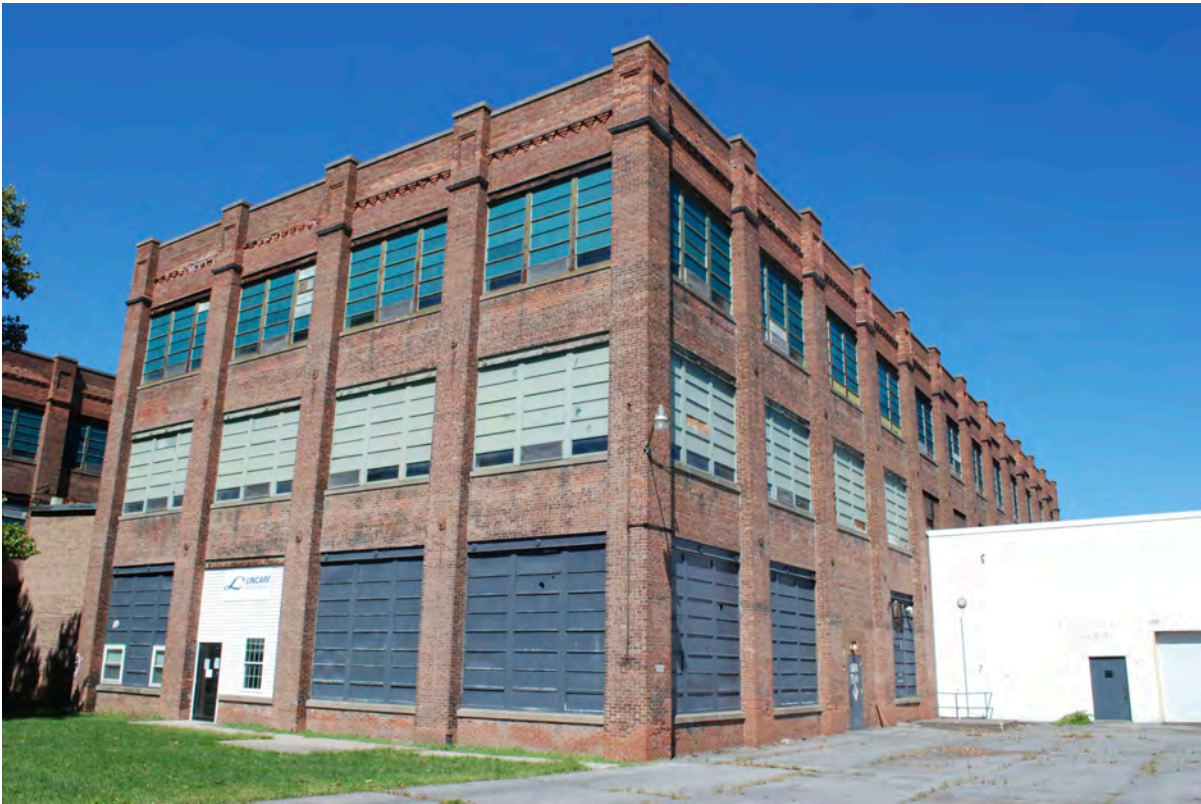
3 Factory east facade with partial 1974 warehouse addition.JPG
