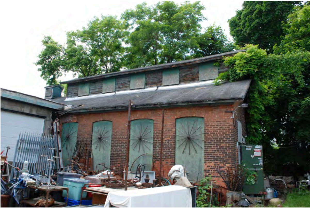
21 Tin plating plant east facade.JPG
