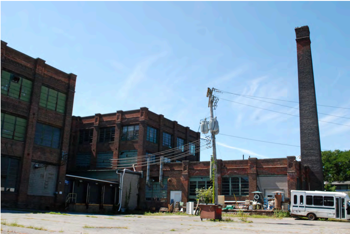
5 Boiler house looking west.JPG
