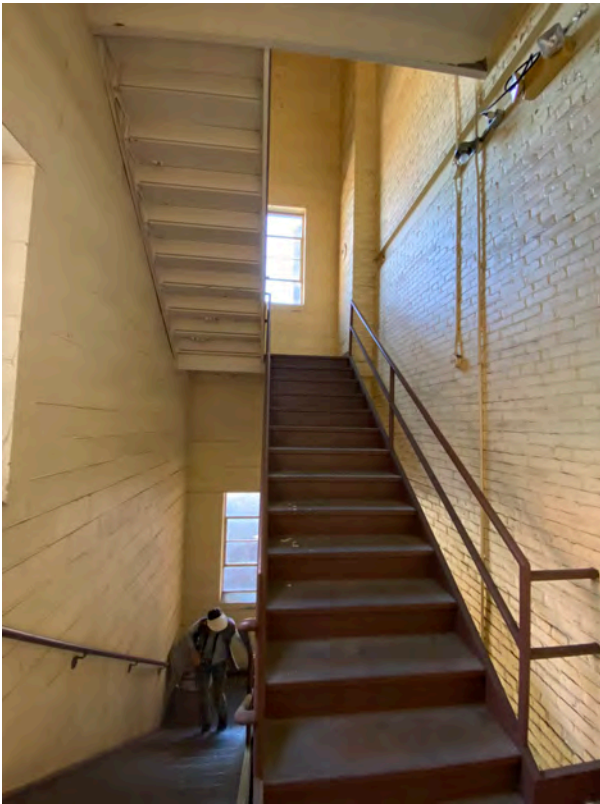
11 North stair level 1JPEG.JPEG
