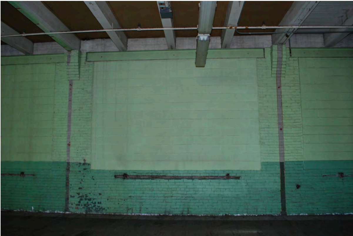
9 East window at level 2 infilled.JPG
