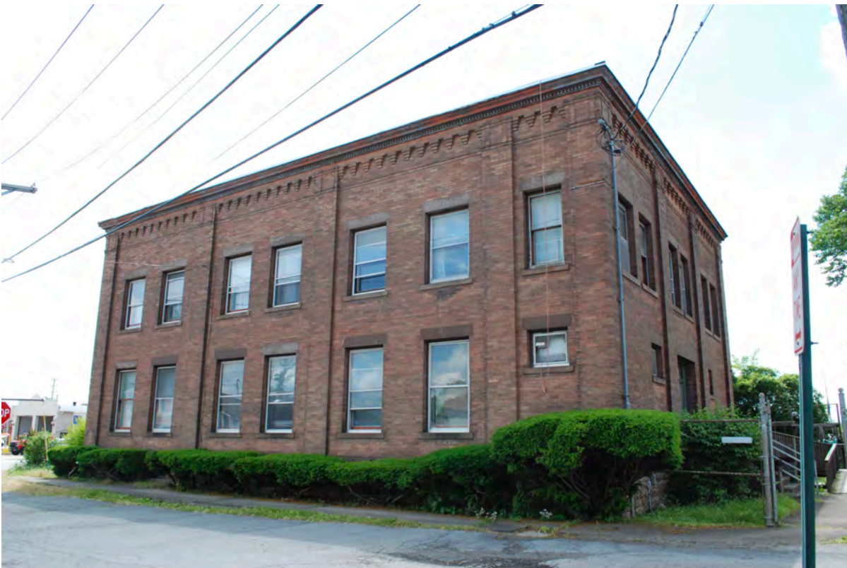
26 Office building east and partial north facades.JPG
