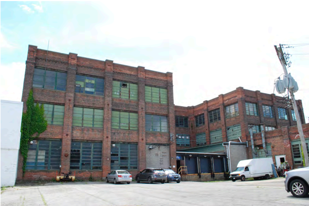
4 Factory north facade.JPG
