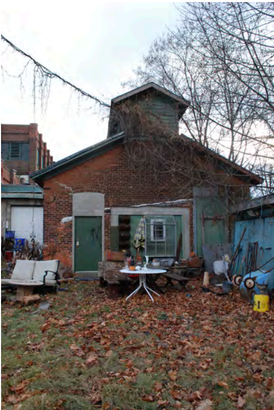
20 Tin plating shed north facade.JPG
