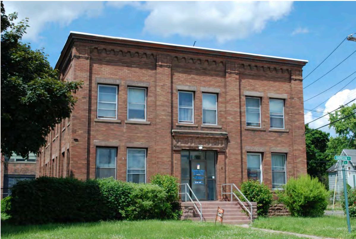
25 Office building south and partial west facades.JPG
