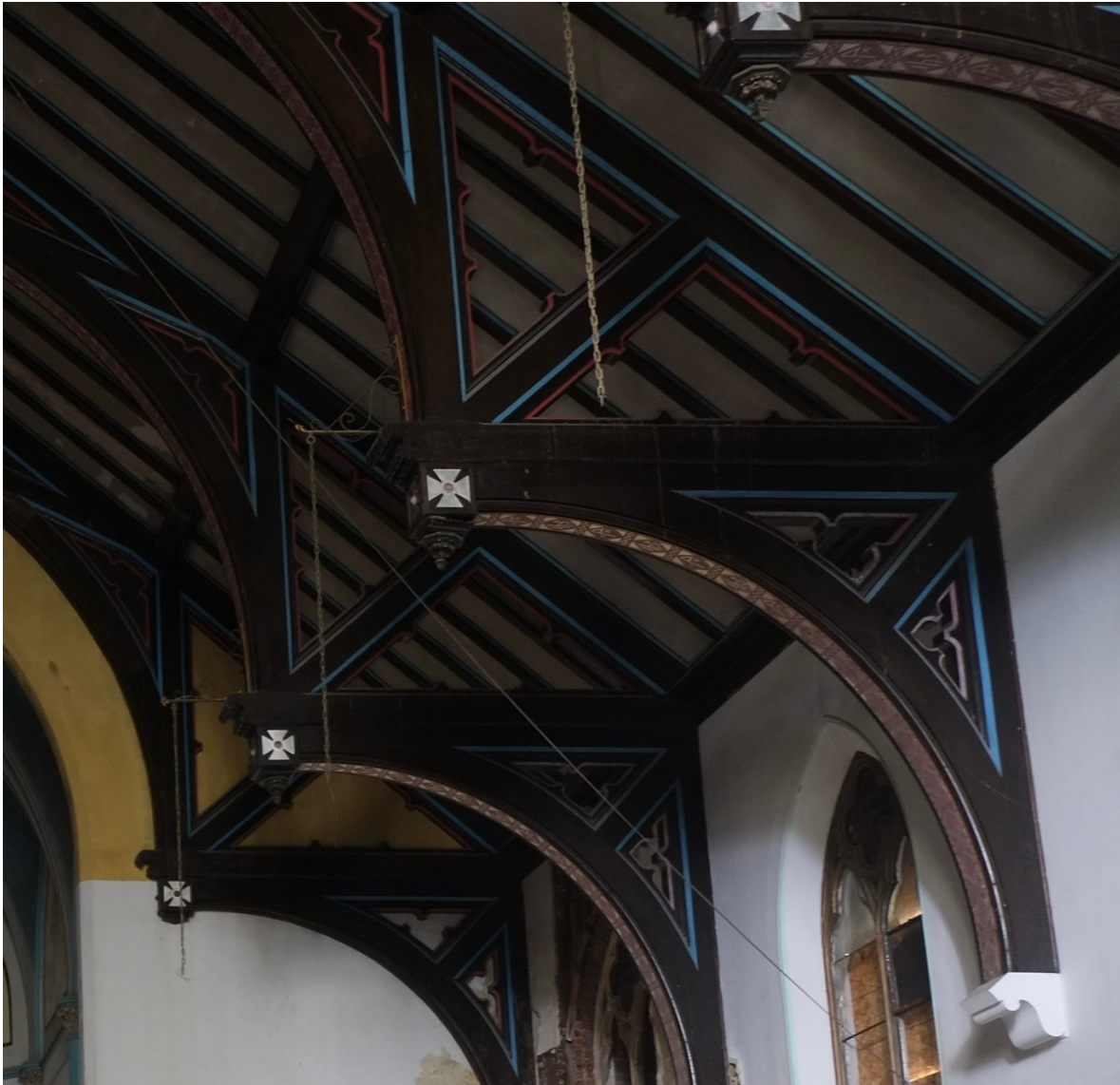
Figure 9: Detail of carving and painting on truss work
