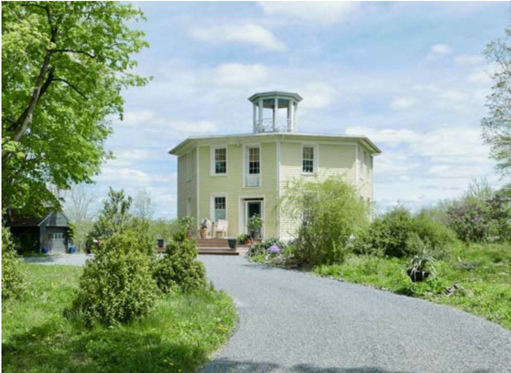
PHOTO 0001: View of house from west.
