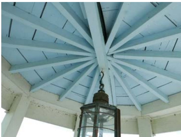
PHOTO 0020: View of interior of belvedere roof.
