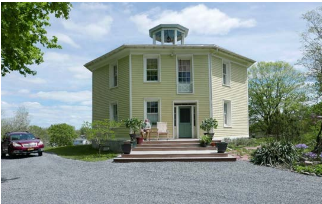
PHOTO 0002: View of facade from west.
