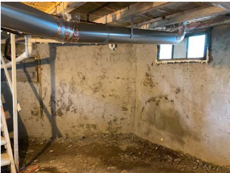
PHOTO 0022: View of grout wall in basement.
