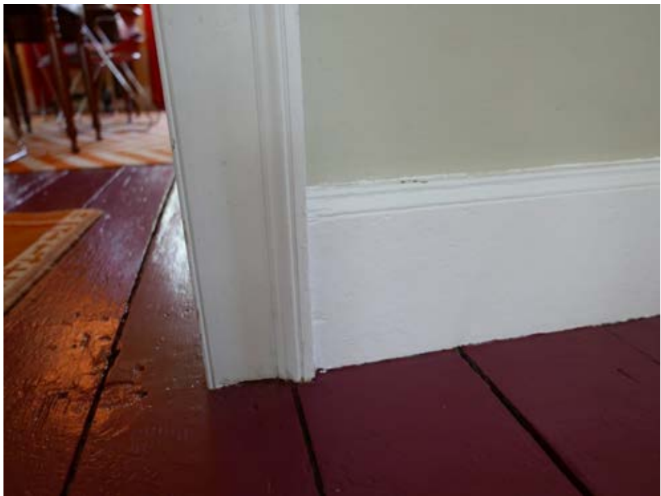
PHOTO 0010: Detail of floor and woodwork in first-floor living room.
