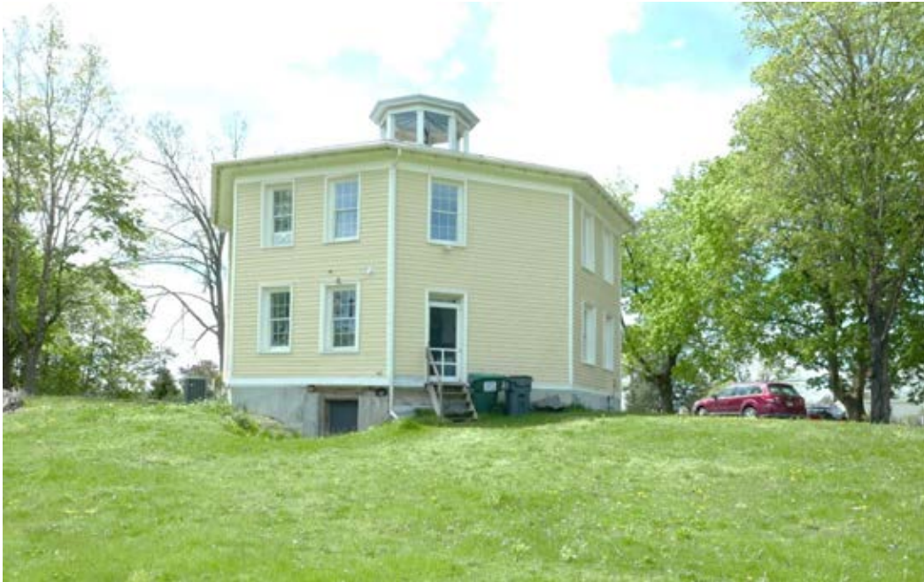
PHOTO 0005: View of exterior from east.
