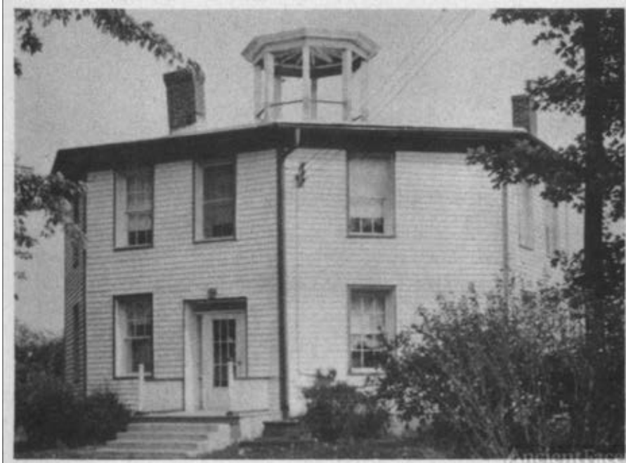
Fig.5: Photograph of house in 1957 with porches removed.
