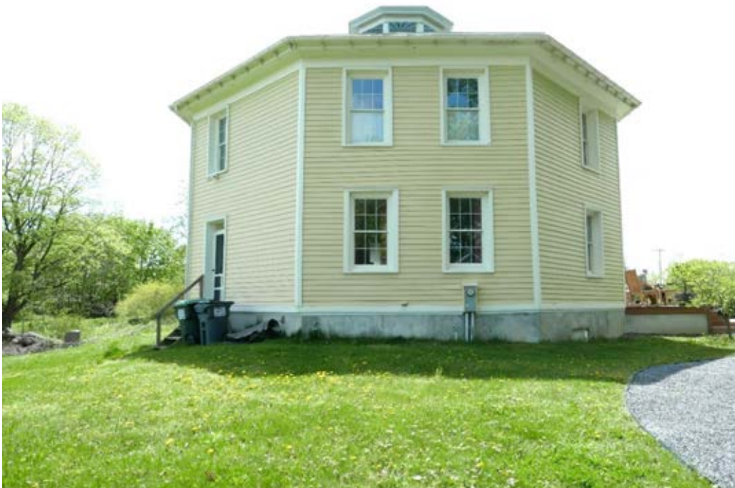
PHOTO 0006: View of exterior from north.
