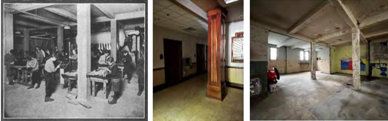
Figure 2-4: 1920s Photo of First Floor Workroom (left), 2022 Photo of Lobby (middle), 2023 Photo of Lobby with Selective Demolition of Contemporary Finishes (right).
