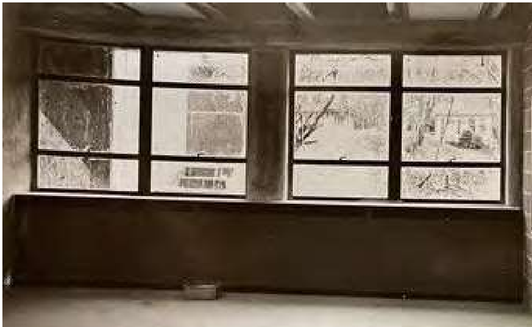
Figures 8 & 9: Construction Photos
