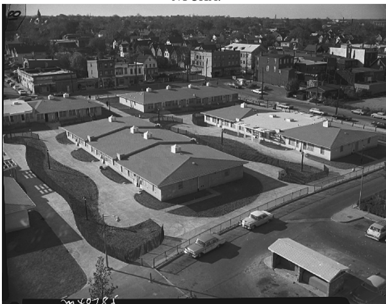
Figure 13. 1965 photograph of West Brighton II showing original curved walkways. Courtesy of the LaGuardia & Wagner Archives.
