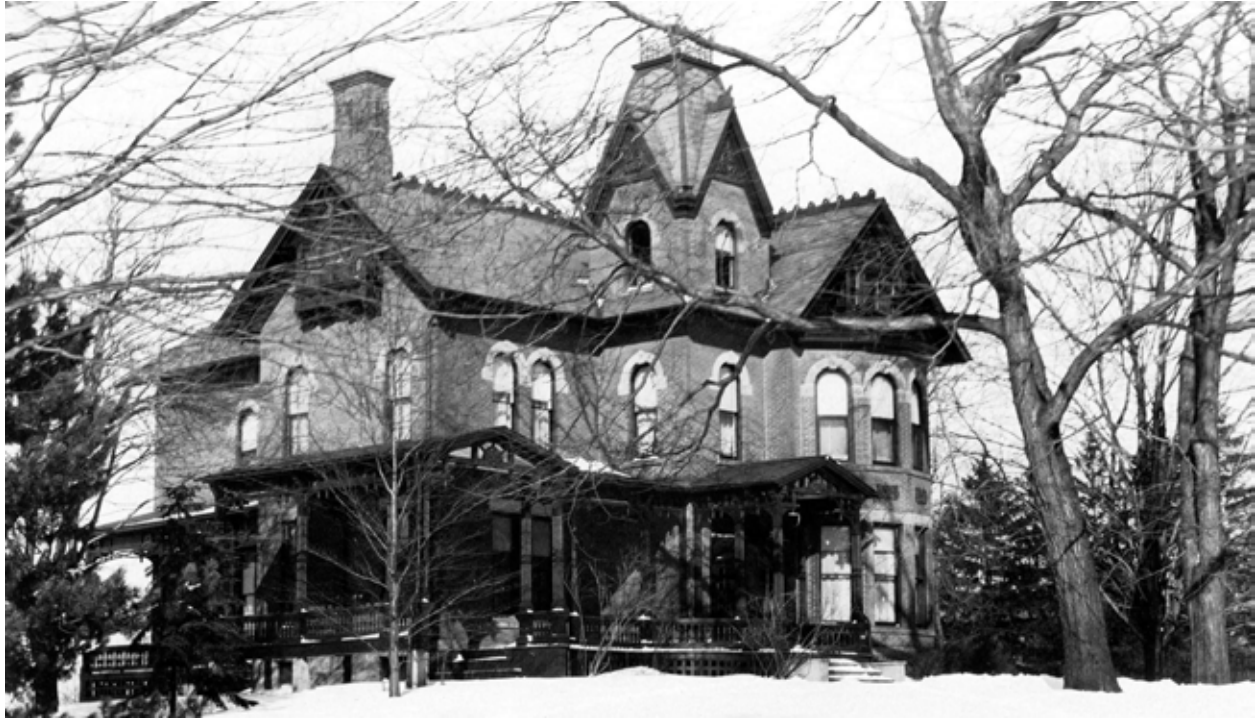
Figure 11: 1923 Photo of the Yeomans House Southwest View. Note the crested tile, porticos, and porte-cochere, missing today.
