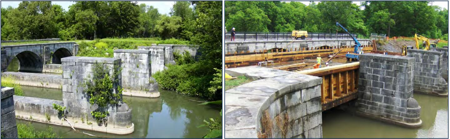
*The aqueduct before (above left) and during its restoration (above right), showing the laminated timber trough being constructed within the limestone structure.*
