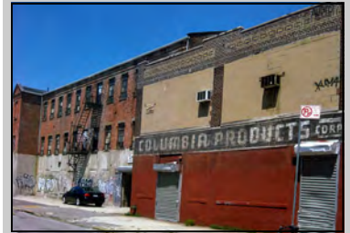
Rehabilitation of 221 McKibben Street in Brooklyn created affordable industrial spaces for small firms and preserved both the physical industrial heritage of the community and local opportunities for industrial jobs.
